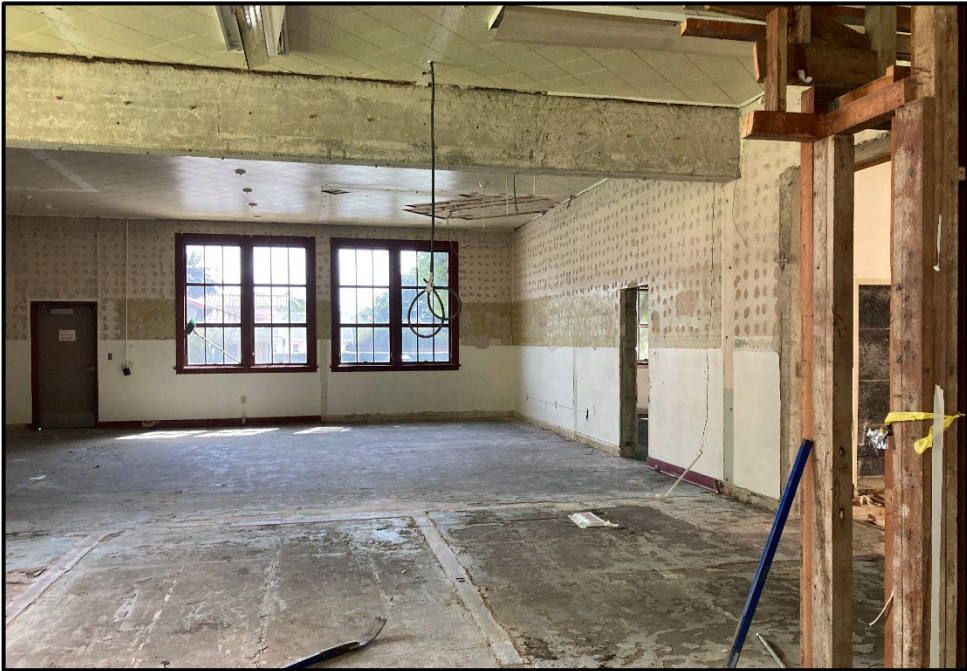
SMHS Admin to Classroom – Demolition of the Interior Continues
