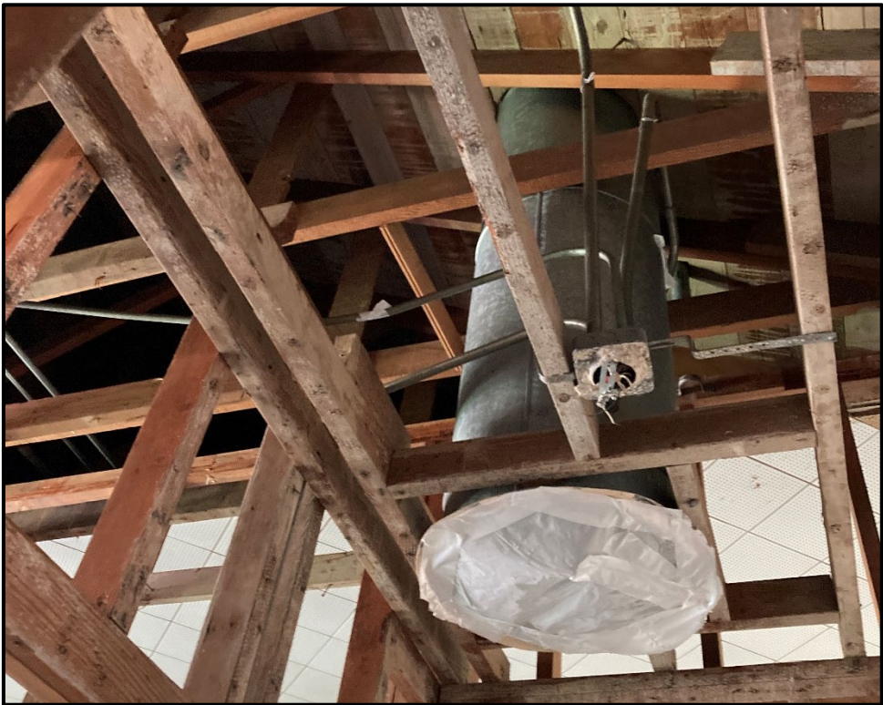
SMHS Admin to Classroom – Exposing Vents for HVAC Installation
