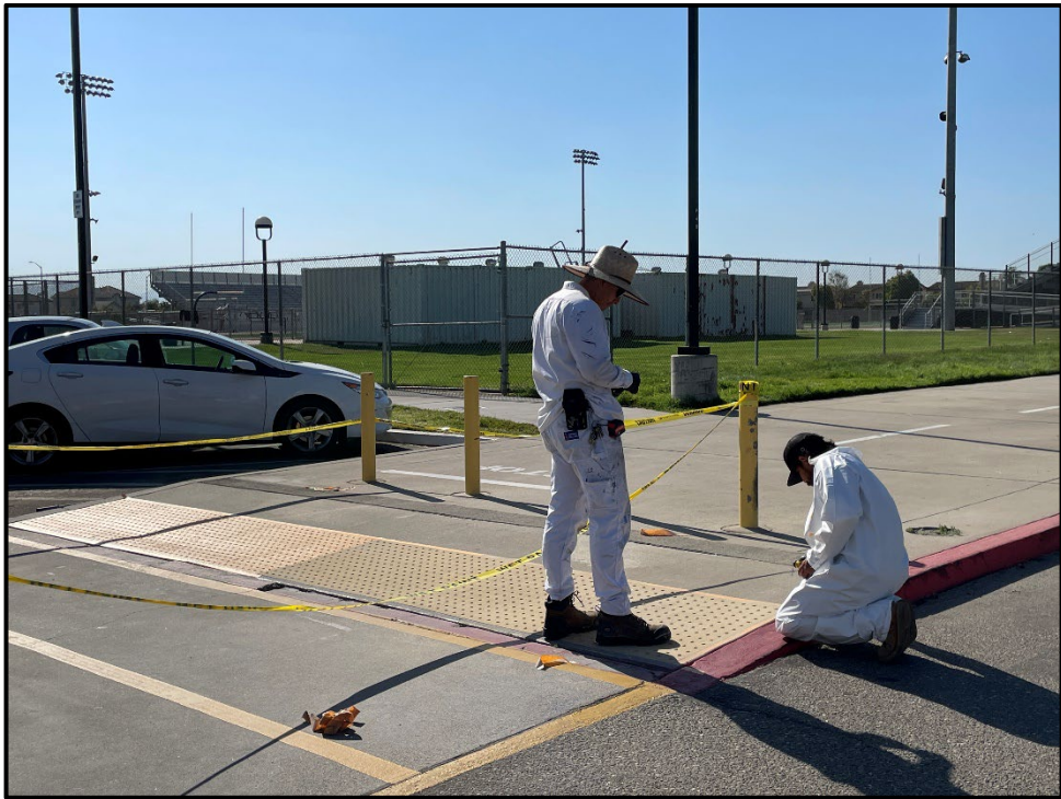
PVHS – Joel Amezcua and Tom Harbold Installing the ADA Truncated Domes
