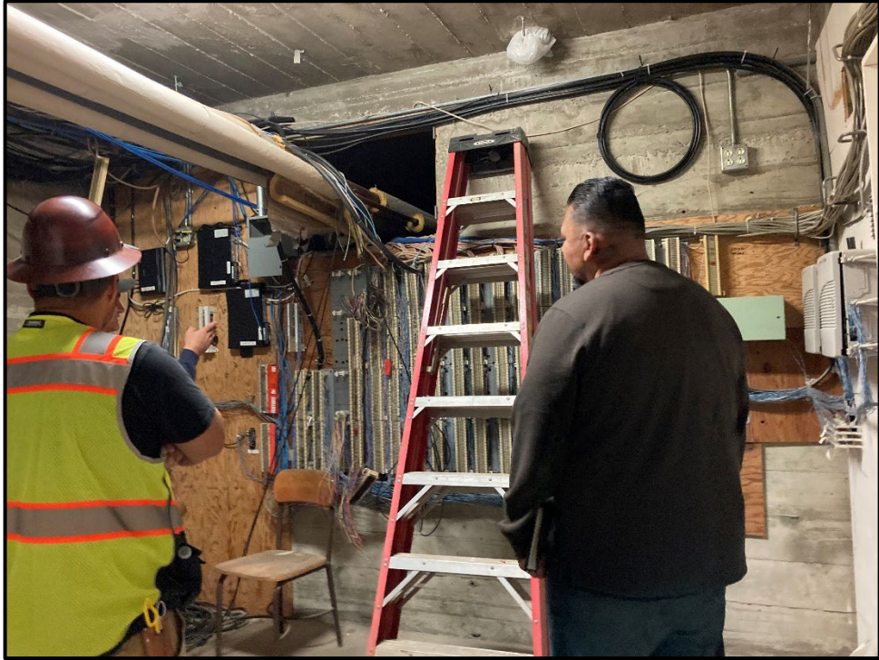
SMHS Admin to Classroom – Subcontractors Reviewing Electrical and Data Layout
