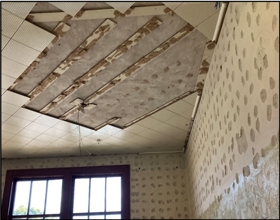
SMHS Admin to Classroom – Removing Ceiling Tiles to Expose Wiring
