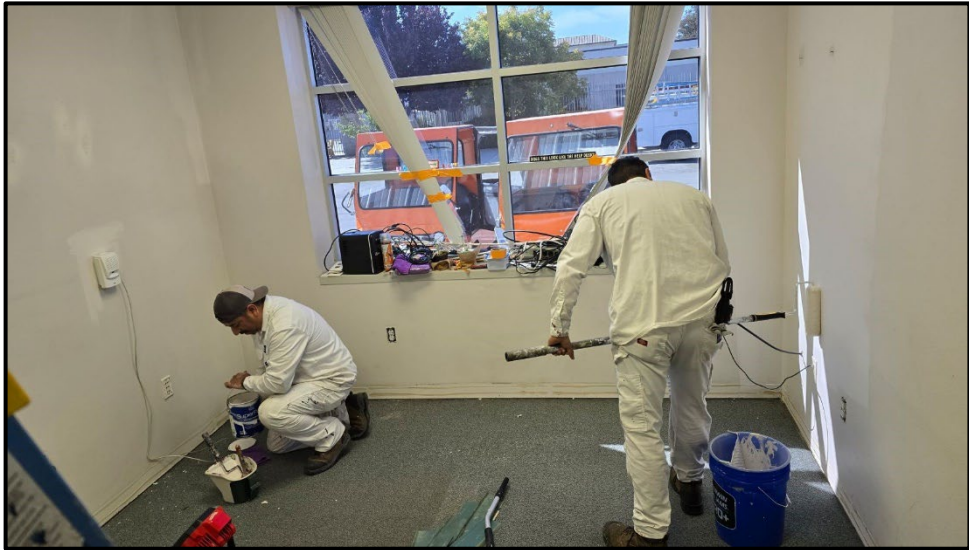
PVHS – Ernest Paz and Joel Amezcua Painting the M+O Offices
