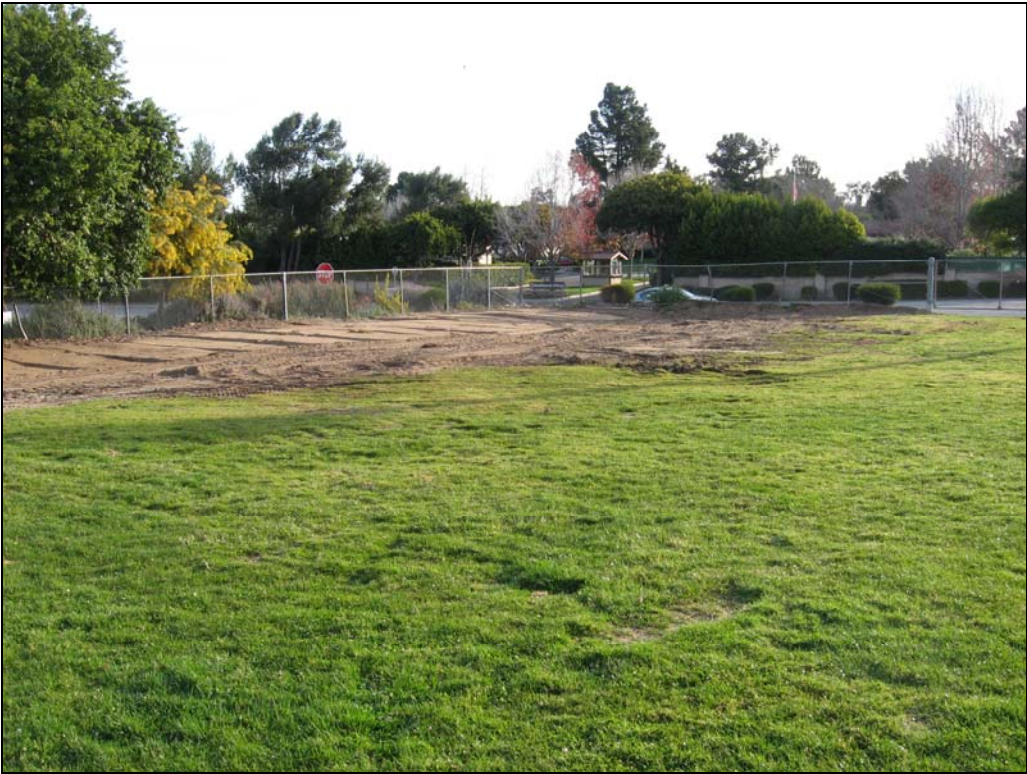
ERHS Baseball Fence Line Cleared to Improve Curb Appeal
