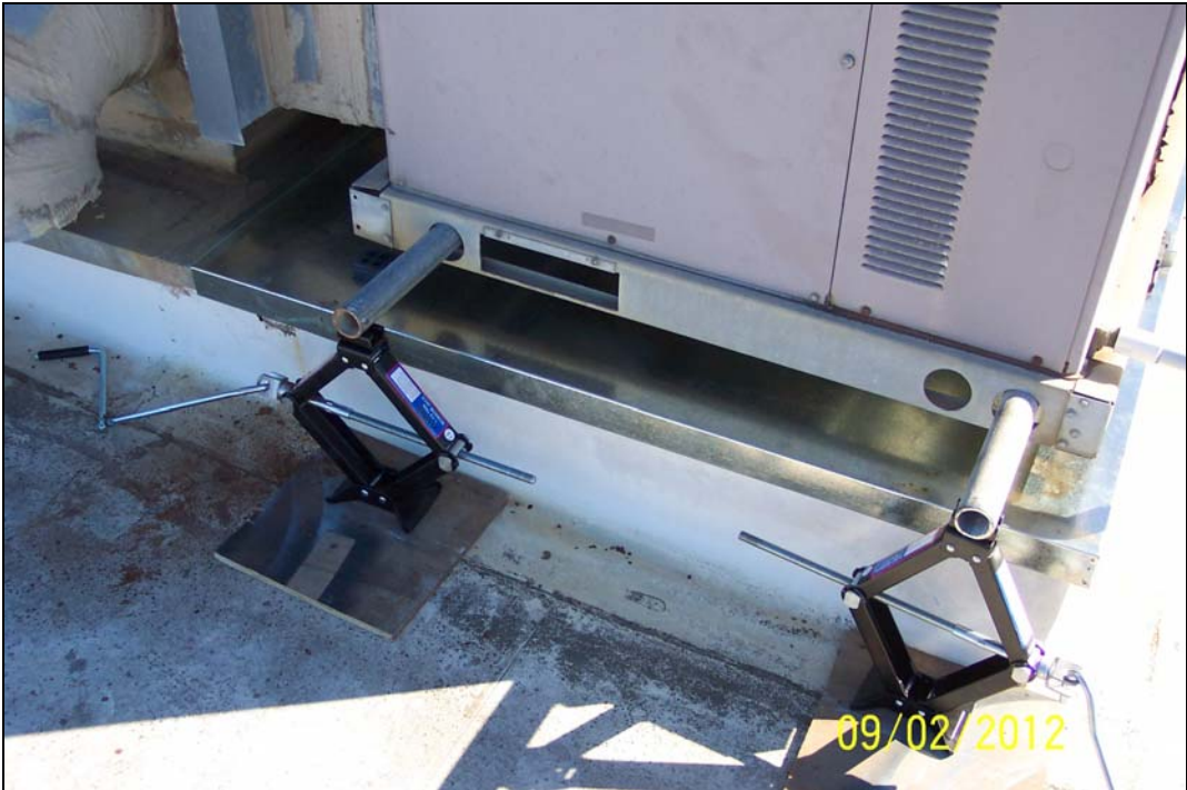
New Sheet Metal Pans for 440s Classroom Heating Units
