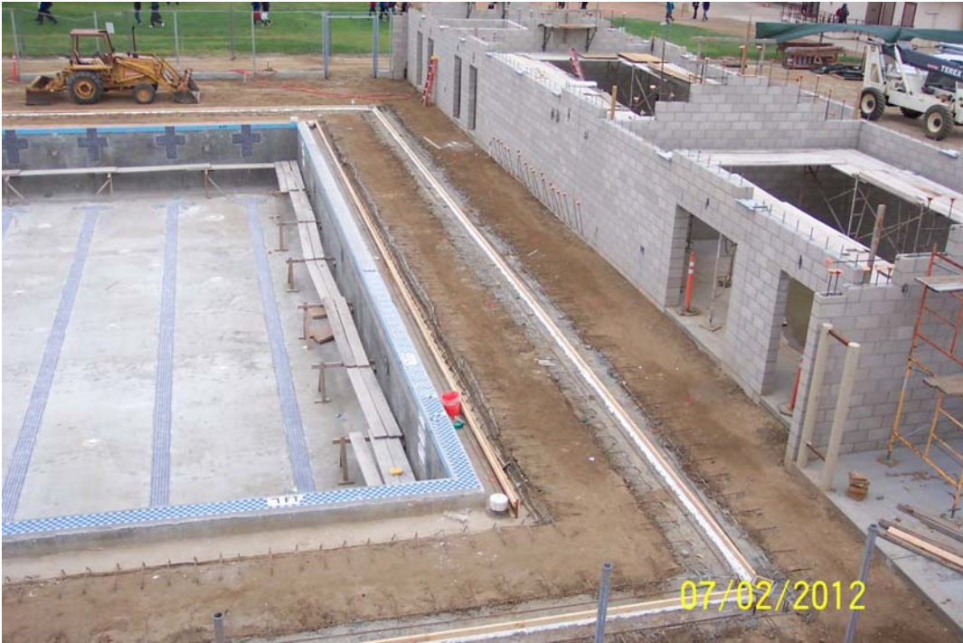
SMHS Pool Deck at Equipment Building – Before Concrete...
