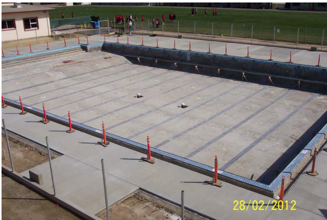
SMHS Pool Deck Begins to Receive Concrete
