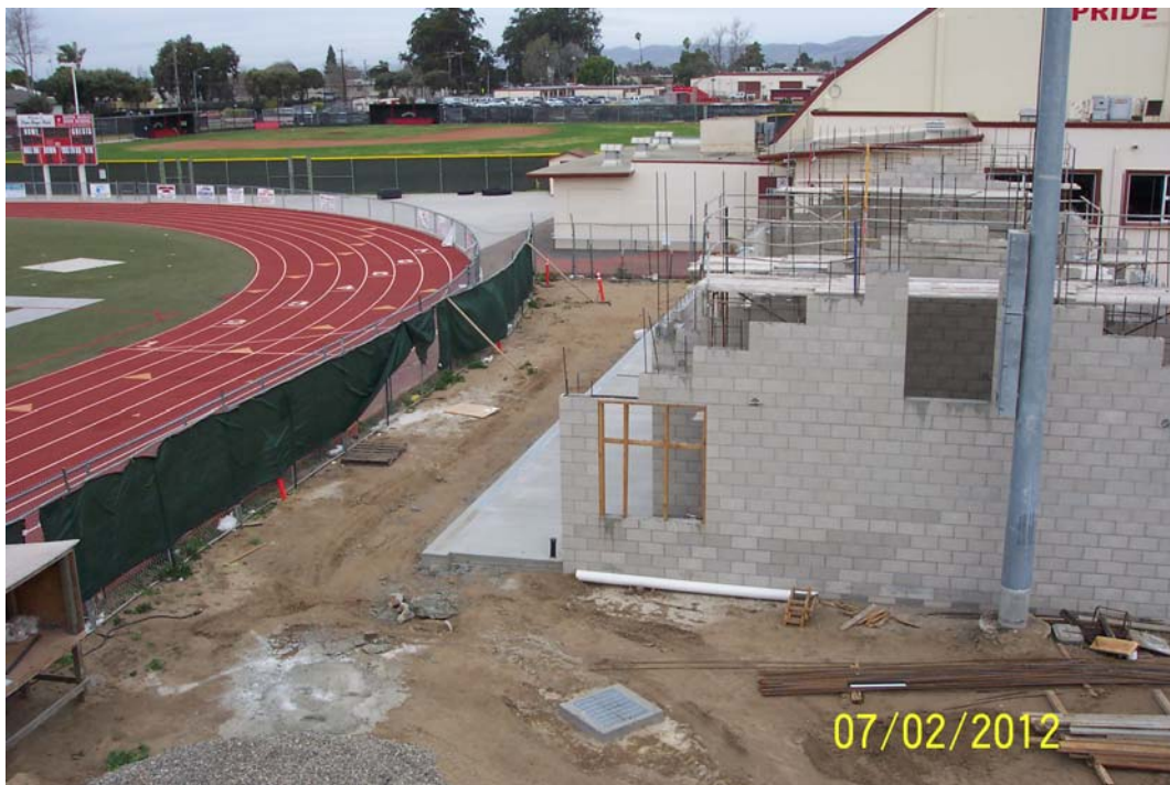
SMHS Pool Concession Ready For Concrete
