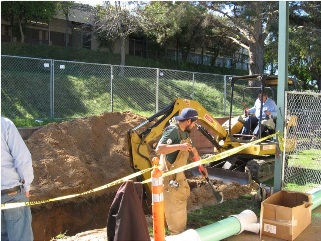
Digging to Replace Sewer Line Near RHS Gymnasium
