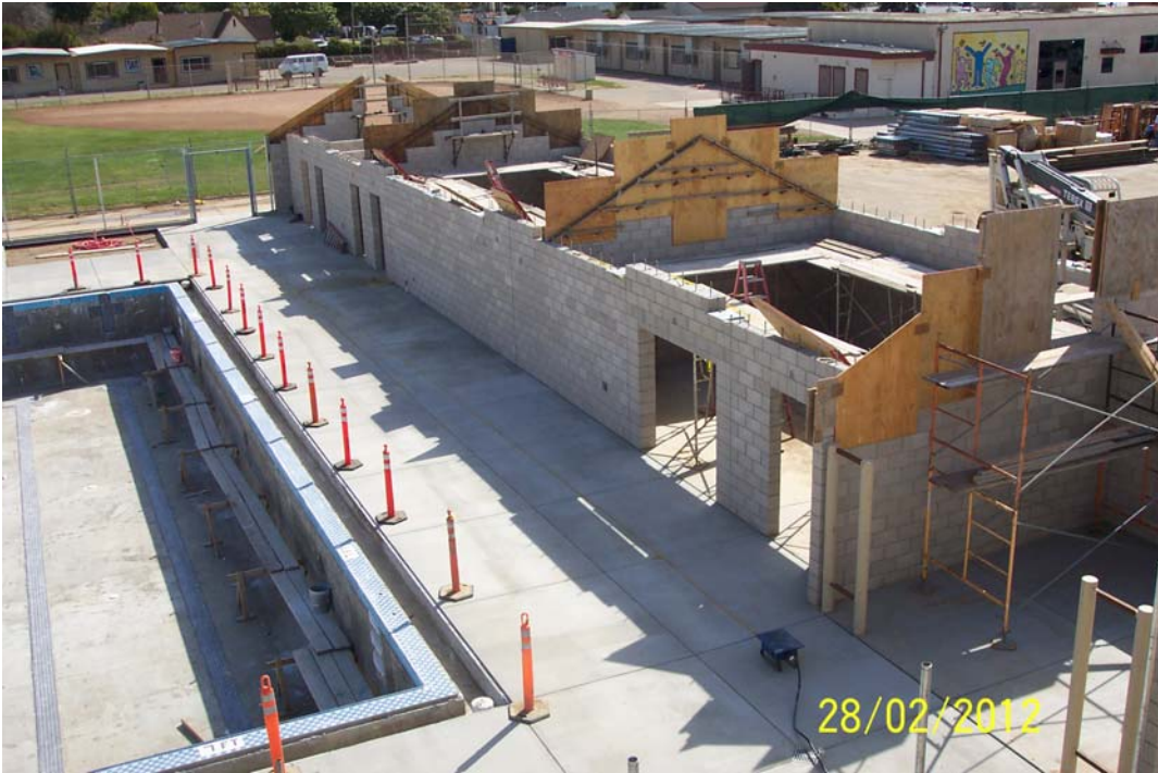
...And After concrete Poured
