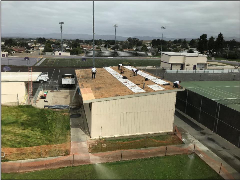
ERHS Weight Room – The Old Roof is Removed and Decking is Patched
