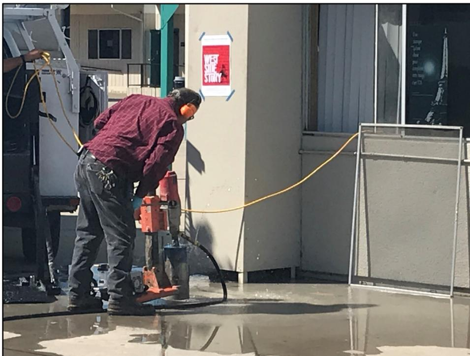
PVHS - José Placencia Drills Holes for Bollards to Protect Fire Sprinkler Risers
