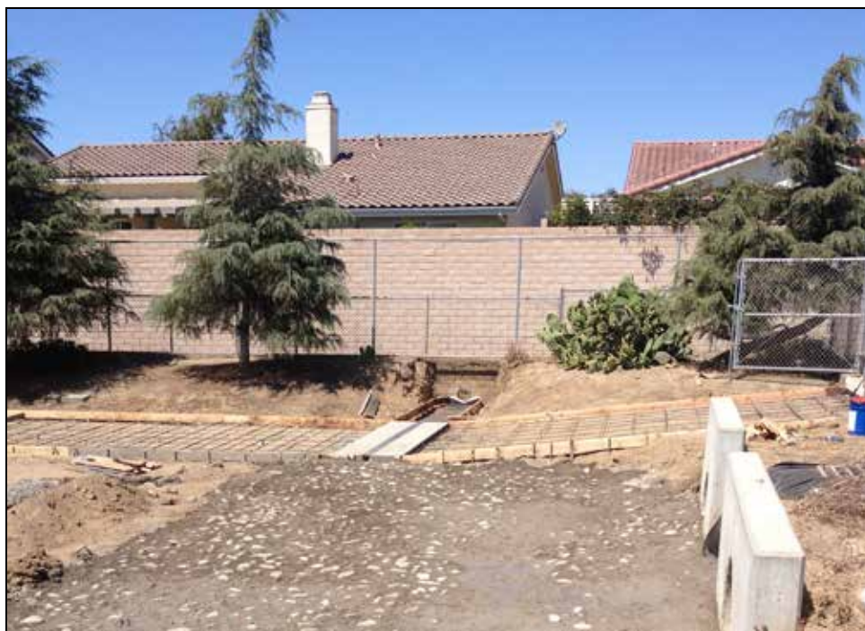
PVHS - Concrete Ramp to the Detention Basin Formed and Ready to Pour
