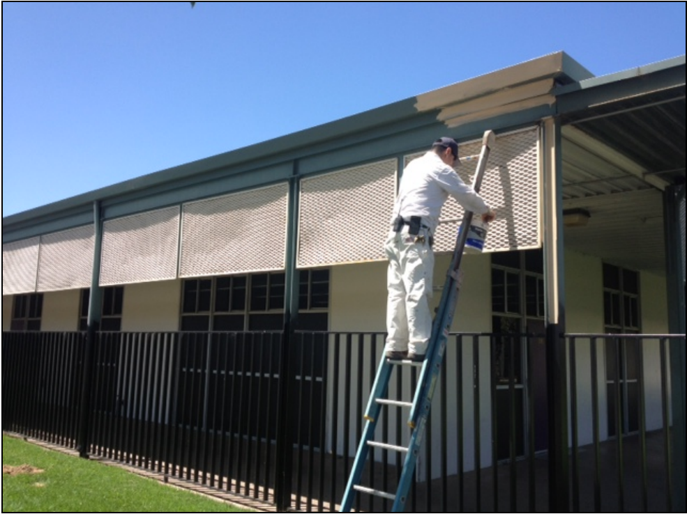
ERHS - Ernest Paz Painting the Trim in the Front of the School
