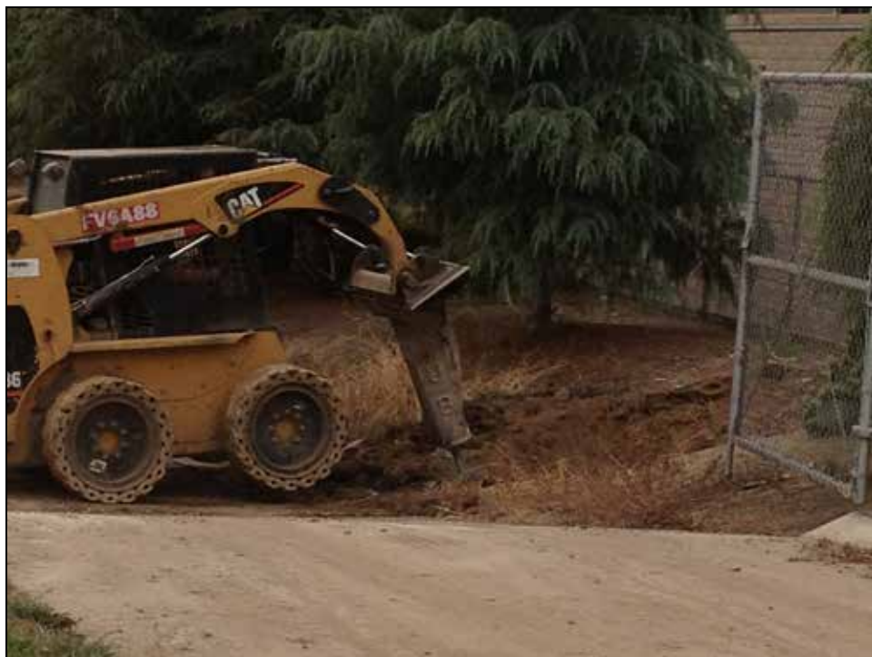
PVHS - Final Concrete Remediation Item - Ramp to the Detention Basin
