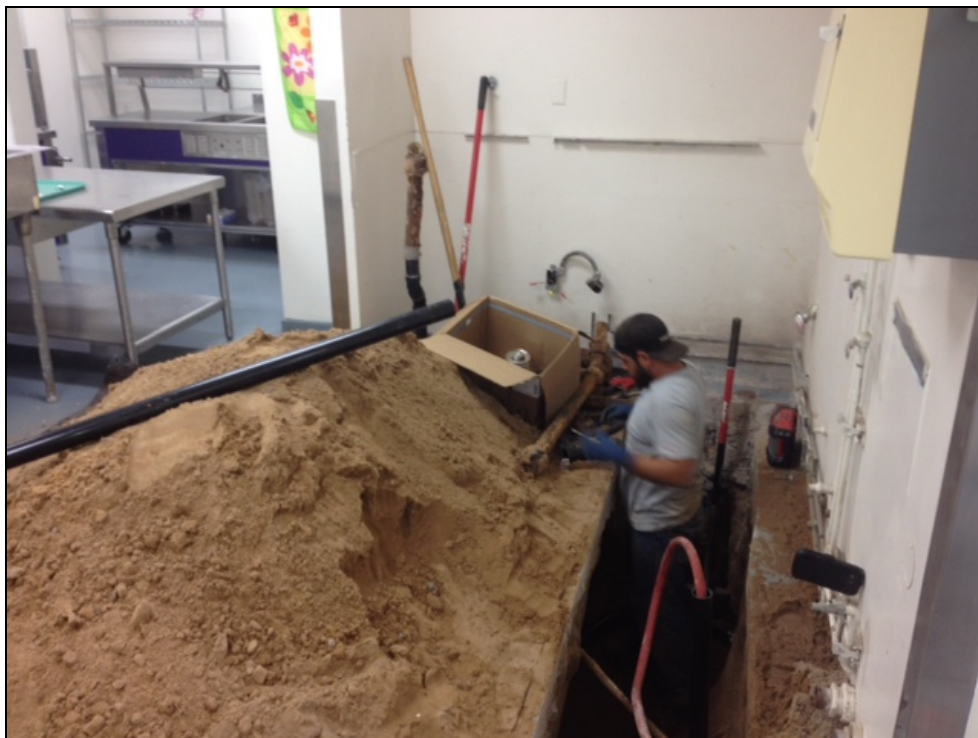
ERHS – Flavio Rodriguez Repairing a Collapsed Drain in the Cafeteria
