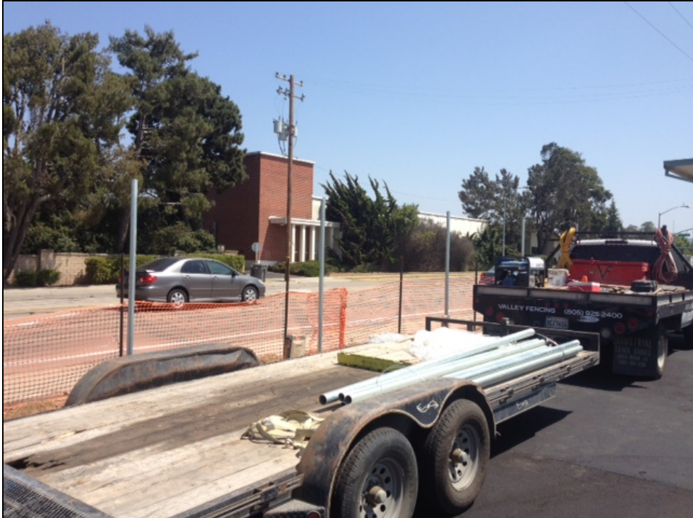
ERHS - New Bradley Road Fencing Improves Curb Appeal
