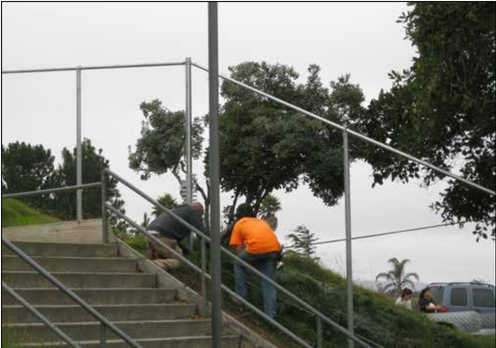
EHRS - Fencing Between the Science Building and Student Parking Lot
