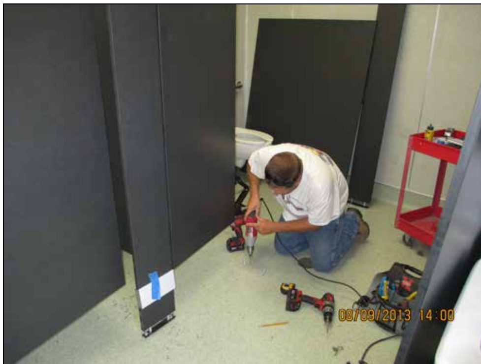
SMHS - Erik Fulton Replaces Restroom Partitions at the Learning Center
