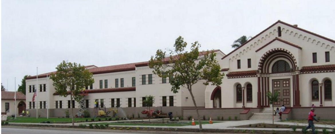
The new two-story classroom building on Broadway (left) and adjacent Ethel Pope Auditorium (right)
