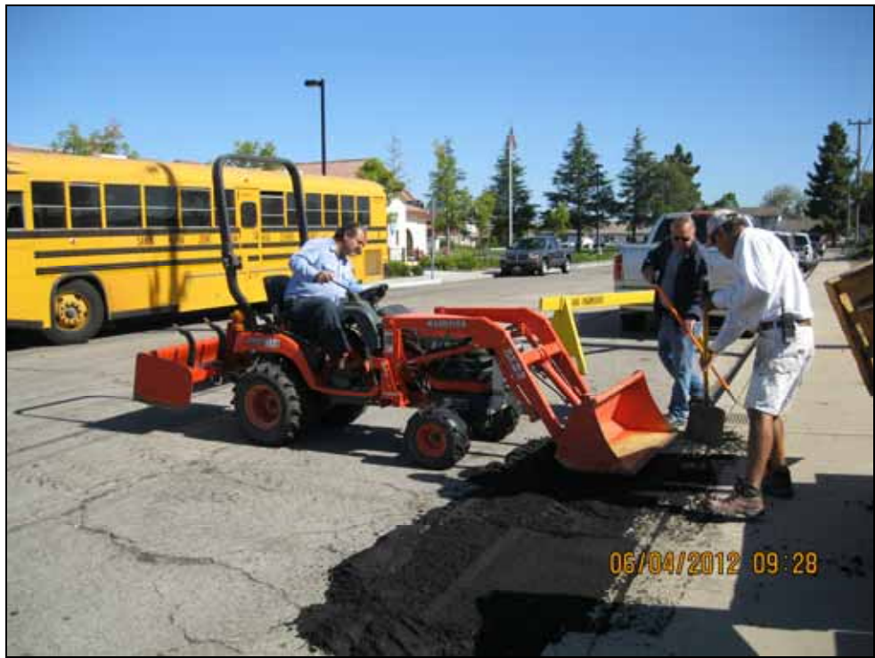
District Maintenance Creates a Parking Lot for DHS Graduation
