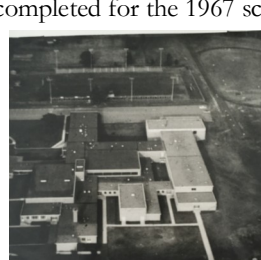
The dark roof is the original part of the school and the light roof is the addition.
