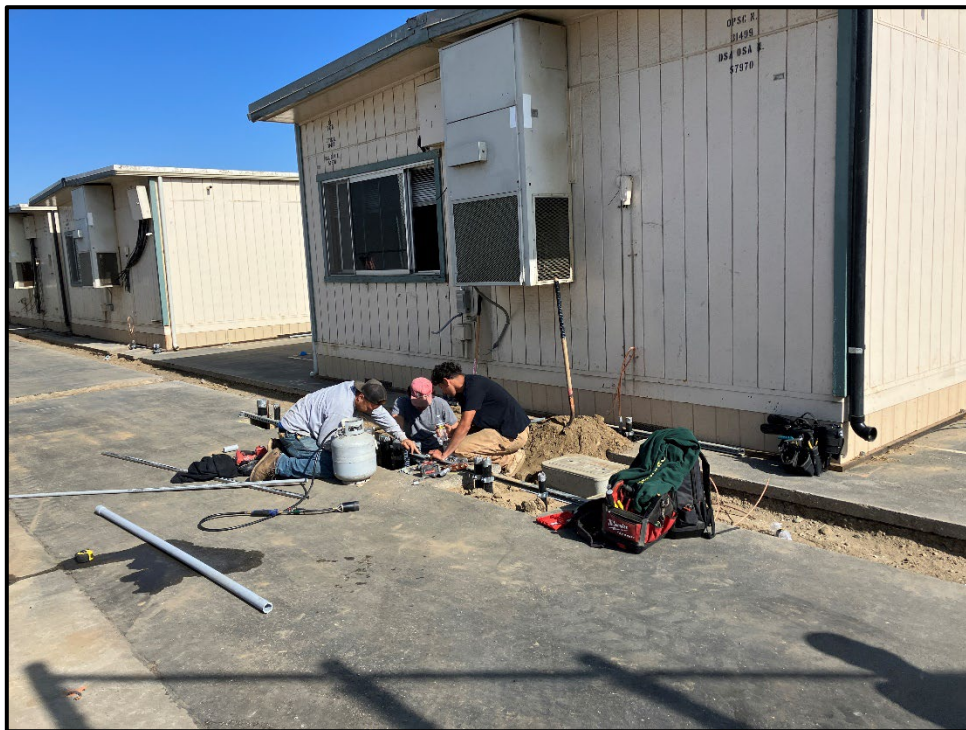
PVHS 10 Portable Classrooms – Electrical and Communication Conduit Installation
