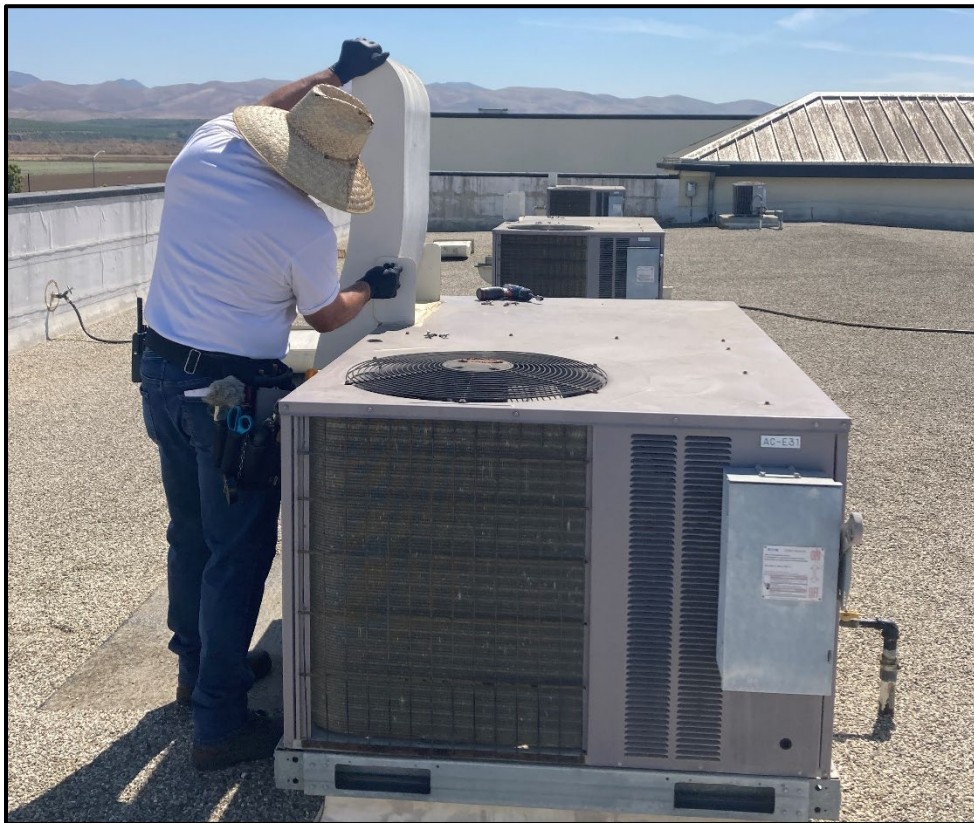
PVHS – Elias Camacho Services a Roof-top Air Conditioning Unit
