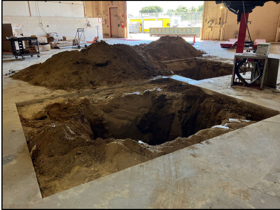
SMHS CTE Modernization – Auto Shop In-ground Hoists are Removed
