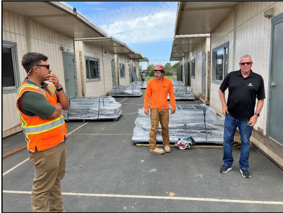
PVHS 10 Portable Classrooms – New ADA Ramps Arrive
