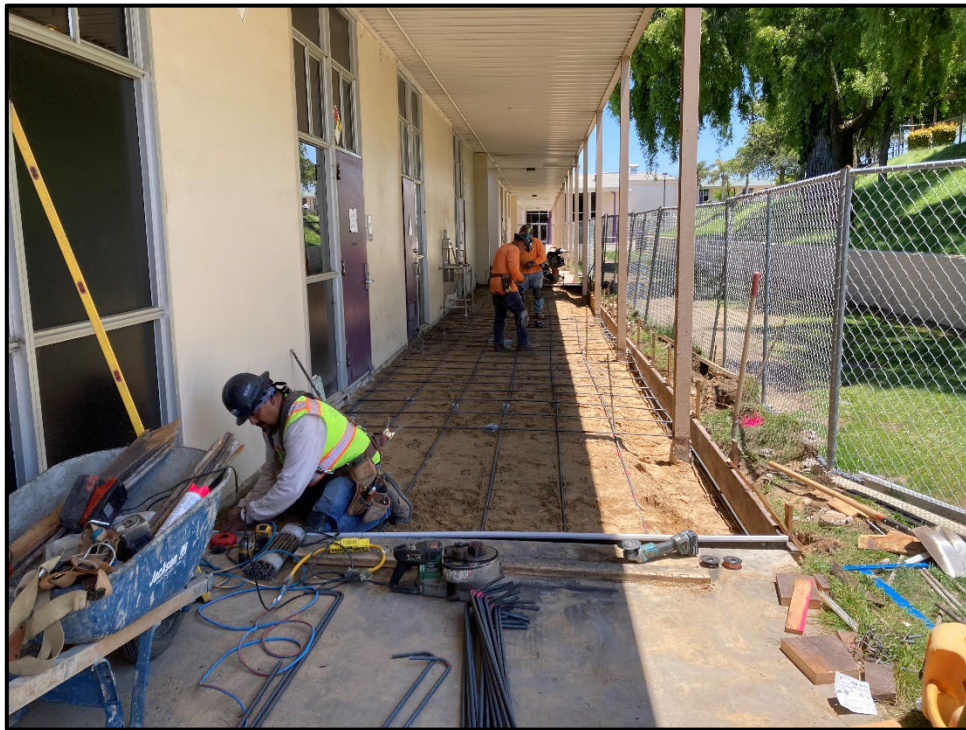
ERHS CTE Modernization – New ADA Compliant Walkways are Formed for Concrete
