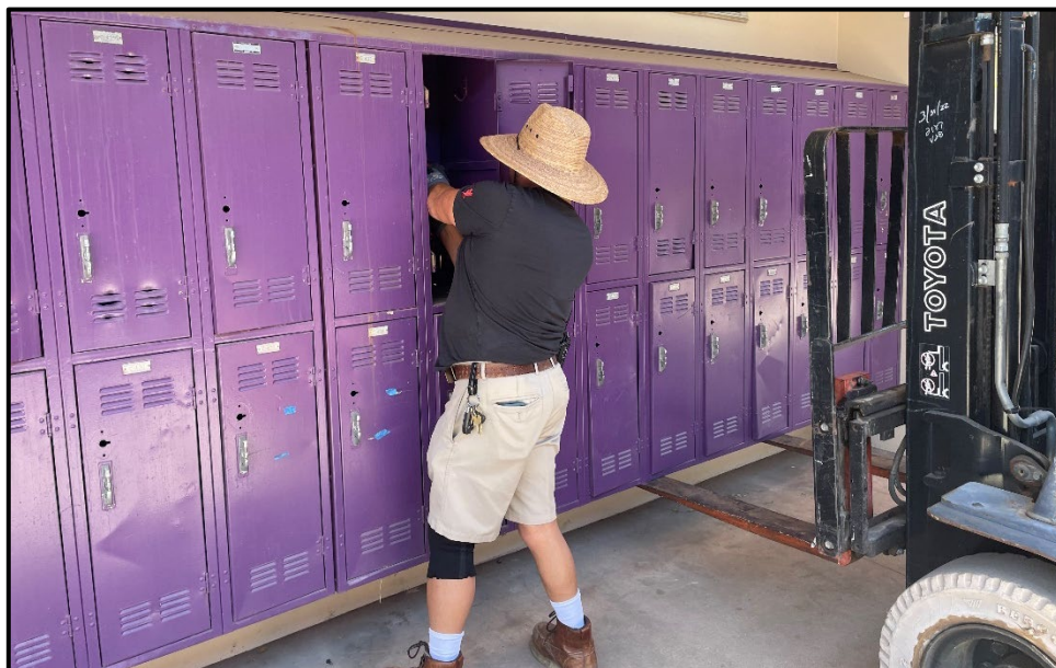
ERHS – Leo Avila Removing Obsolete Lockers
