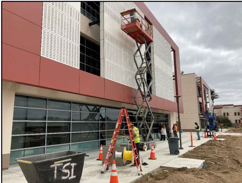
SMHS 50-Classroom Building – Sun Shade Panel Installation Continues
