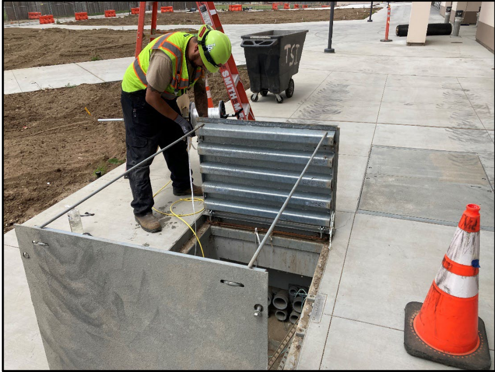
SMHS 50-Classroom Building – Communications Cable Pulling is Underway
