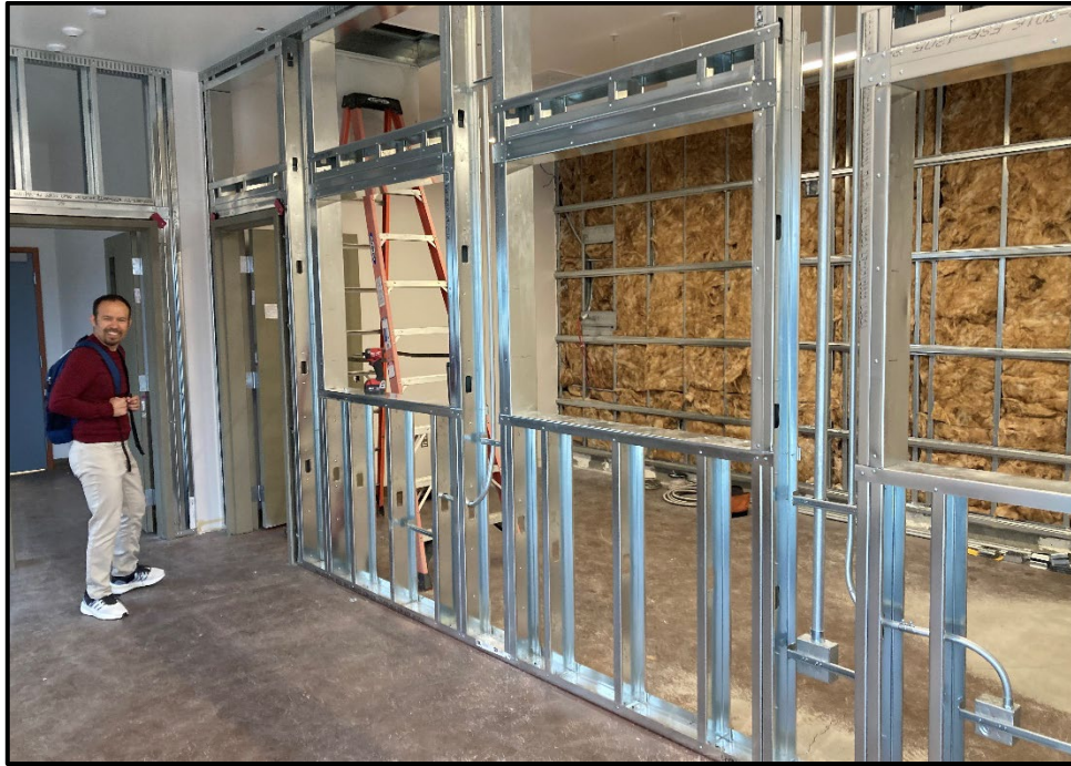
MRCTECAF Front Office Space – Wall Framing and Electrical “Rough-in” is Complete
