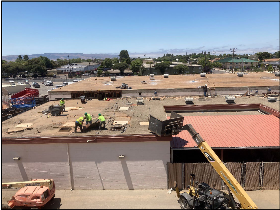
SMHS CTE Modernization – Roofing Demolition in Progress
