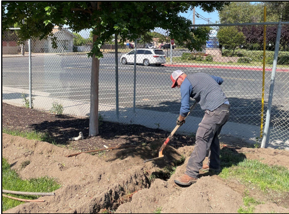
SMHS – Nick Canaan Installing New Irrigation Near the High Jump Area
