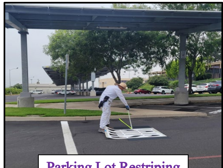
Parking Lot Restriping
