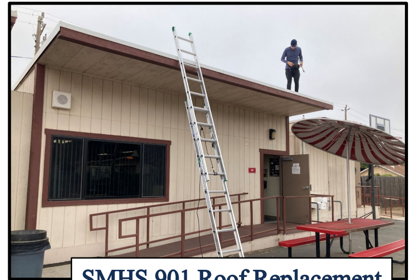
SMHS 901 Roof Replacement
