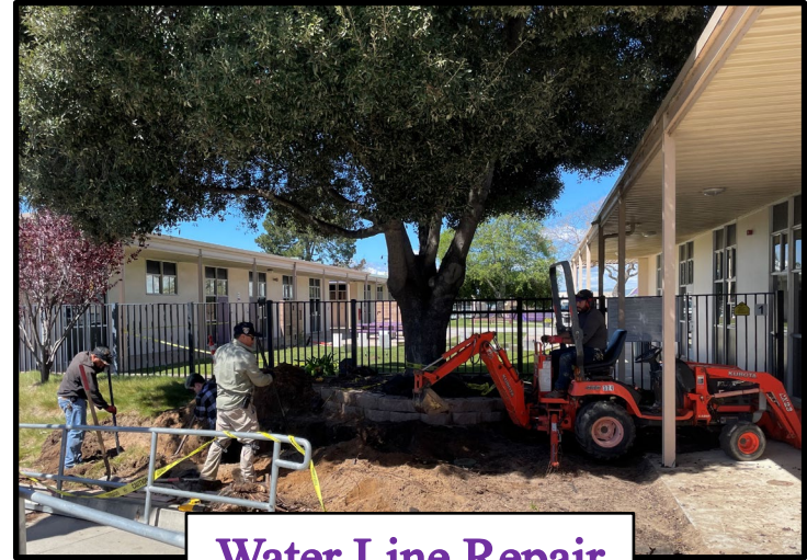
Water Line Repair
