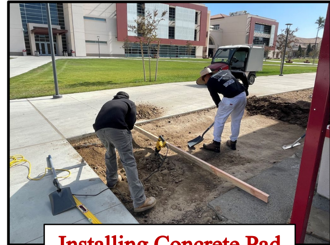
Installing Concrete Pad
