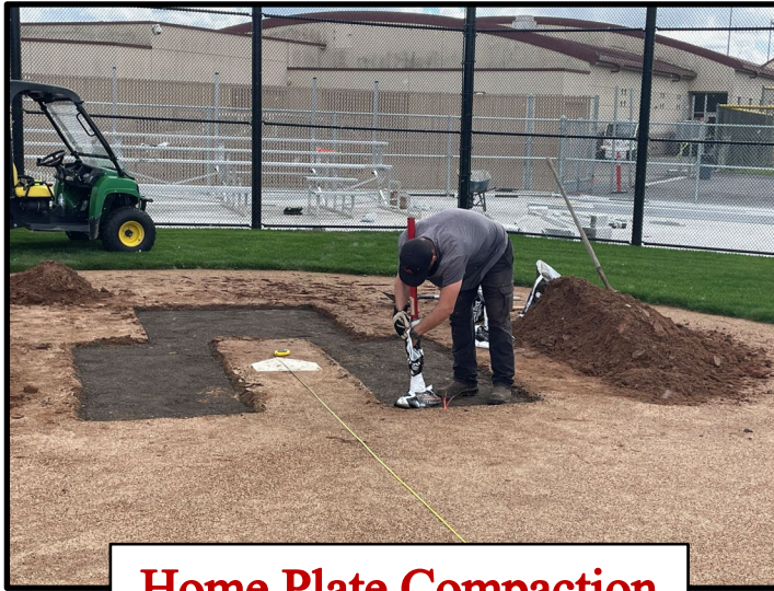
Home Plate Compaction
