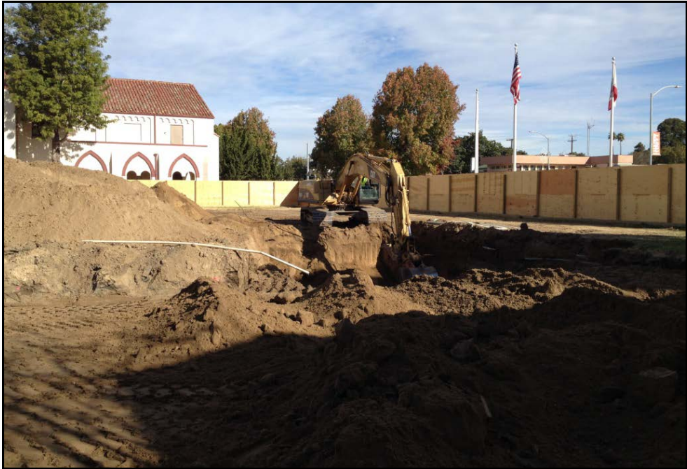
SMHS - Earth Work for Building Foundations is Underway
