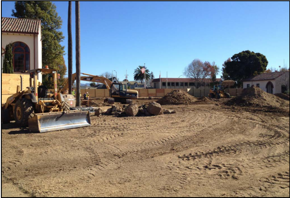
SMHS - 14-Classroom Building Construction Begins
