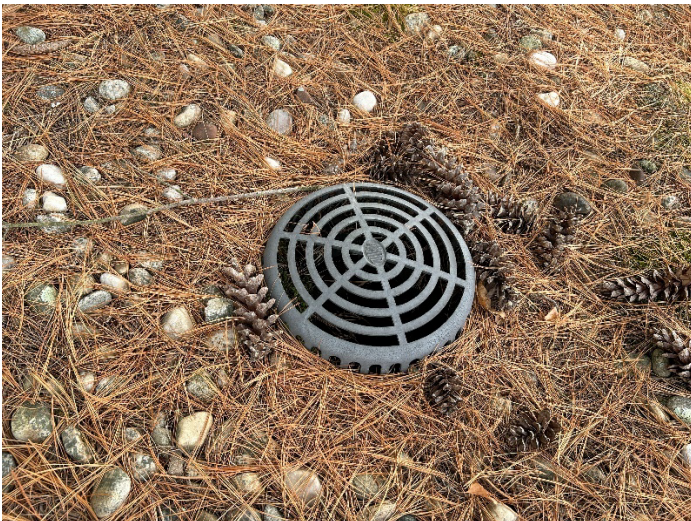
Typical roof drain – roof 1 (trees overhanging roof above)
