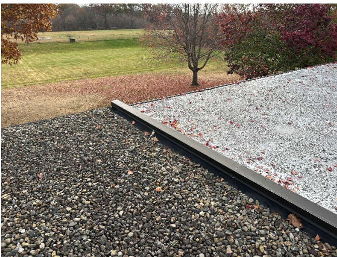
Roof transition between roofs 4 & 5
