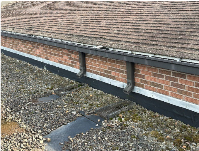
General condition of sloped roof & gutters/downspouts
