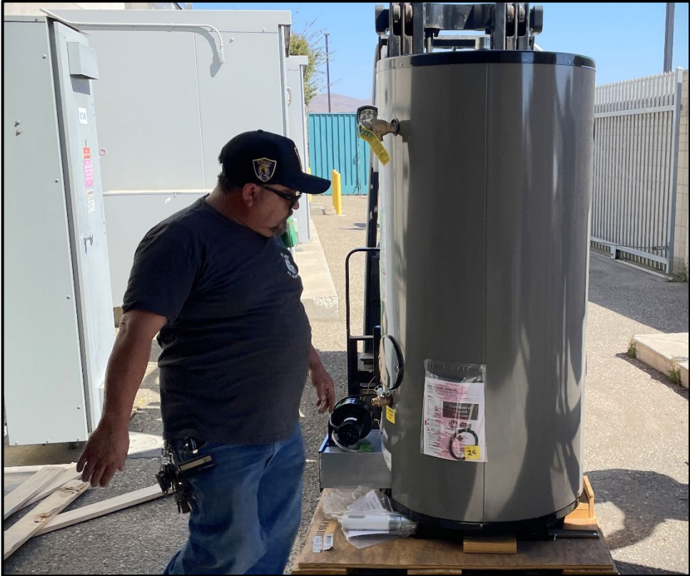
PVHS – Jesus Reyes Installing a New Water Heater in the Cafeteria
