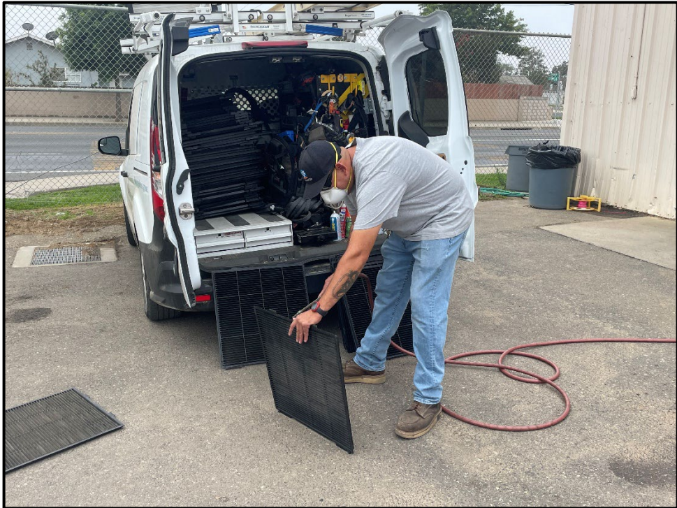
SMHS – David Velasco Cleaning the HVAC Air Filters
