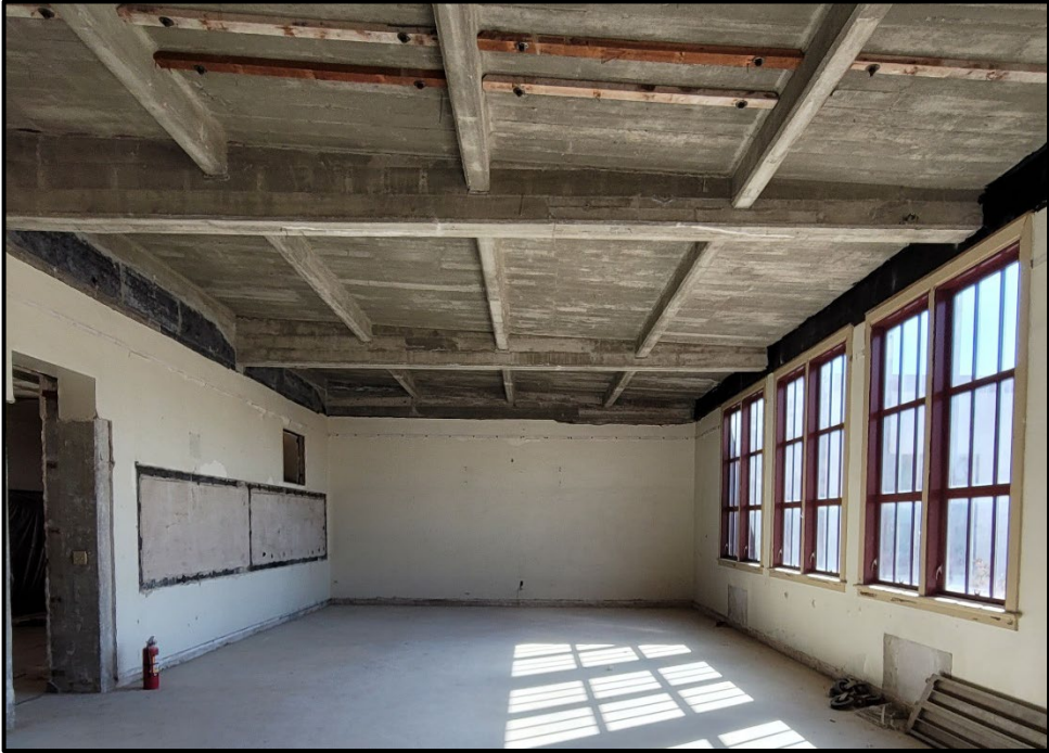
SMHS Admin to Classroom – Demolition Continues in the Old Administration Building
