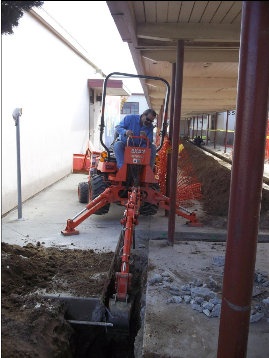
SMHS – José Placencia Trenches for the Natural Gas Line Relocation
