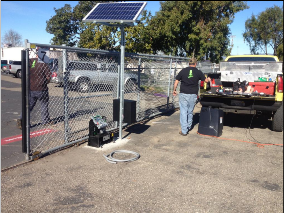
ERHS – The Newest Solar Powered Gate – Accessing the Pool Chemical Room
