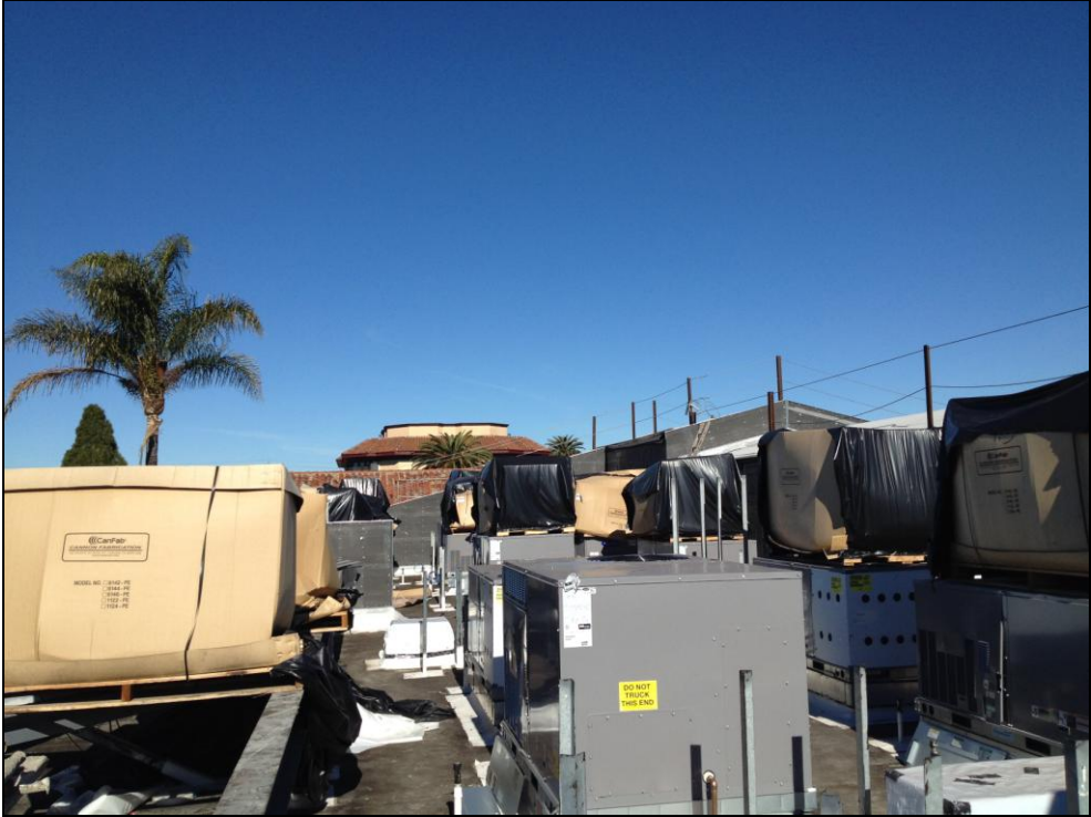
SMHS – Mechanical Well on the Broadway 14-Classroom Building Fills Up
