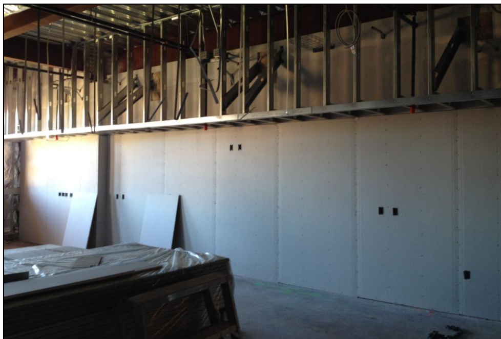
SMHS – Drywall Installation Continues in the Broadway 14-Classroom Building
