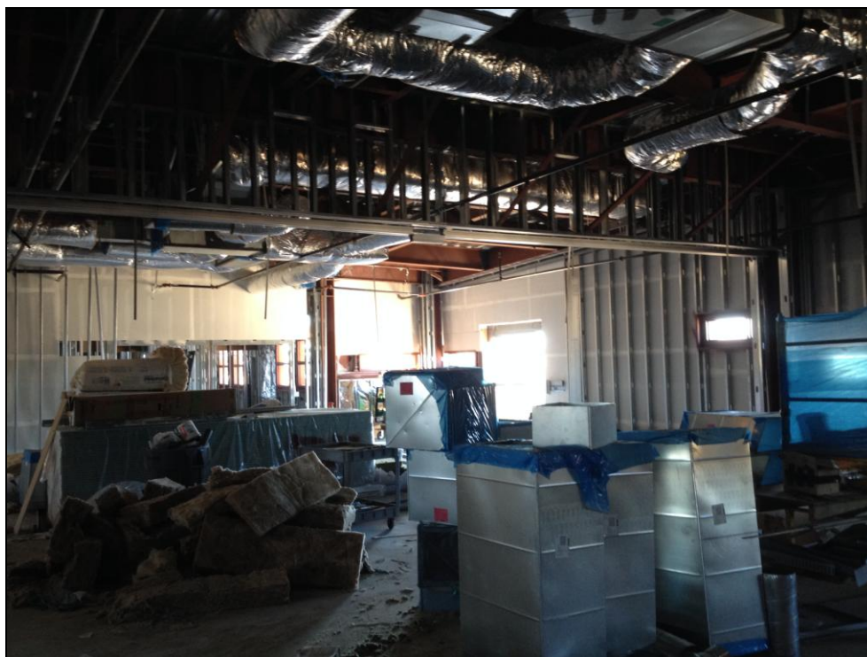
SMHS – Ventilation Equipment Staged for Installation in the Broadway 14-Classroom Building
