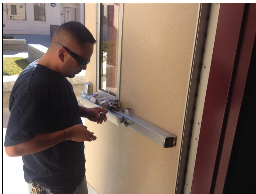
SMHS – Jimmy Salutan Installs the New Cyberlocks® lock Cylinders
