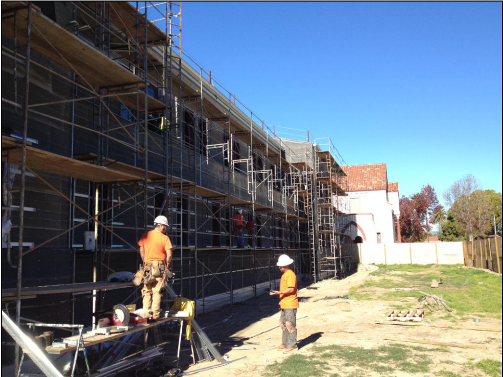
SMHS – 14-Classroom Building Window Flashing Installation in Progress
