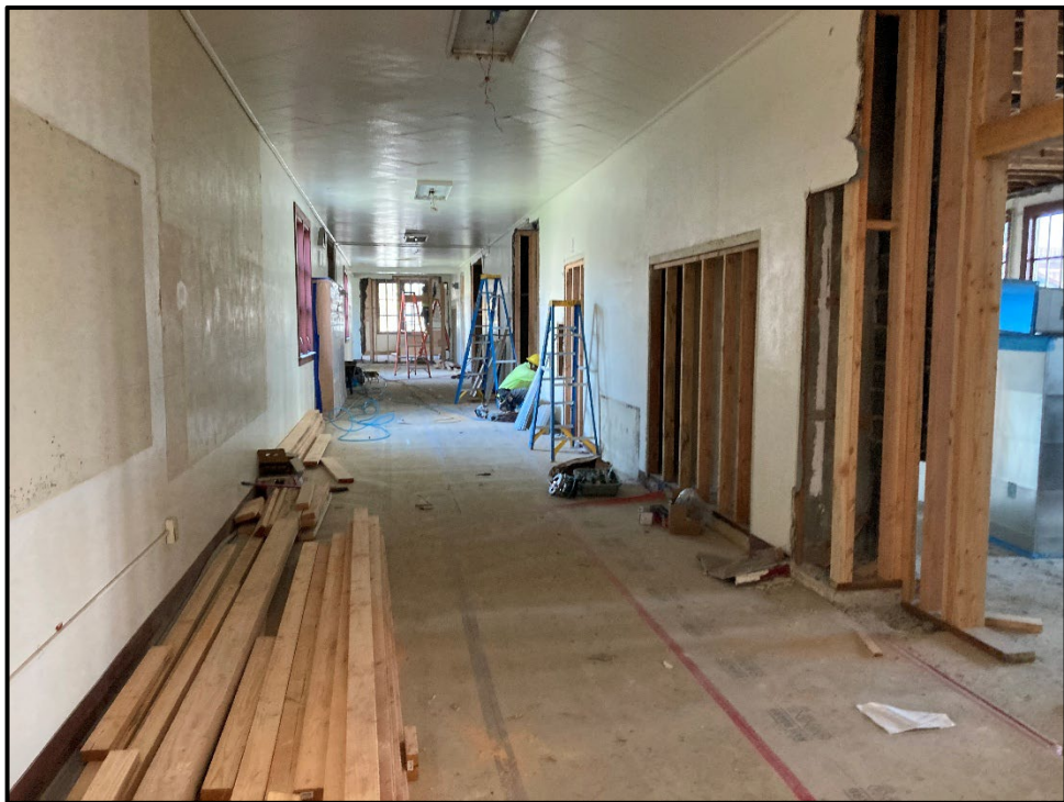
SMHS Admin to Classroom – Framing and Patching the Hallway Walls
