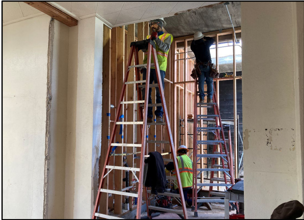
SMHS Admin to Classroom – Electrical Rough In Continues
