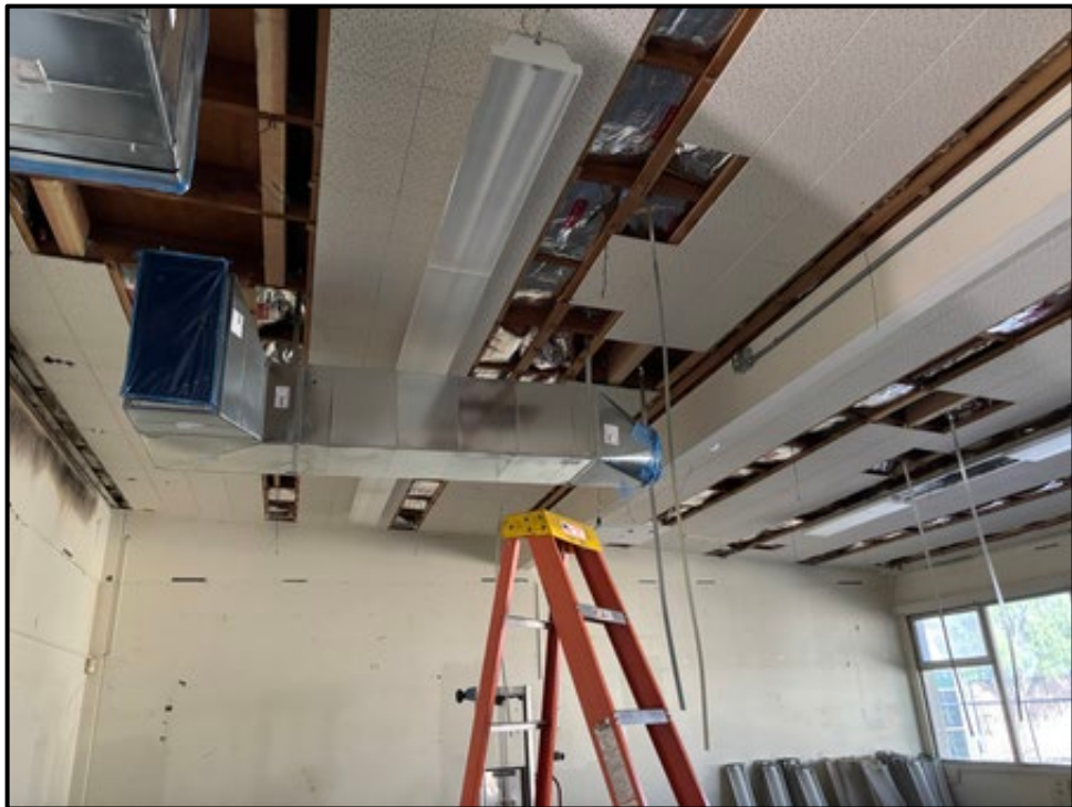
SMHS 37 Classroom – HVAC Ducting is Being Installed
