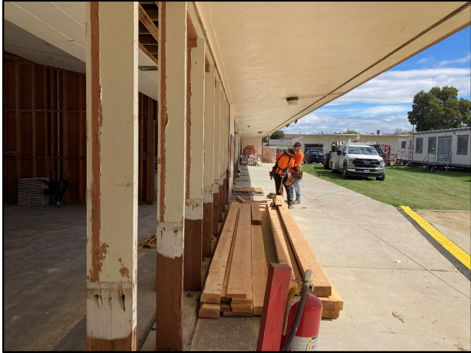
SMHS 37 Classroom – Framing of Sliding Glass Wall Begins
