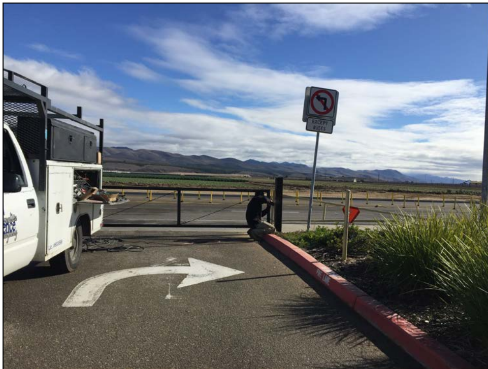
PVHS – New Gates Installed in Front of the School
