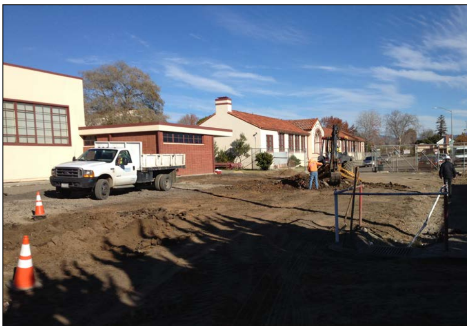
SMHS – ... and Will Become a New Visitor Parking Lot
