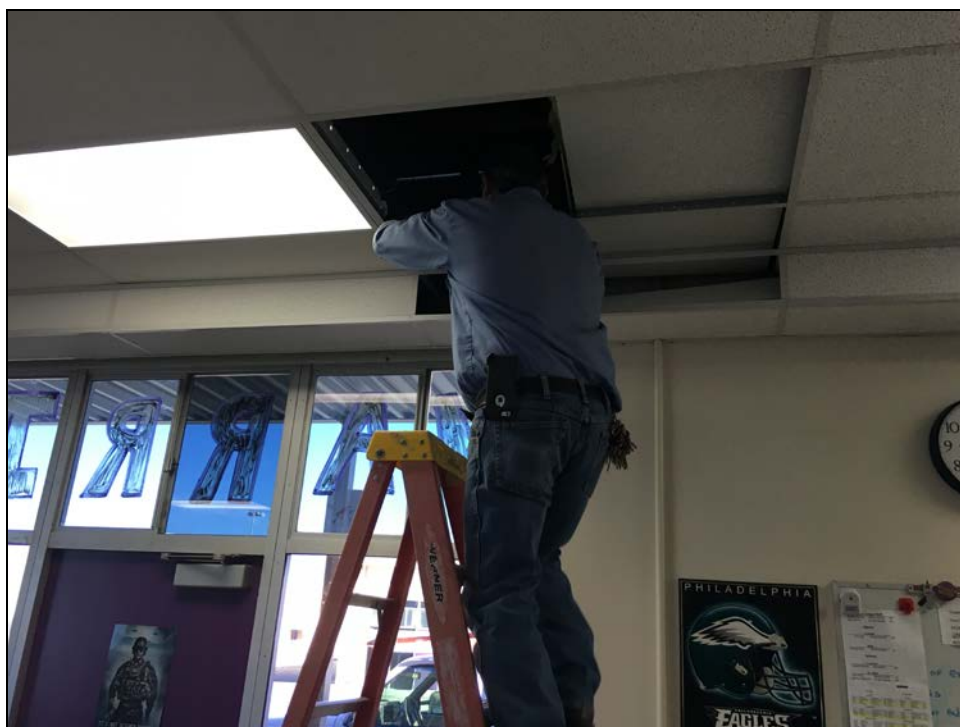
ERHS - José Placencia Installs Seismic Braces in Industrial Arts
