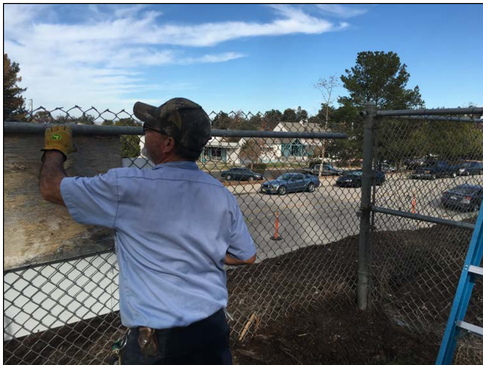
ERHS - Juan Rodriguez Repairs the South Fence Along Larch Street
