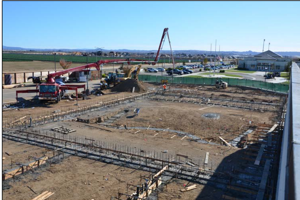
PVHS – Performing Arts Center Concrete Footing Pour Underway
