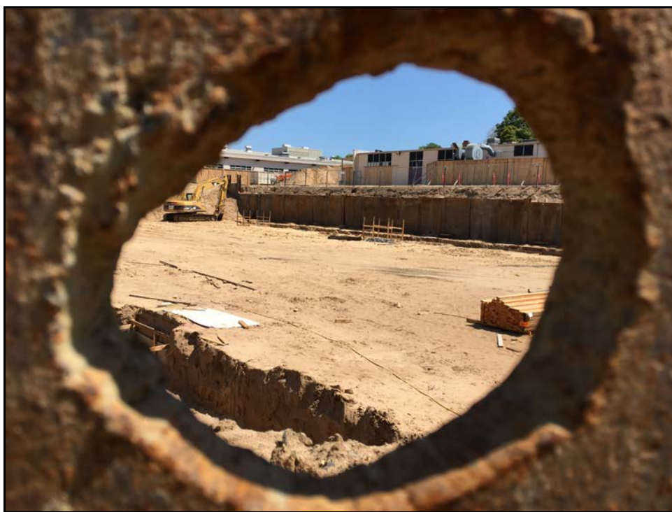
ERHS 38 Classroom Building – A Peek at the Construction Site Through Sheet Piling
