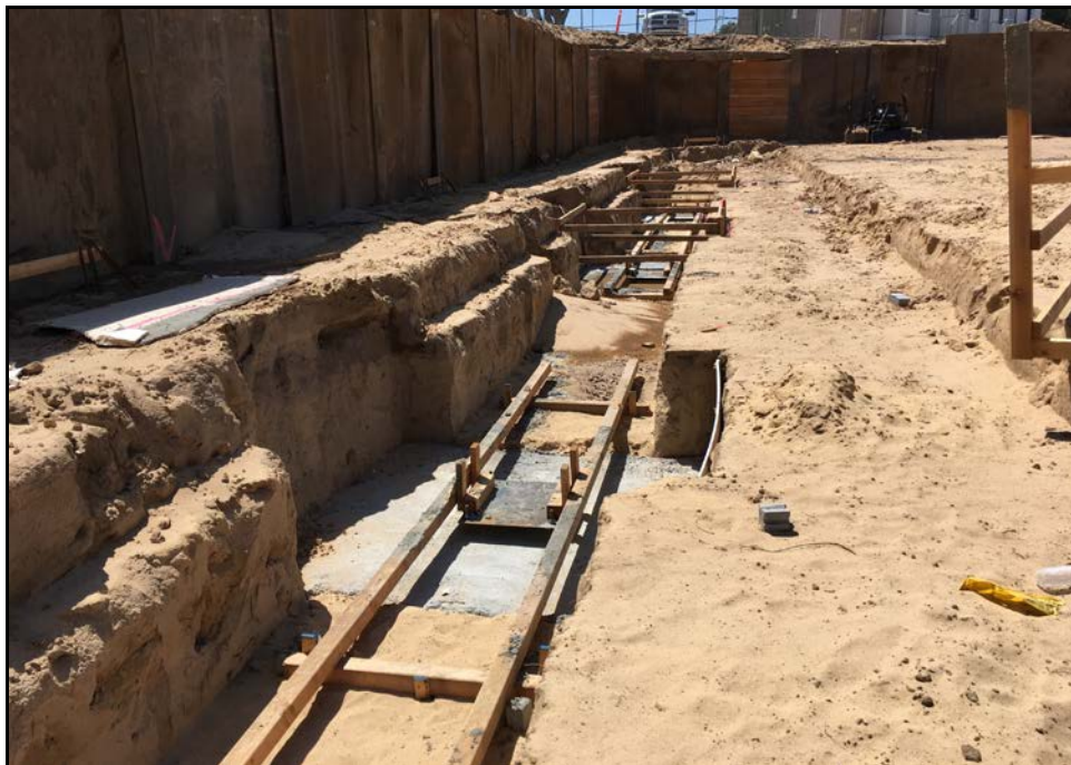
ERHS 38 Classroom Building – Concrete Footings Poured and Curing
