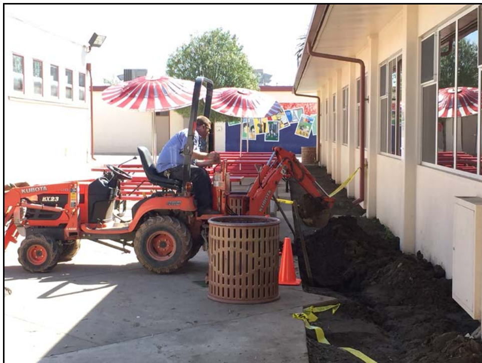
SMHS - Erik Fulton Investigates Math Building Heating Leak
