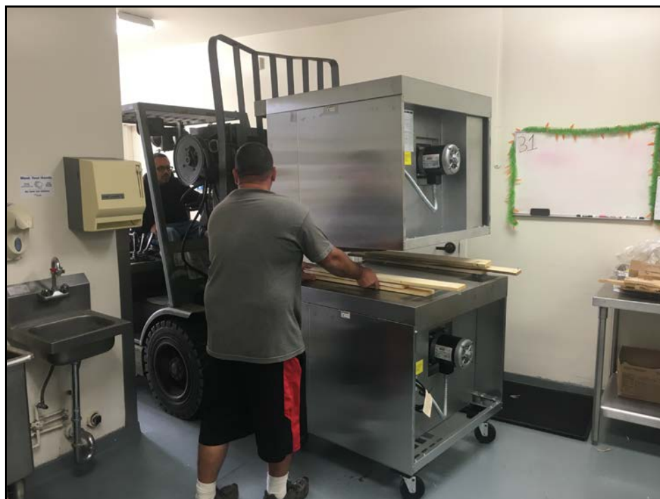
ERHS – Jimmy Salutan and Mike Roberson install new Convection Ovens in the Cafeteria
