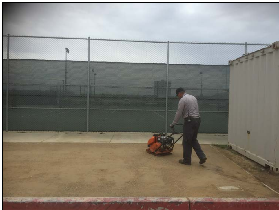
PVHS - José Gamino Prepares a New Pad for ASB Storage Container
