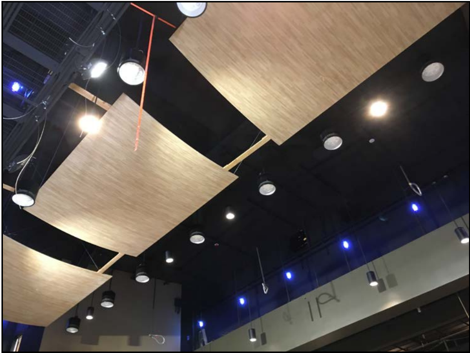
PVHS Performing Arts Center – Interior Lighting and "Sound Clouds" Installed
