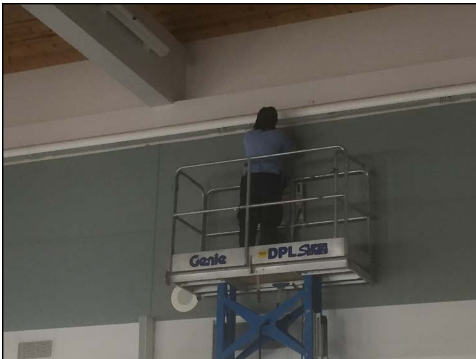
PVHS - Jennifer Abend Replaces Lights in the Cafeteria
