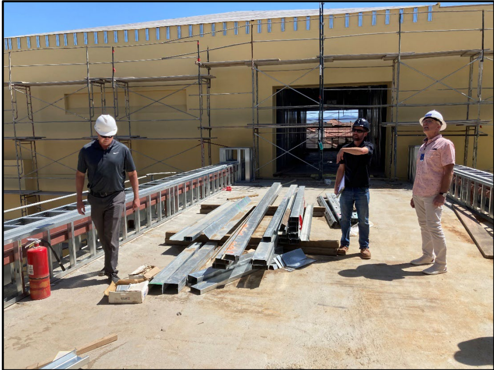
SMHS 50-Classroom Building – Architects Review Progress from the Third Floor Bridge
