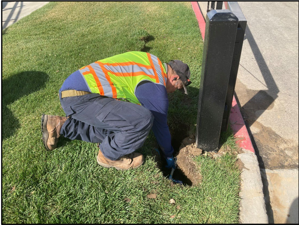
PVHS – Matt Schlereth Repairing a Broken Sprinkler Line
