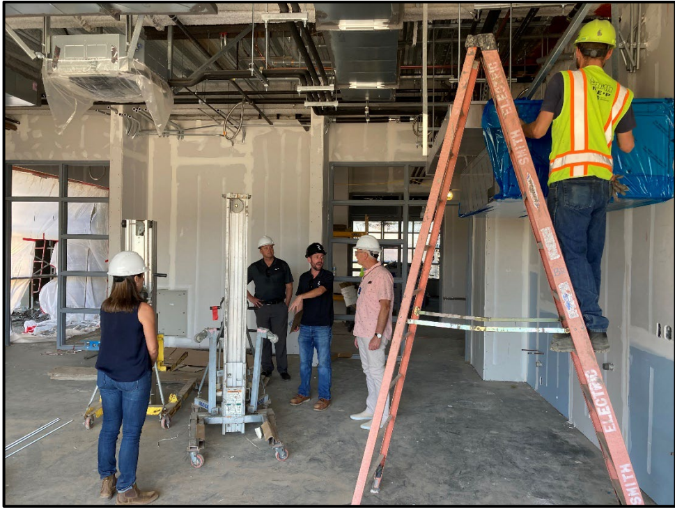
SMHS 50-Classroom Building – Foods Lab Ventilation hood Installation is Underway
