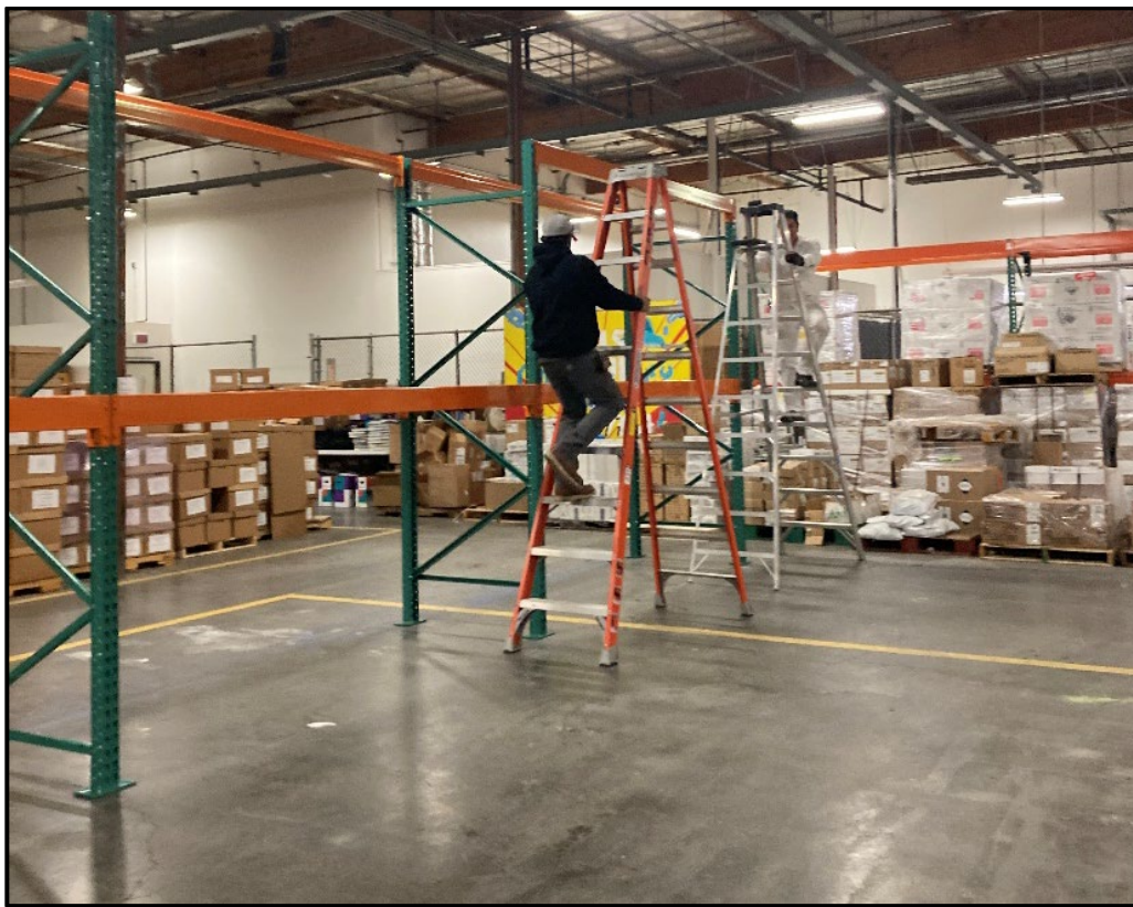
SSC – Tom Harbold and Joel Amezcua Installing Warehouse Pallet Racks
