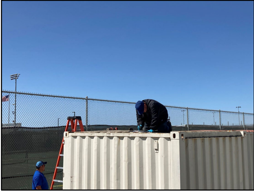
PVHS – Paul Alvarez Installing a Turbine Roof Vent
