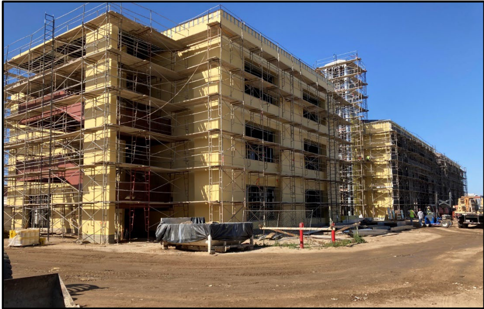
SMHS 50-Classroom Building – Exterior Received Stucco
