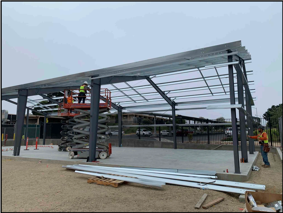
ERHS Maintenance and Operations Building – Roof Framing Defines the Size of the Shop
