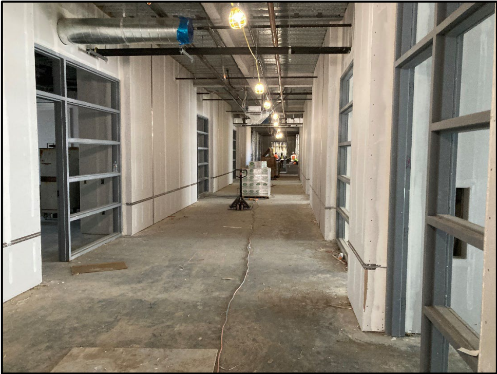
SMHS 50-Classroom Building – Classroom Windows and Doorways Frame the Interior Hall
