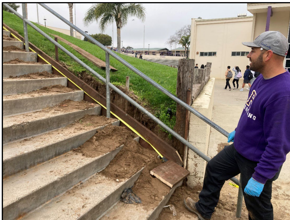
ERHS – Jordan Markstone Repairing the Stairs for Erosion Control
