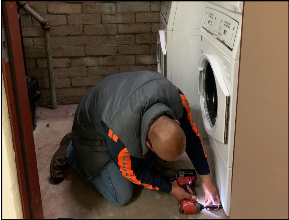
SMHS – Alex Anguiano Installing a New Washer and Dryer in the Wilson Gym
