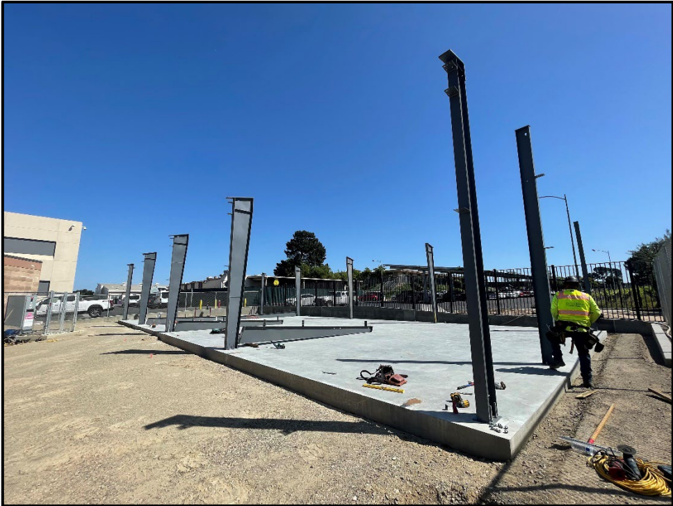
ERHS Maintenance and Operations Building – Structural Steel Begins to Sprout from the Floor
