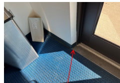
Damaged gyp. board wall and loose wall base.
