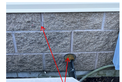
Masonry repairs / seal wall penetration
