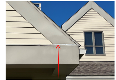
Existing metal trim repair
