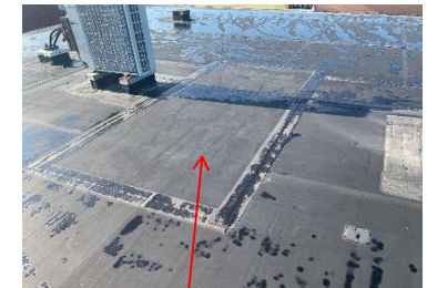
Large roof repair
