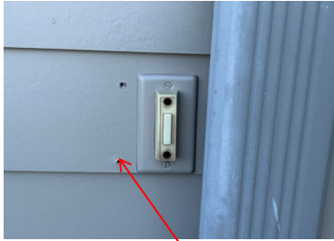
Repair / seal wall
