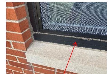
Repair joint sealant at window.
