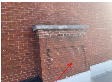
Masonry repairs and staining.
