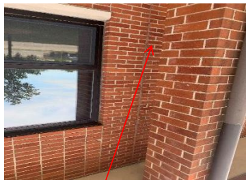
Reseal masonry joint.
