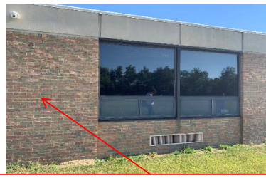
Rough brick at middle section of wall. Cracking and popping.
