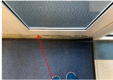
Repair door threshold.
