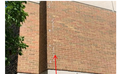
Masonry - repair / tuck point.
