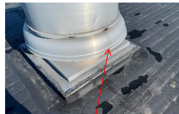
Damaged roof vent. Need to repair caulk joint.
