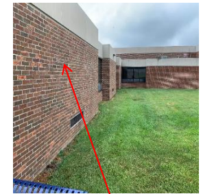
Masonry - repair / tuck point.
