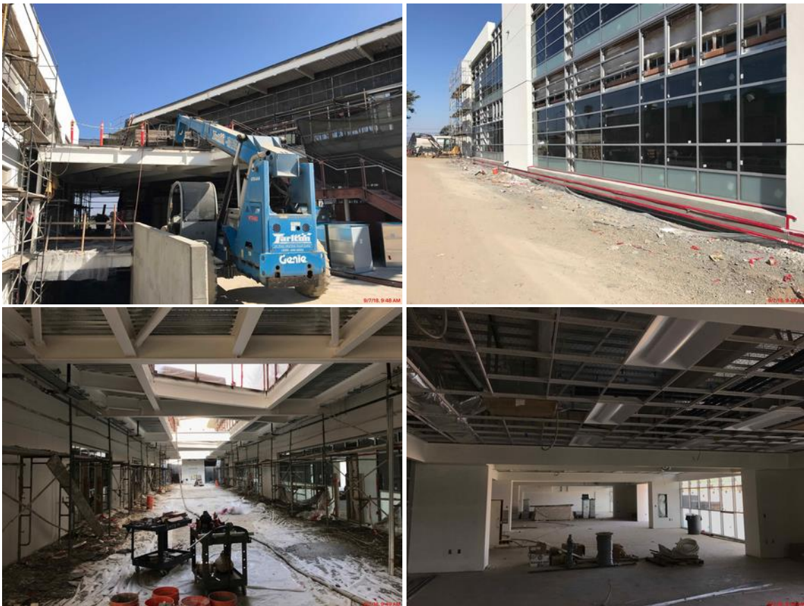
Righetti High School New 38 Classroom Building Construction Progress (September 2018)
