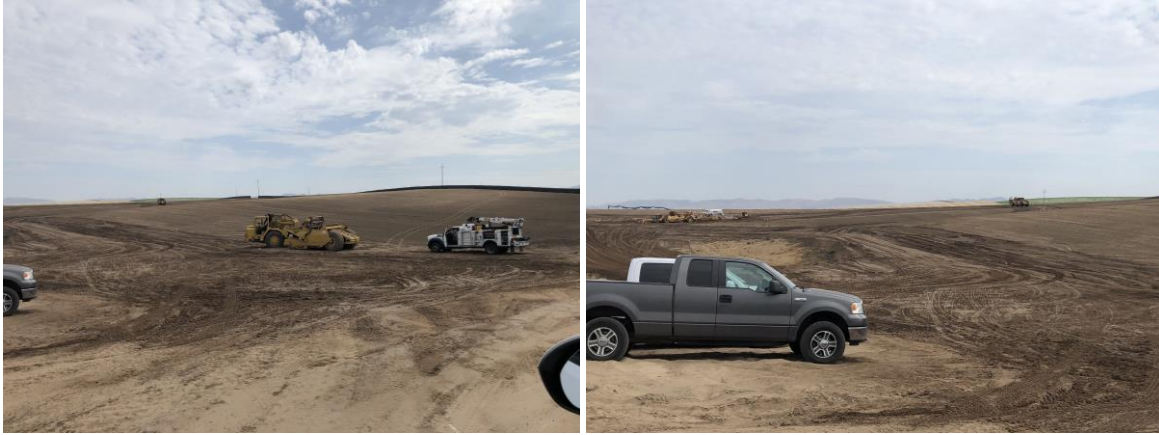
Rough grading of the CTE Center/Ag Farm begins (July 2018)
