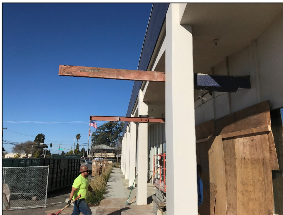
SSC Canopy Removal – Underlying Structure of the Canopy is Exposed
