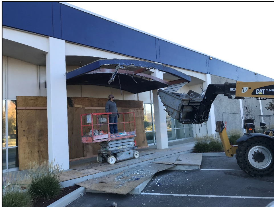
SSC Canopy Removal – The Old Building Entrance Canopy Removal is In-process
