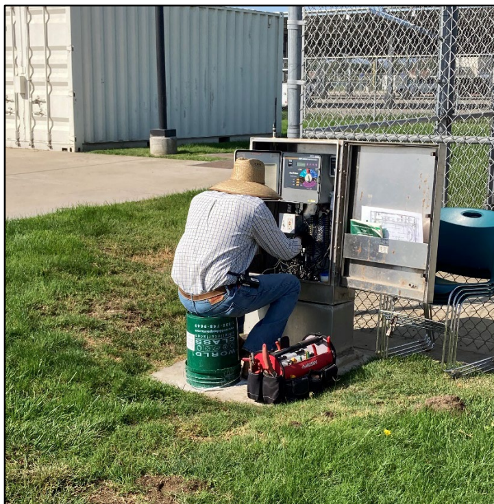
PVHS – José Gamino Repairs the Stadium Irrigation Clock Wiring
