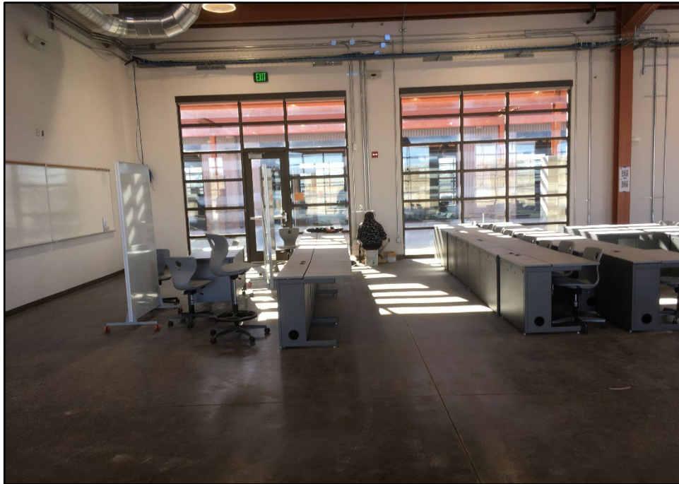
CTE / Ag Center – A Technician Installs Data Ports in the Shop Buildings
