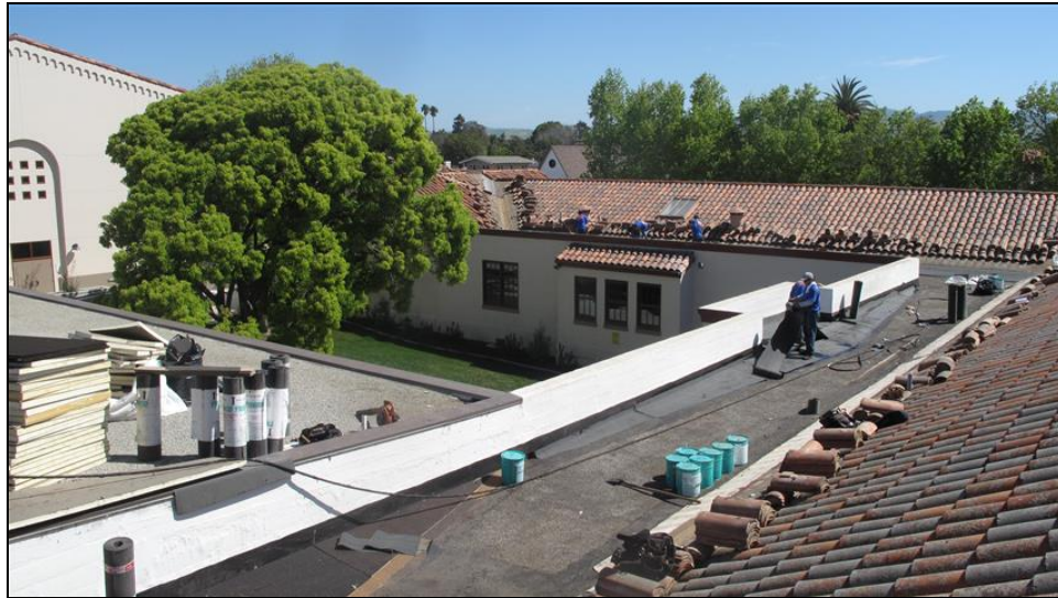
SMHS – Administration Building Roof Repairs are Underway
