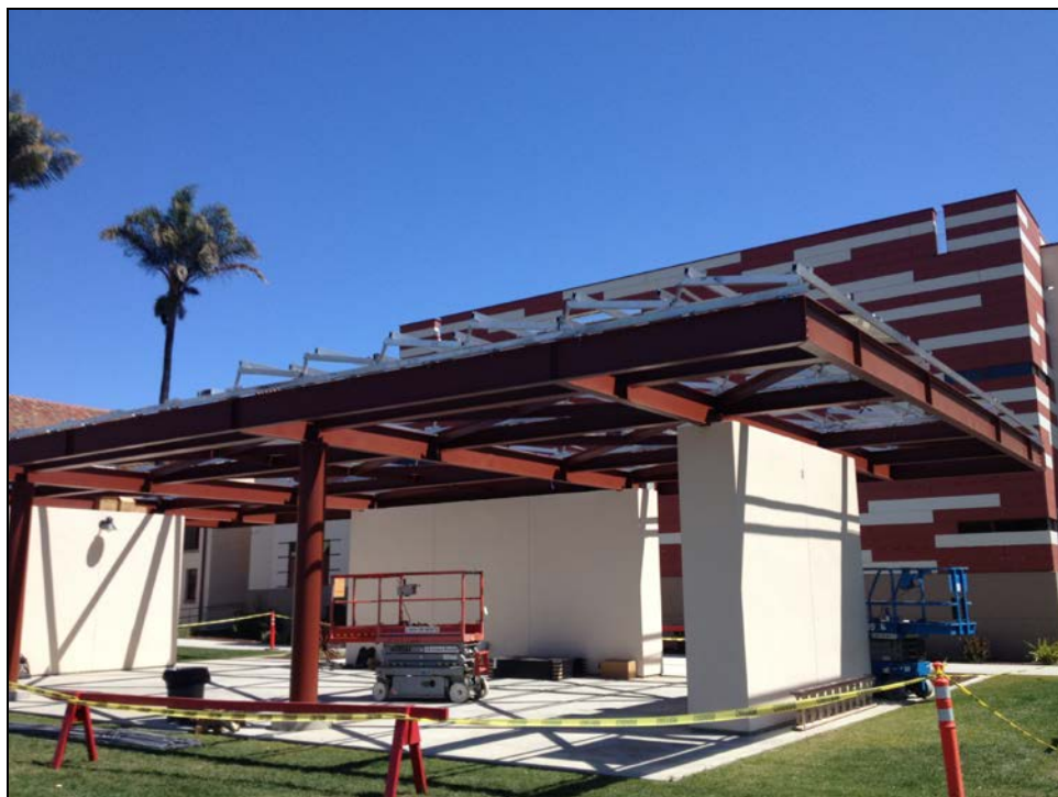
SMHS – Solar Panel Installation Beginning at the Broadway Classroom Building
