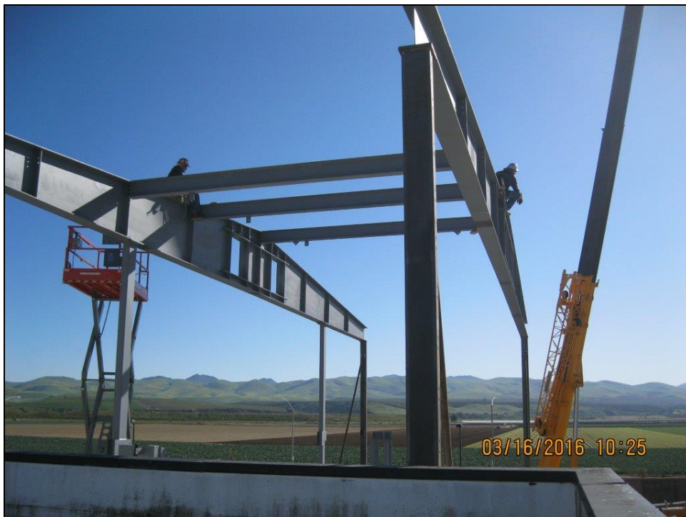
PVHS – Performing Arts Center Structural Steel Assembly Begins
