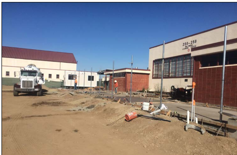
SMHS – Concrete Walkway Installation for the New Parking Lot
