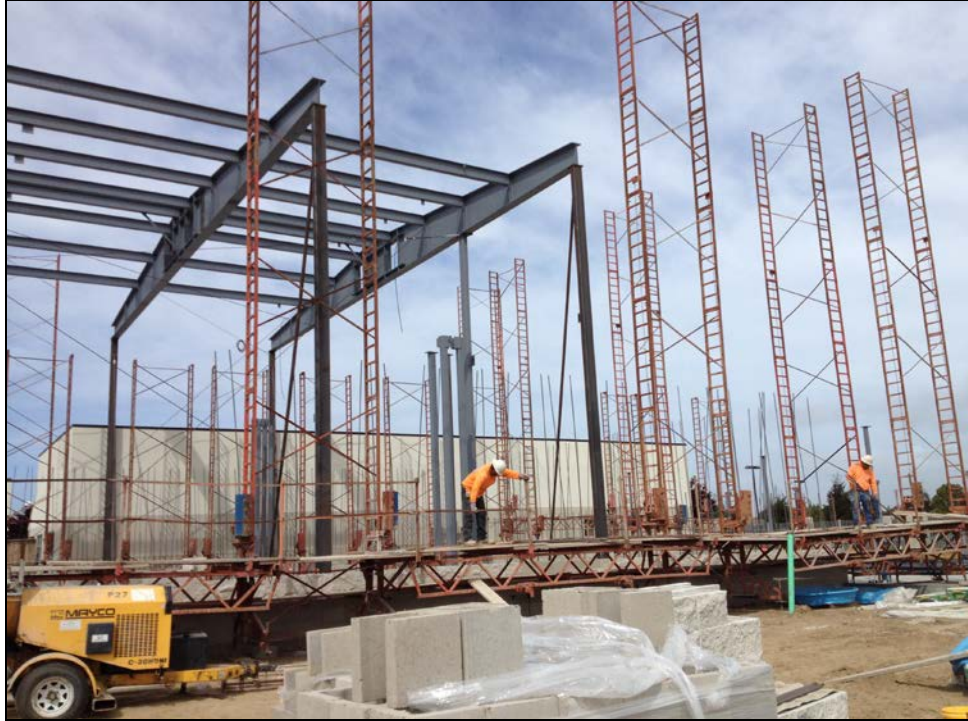
PVHS - Scaffolding is Assembled for Block Wall Installation
