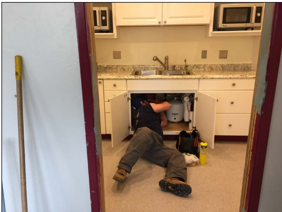
ERHS – Flavio Rodriguez Completes the Plumbing in the Revised Staff Kitchen
