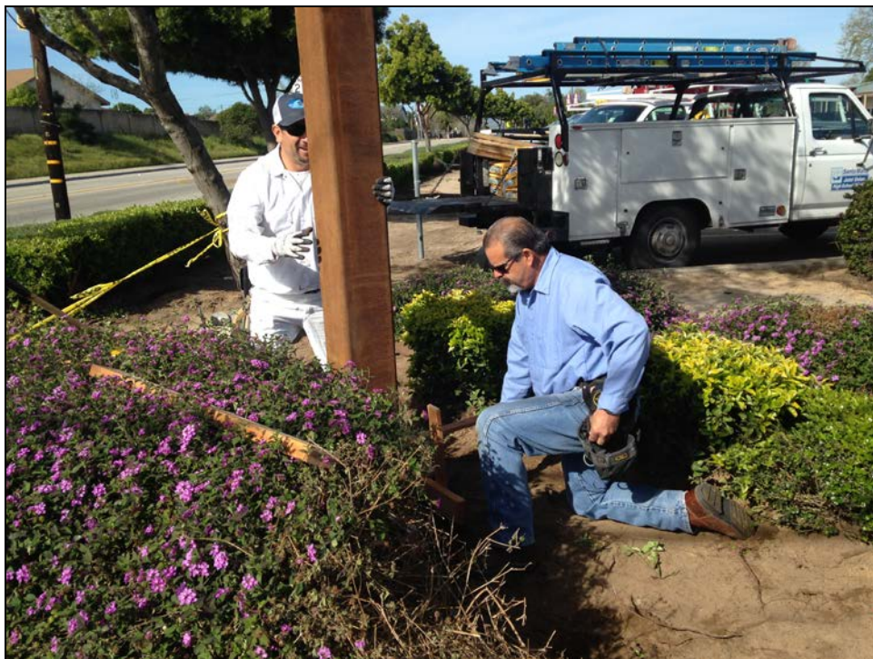
ERHS – Ernest Paz and José Placencia Erect Supports for the New Marquee at Foster Road and Bradley Road
