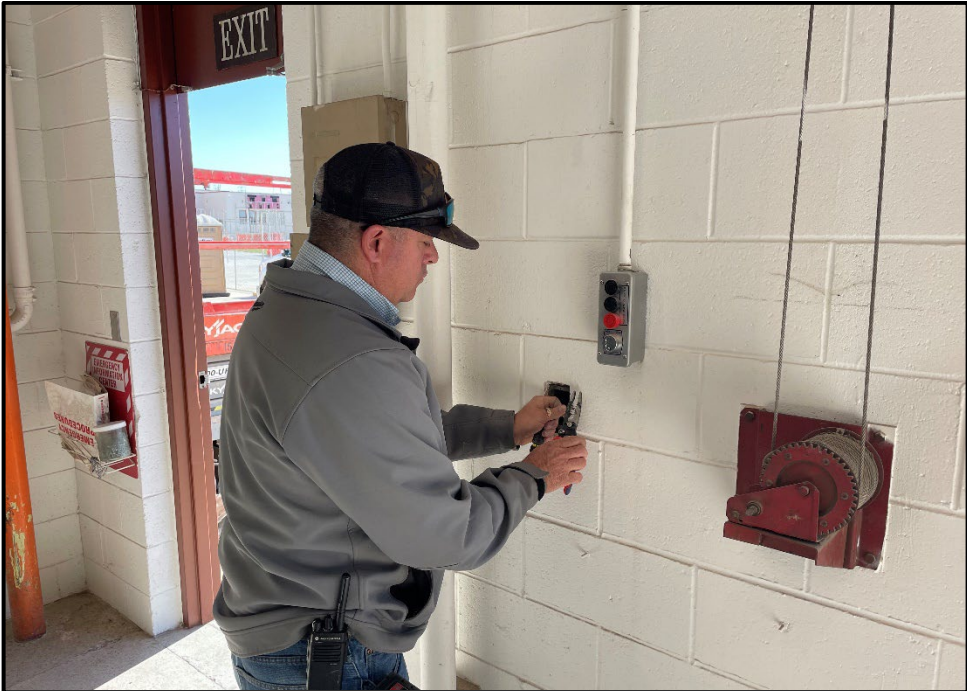
SMHS – Andy Freitas Replacing Electrical Outlets in Classroom 511
