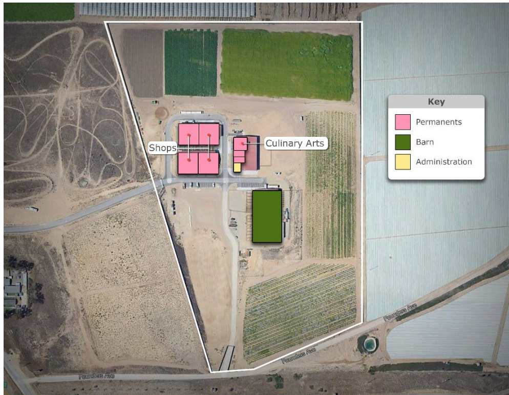
Figure 10: CTE Center Existing Conditions
