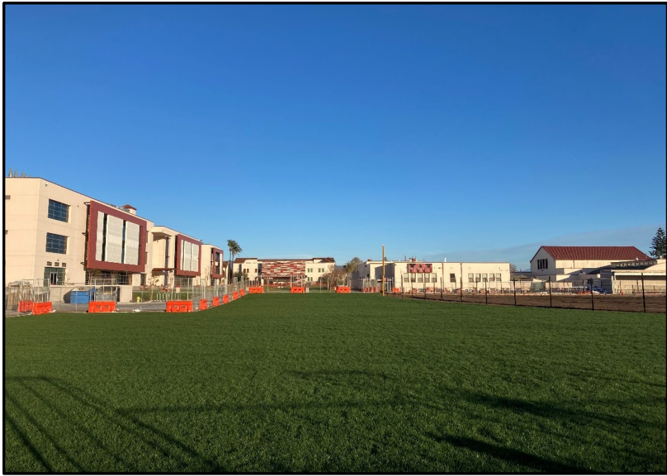
SMHS Reconstruction – Sod Installation is Complete
