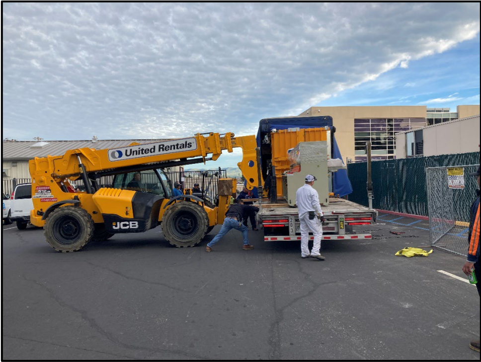
ERHS CTE Modernization – Metal Shear is Delivered for the Welding Shop
