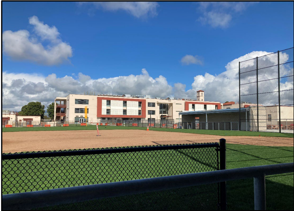
SMHS Reconstruction – New Softball Fencing is Installed
