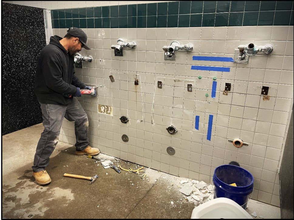
PVHS – Tom Harbold Removing Damaged Restroom Tiles
