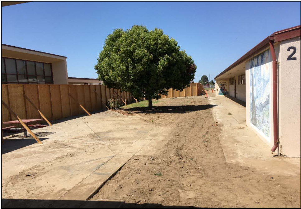
SMHS Reconstruction – Underground Utilities Buried and Construction Fencing In-place
