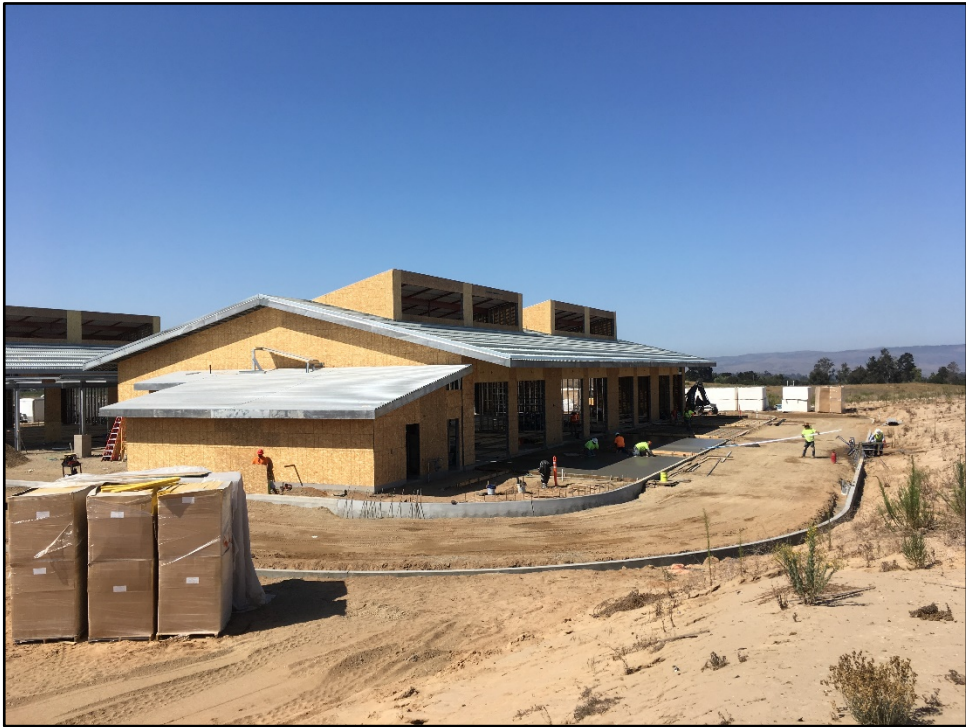
CTE Ag Center - Road Curbs Poured and Shop Driveways In-Progress
