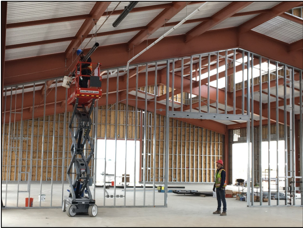
CTE Ag Center - Plumbers Install Pipe in Shop Buildings
