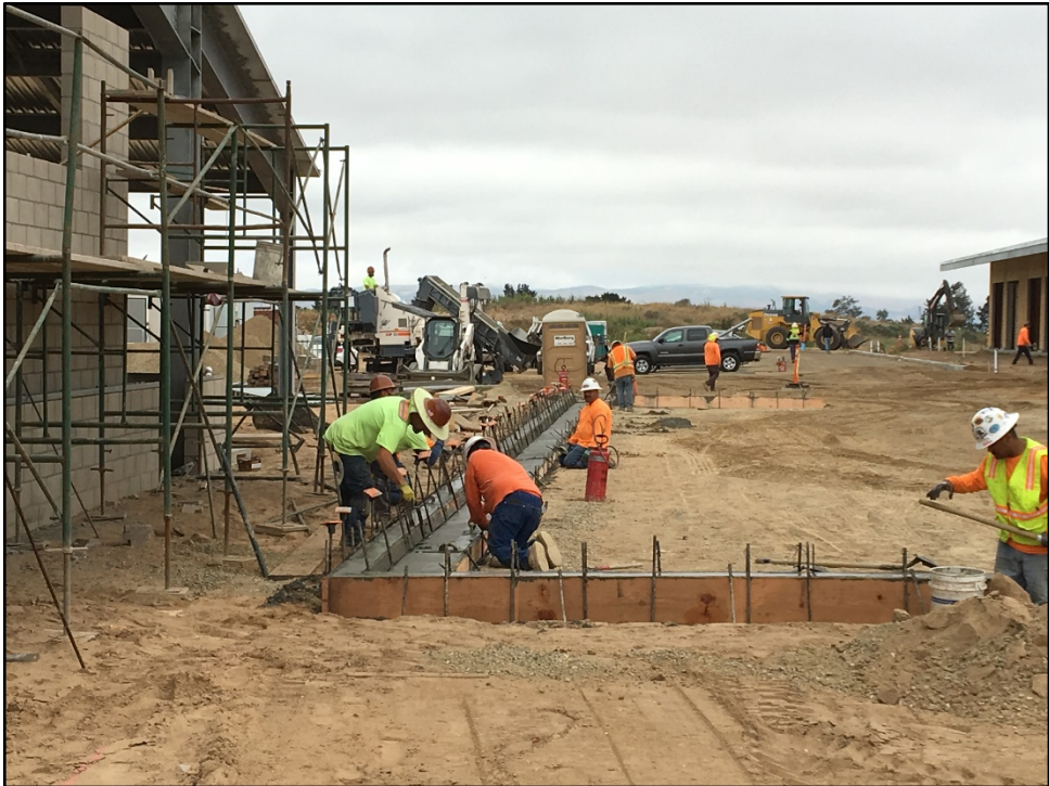
CTE Ag Center – Curbs are Formed and Poured for Parking Area
