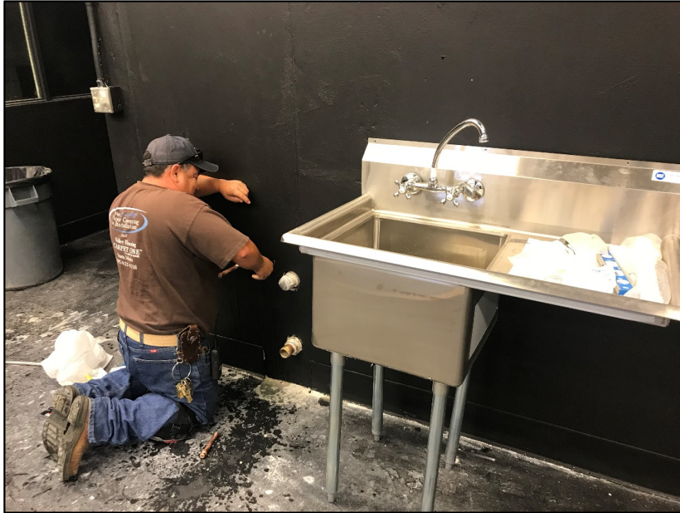
ERHS – Jesus Reyes Replaces the Sink in the Drama Classroom
