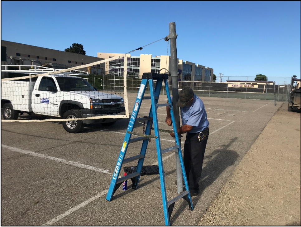
ERHS – Juan Rodriguez Installs New Outdoor Volleyball Nets
