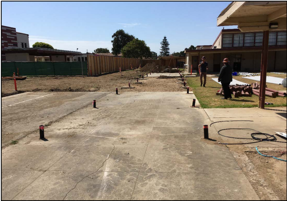
SMHS Reconstruction – Facilities Planner Marybeth Gallas Inspects the Demolished Walkway
