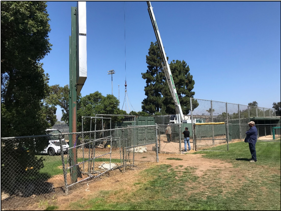
ERHS – Bernie Rayner Oversees Setting of New Storage containers for Baseball
