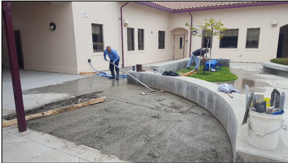
DHS - José Placencia Finishes Concrete Walkway in the Quad
