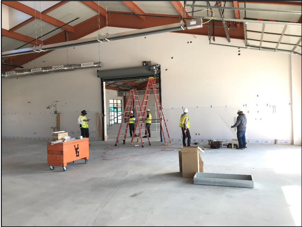
CTE Ag Center – Roll-up Door Installation in the Shop Building
