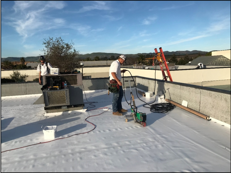
PVHS – Modular Classroom Roofs Received Seam Welded Tri-Polymer Alloy (TPA) Roofing
