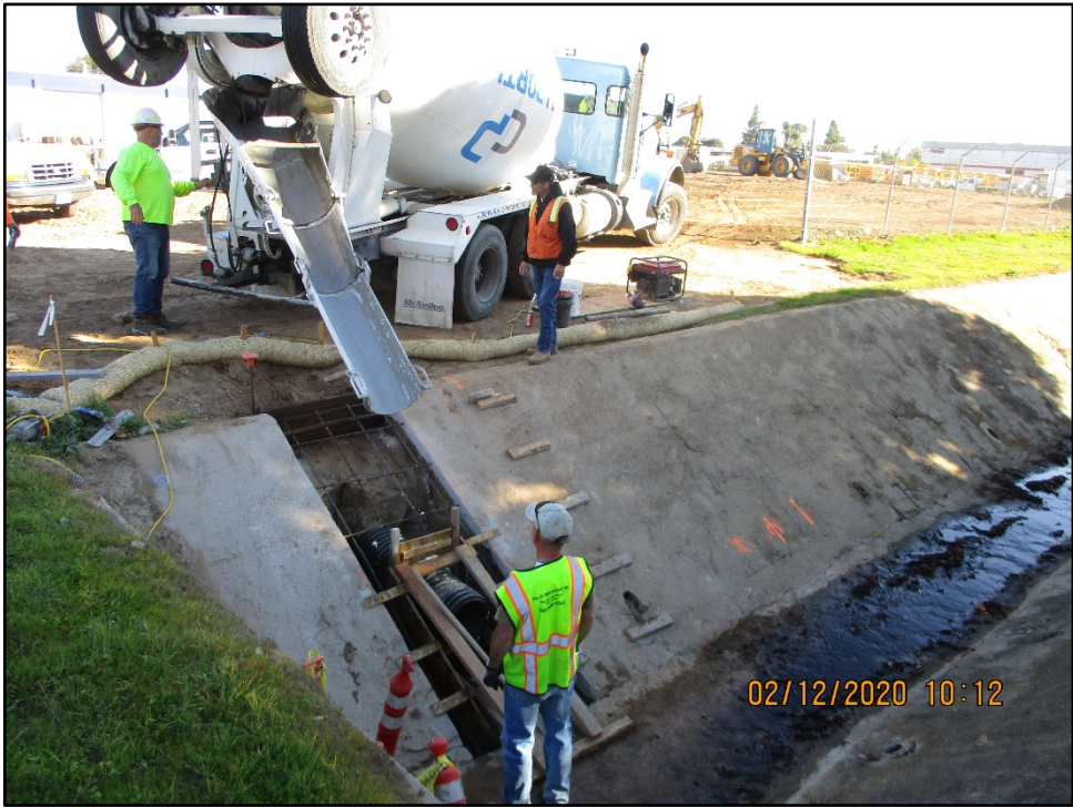
SSC West Parking – Detention Basin Overflow Drain Installation
