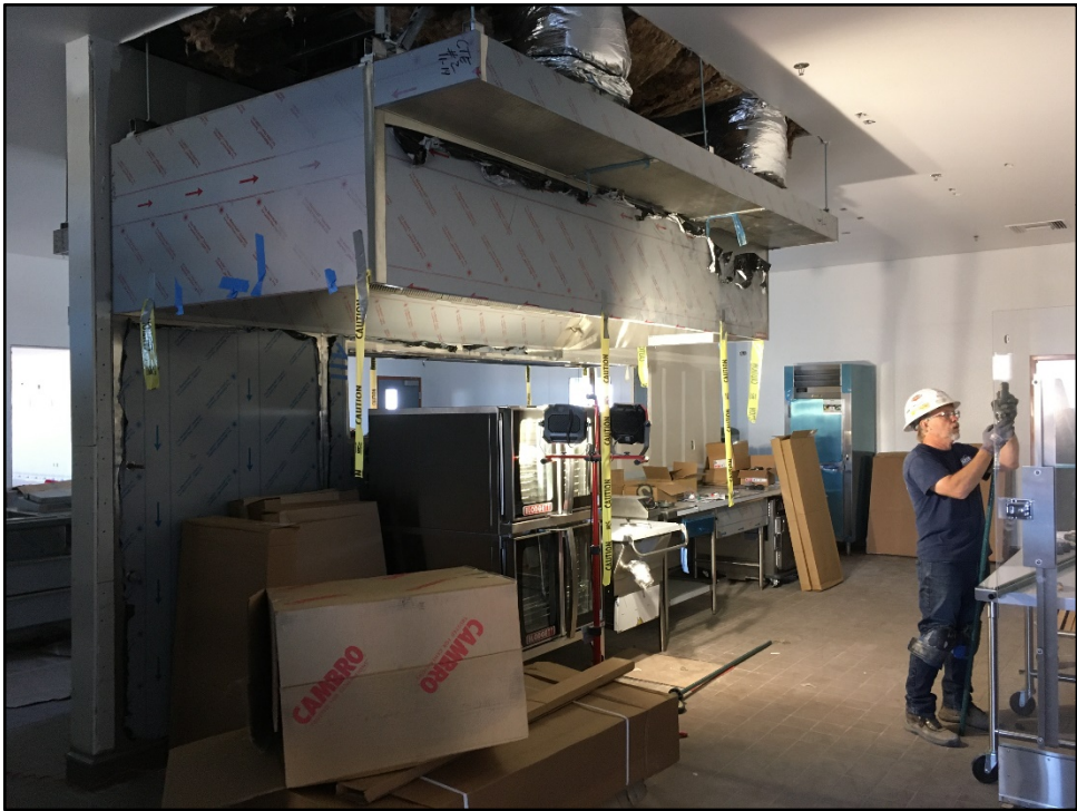
CTE Ag Center – Culinary Arts Kitchen Equipment Installation Underway
