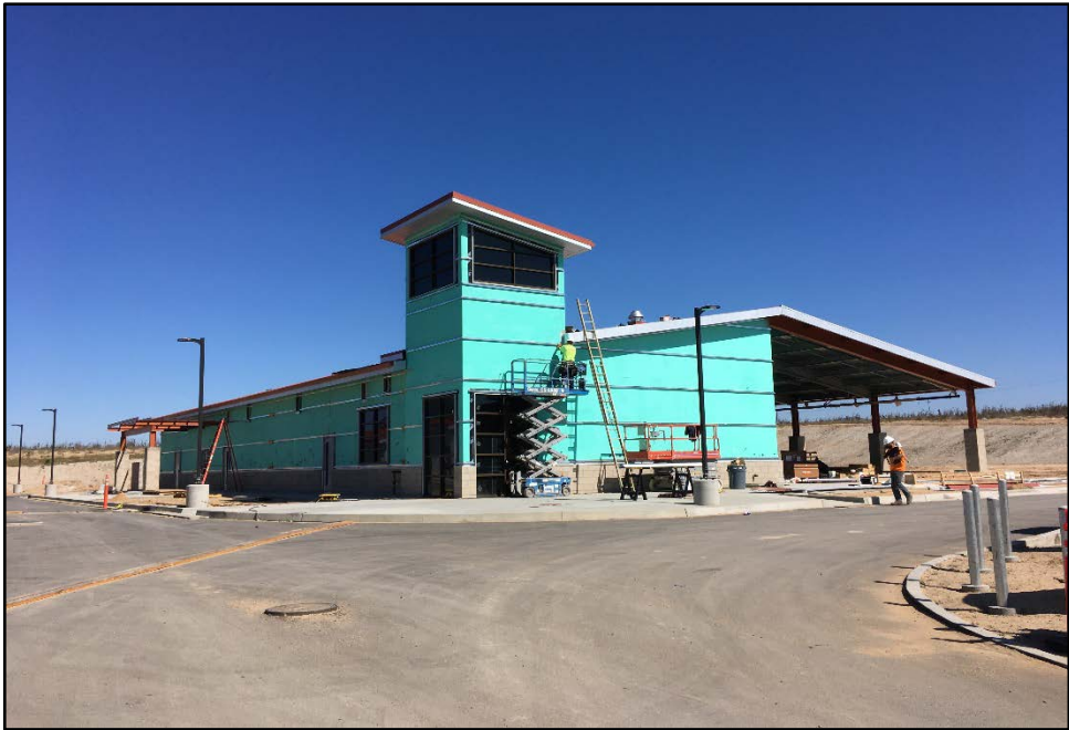
CTE Ag Center – Culinary Arts Siding Installation In-progress
