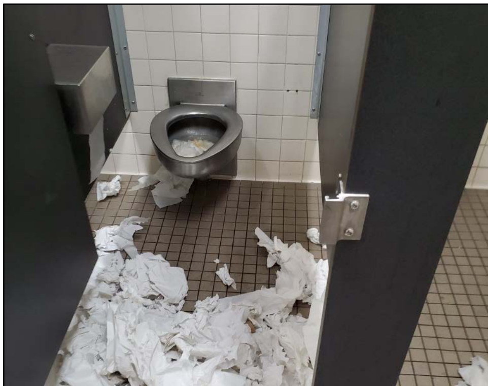
SMHS – Vandalism in the Boys' Locker Room Student Restroom
