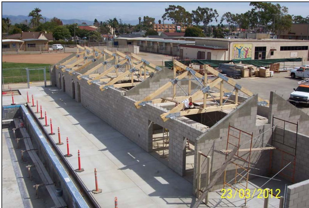
SMHS Pool Building Trusses Arrive!
