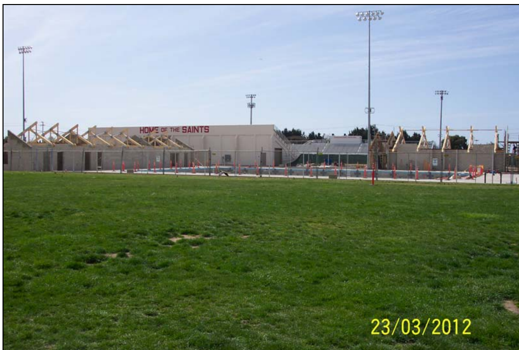
SMHS Pool – Long Shot of the Whole Project
