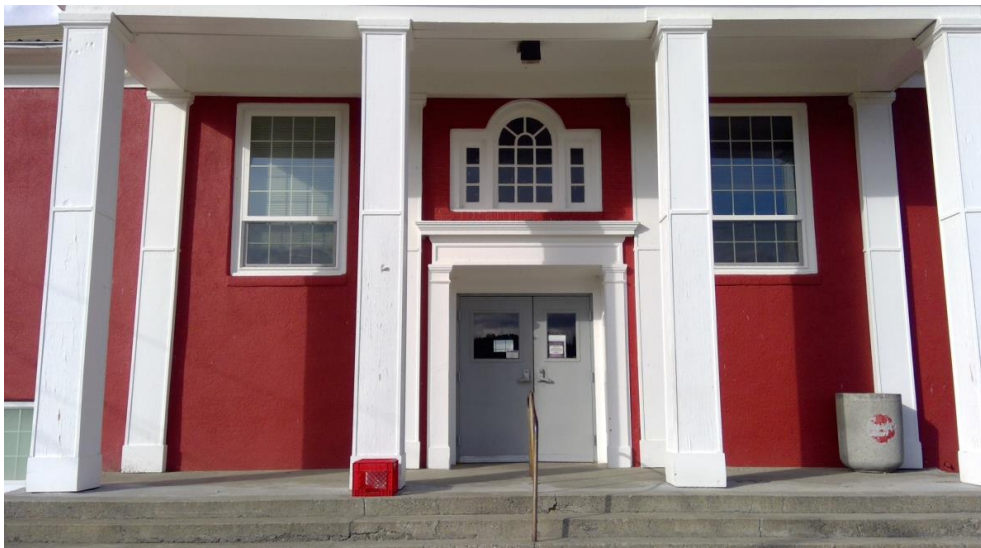
Closeup of Original Schoolhouse Entry
