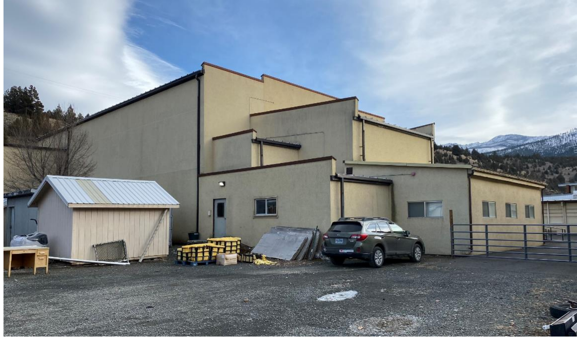
West (rear) Elevation of Original Schoolhouse
