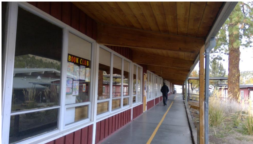
Classroom Wing Exterior Corridor
