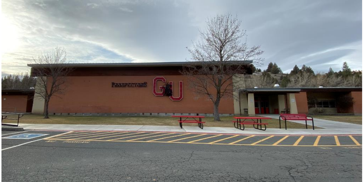
East (front) Elevation of Gymnasium / Classroom Wings
