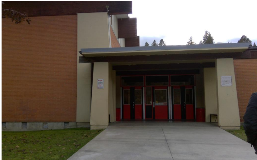
Closeup of Current School Entry (adjacent to gymnasium)
