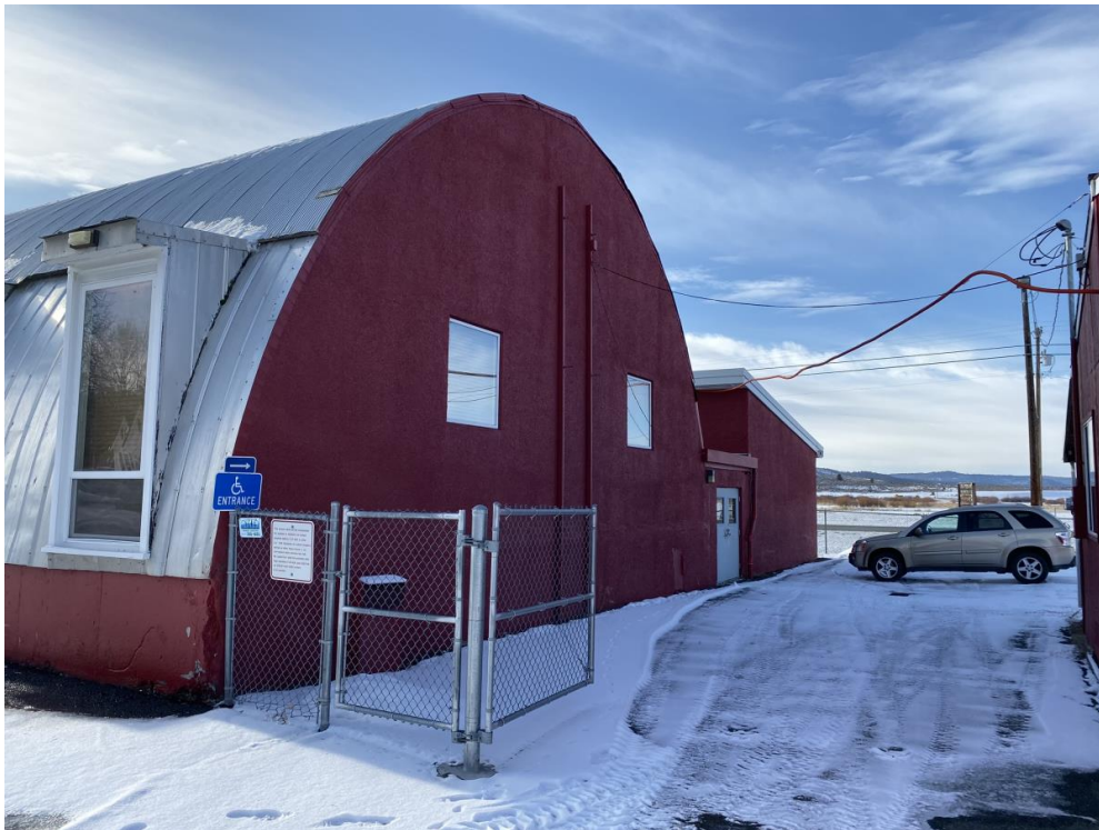
Rear (North Elevation) of Quonset Hut & Classroom Addition
