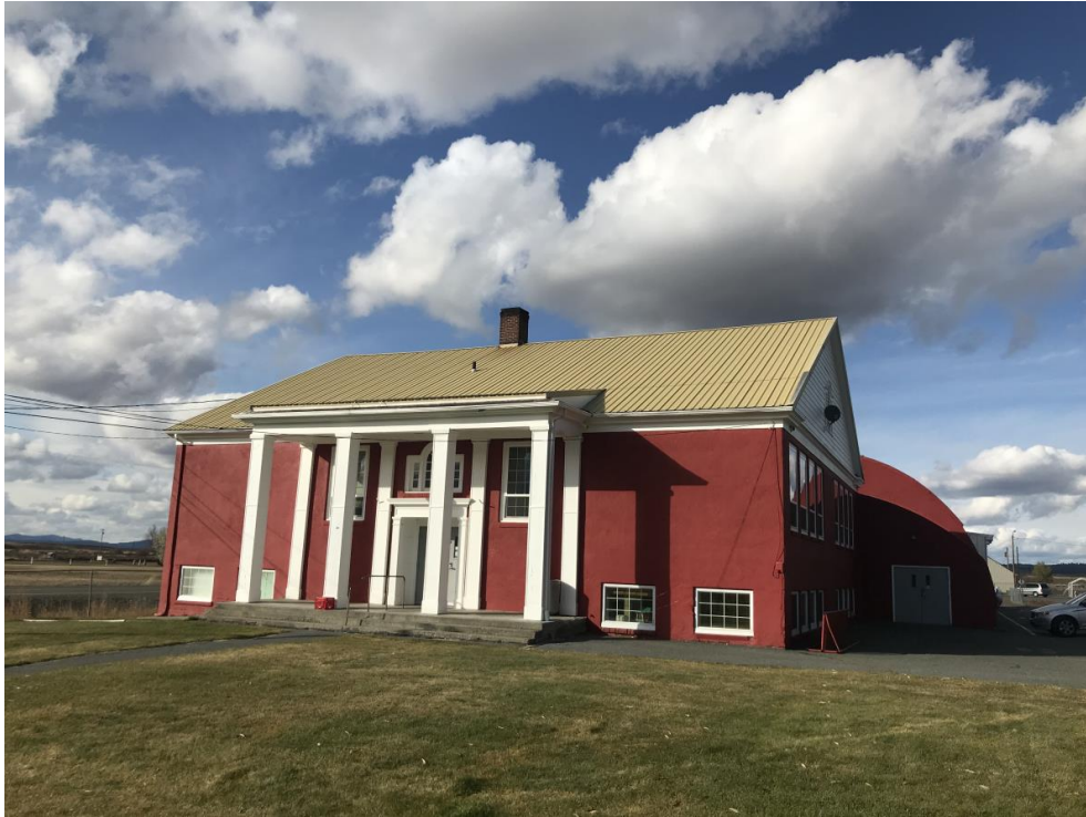
Front (South Elevation) of Original Schoolhouse (with Quonset Hut Gym Addition in Rear)
