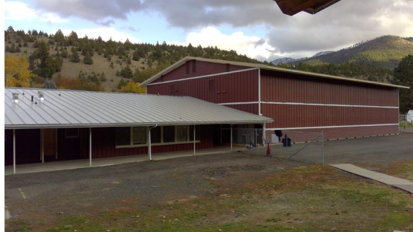
West Elevation of Original Classroom Wing and Gymnasium Addition
