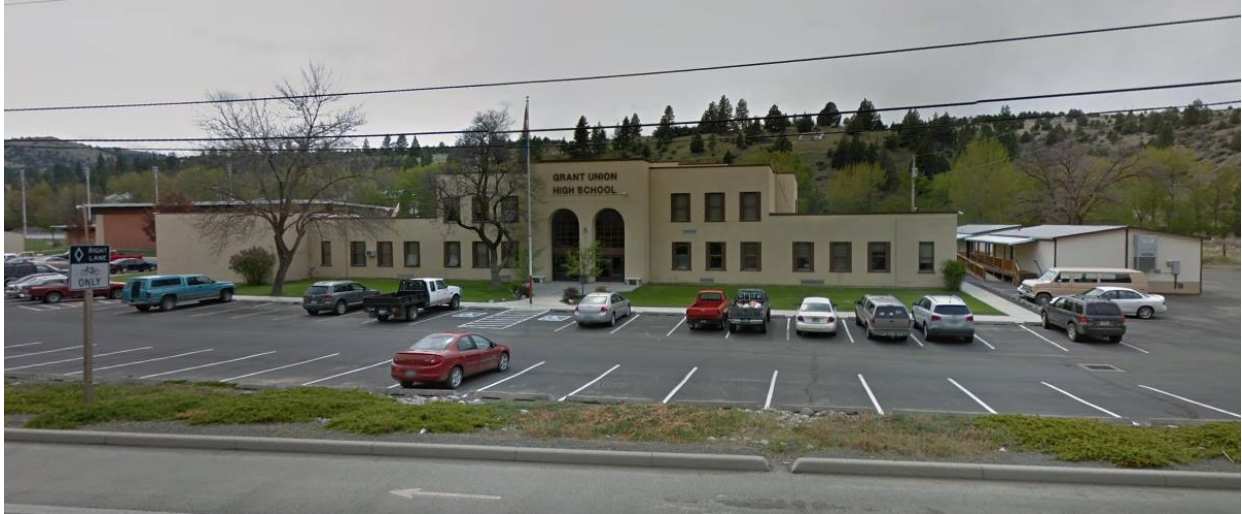
East (front) Elevation of Original Schoolhouse with Office/Library Addition on Left and Portables on Right
