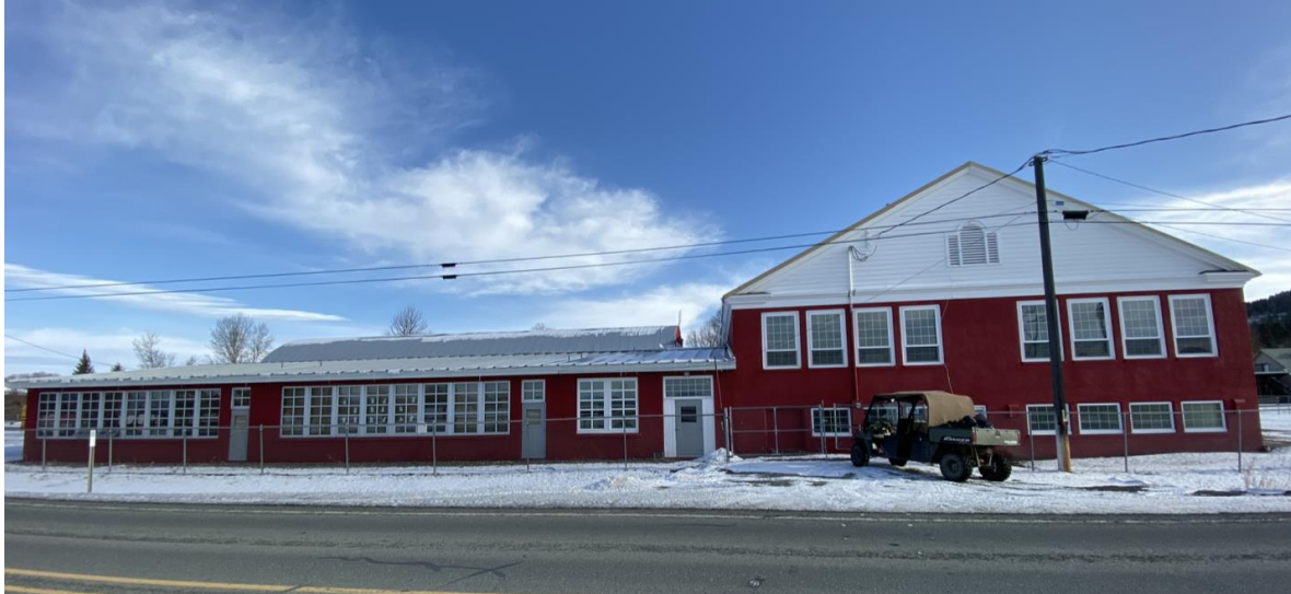
West Elevation of Original Schoolhouse & Classroom Addition
