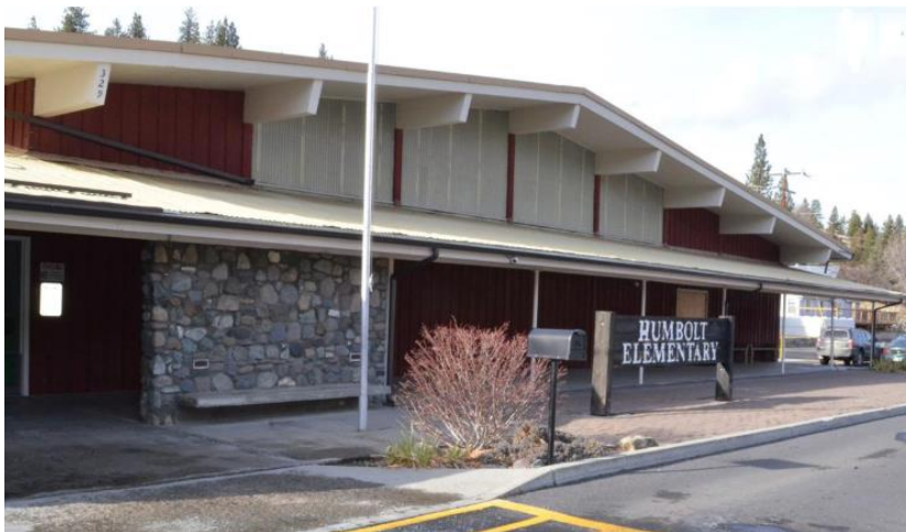
Closeup of Front Entry (East) Elevation of School
