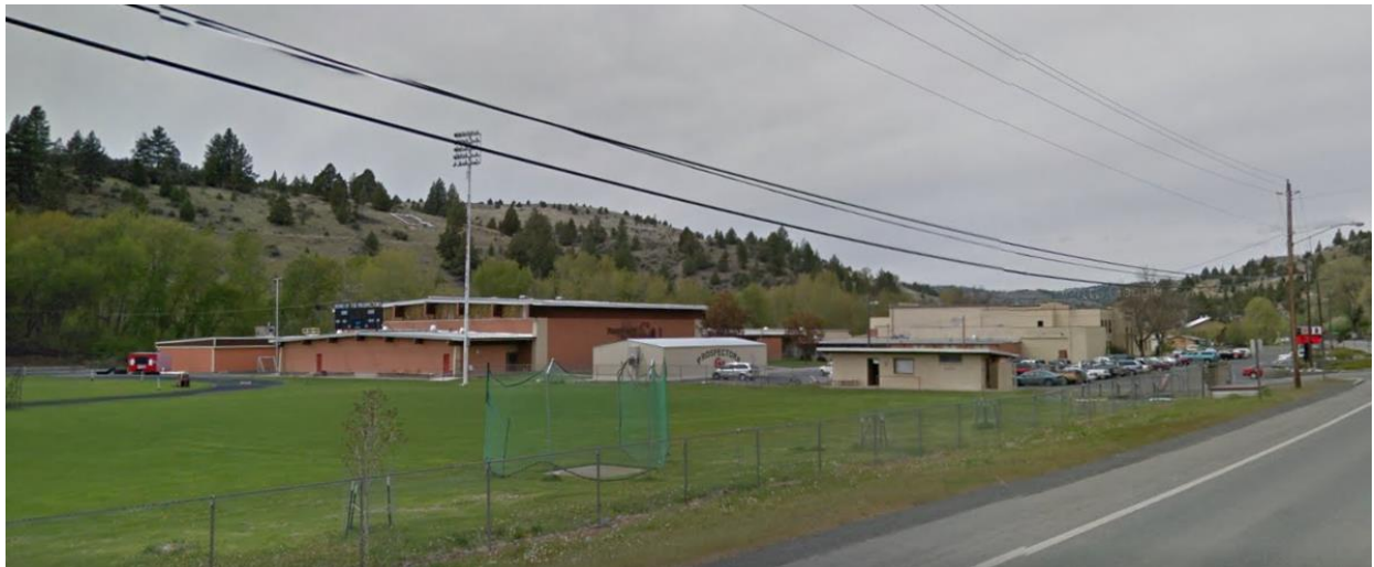
South (side) Elevation of Gymnasium and Classroom Additions, Field House in Foreground Right with Original Schoolhouse in Background
