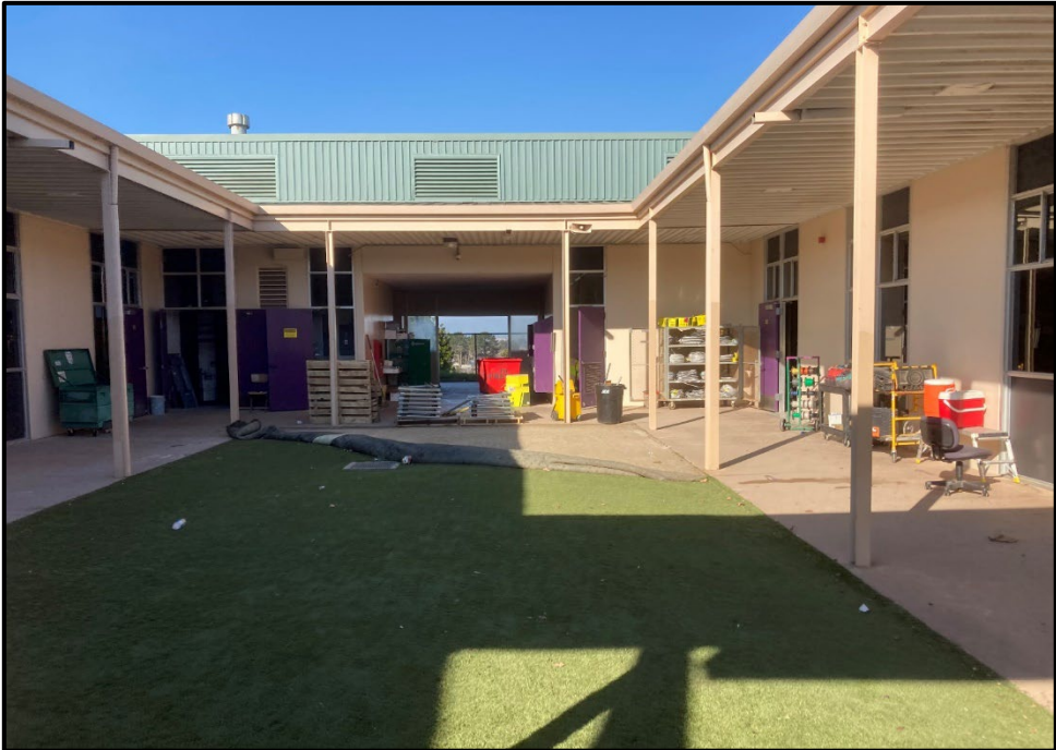
ERHS Modernization Phase II – Exterior Walkways are Used to Store Tools and Equipment
