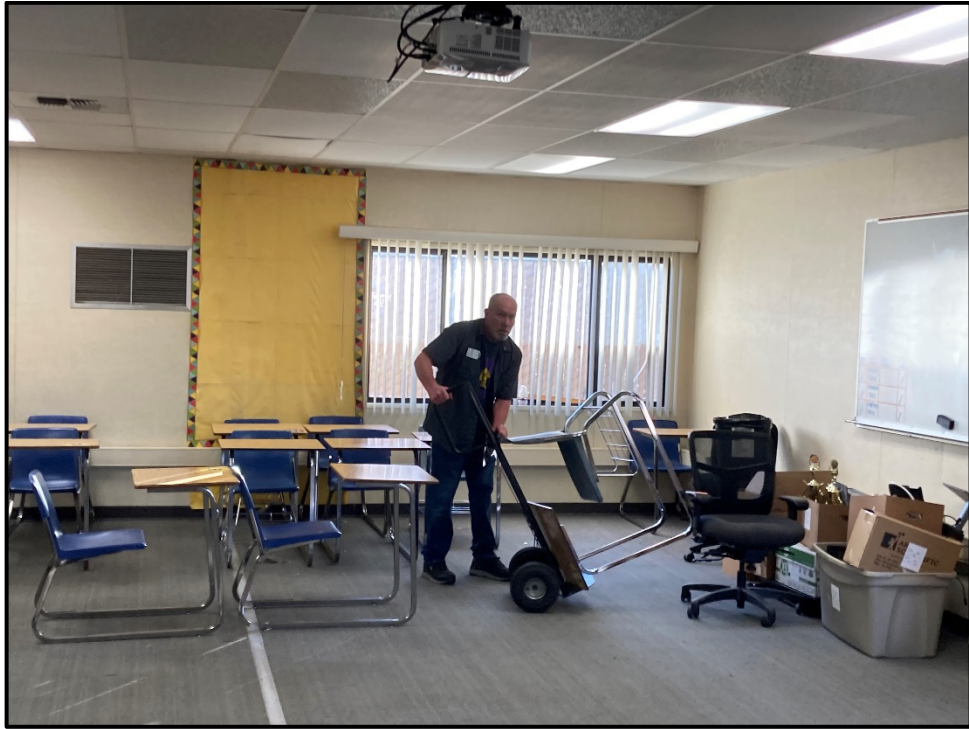
ERHS – Gordon Greer Removing Items for Classroom Renovations
