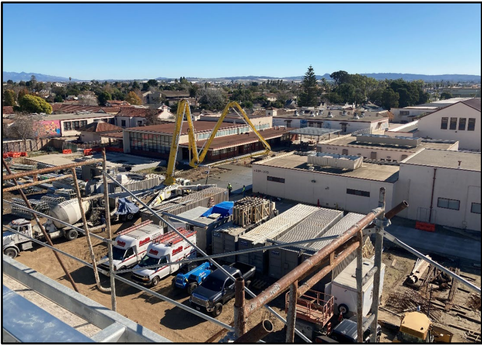
SMHS 50-Classroom Building – Concrete Walkways Poured During Winter Break to Tie the New Building into the Existing Campus
