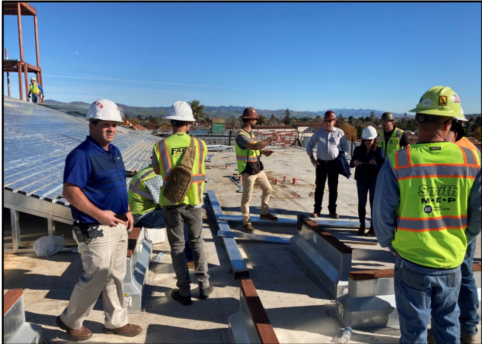
SMHS 50-Classroom Building – Plant Manager Ken Groppetti Participates in the Roofing Pre-Construction Meeting
