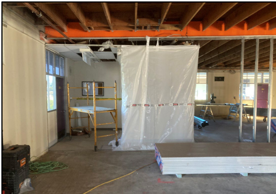
ERHS Modernization Phase II – Abatement of Asbestos Floor Tiles is Underway in Environmental Containment
