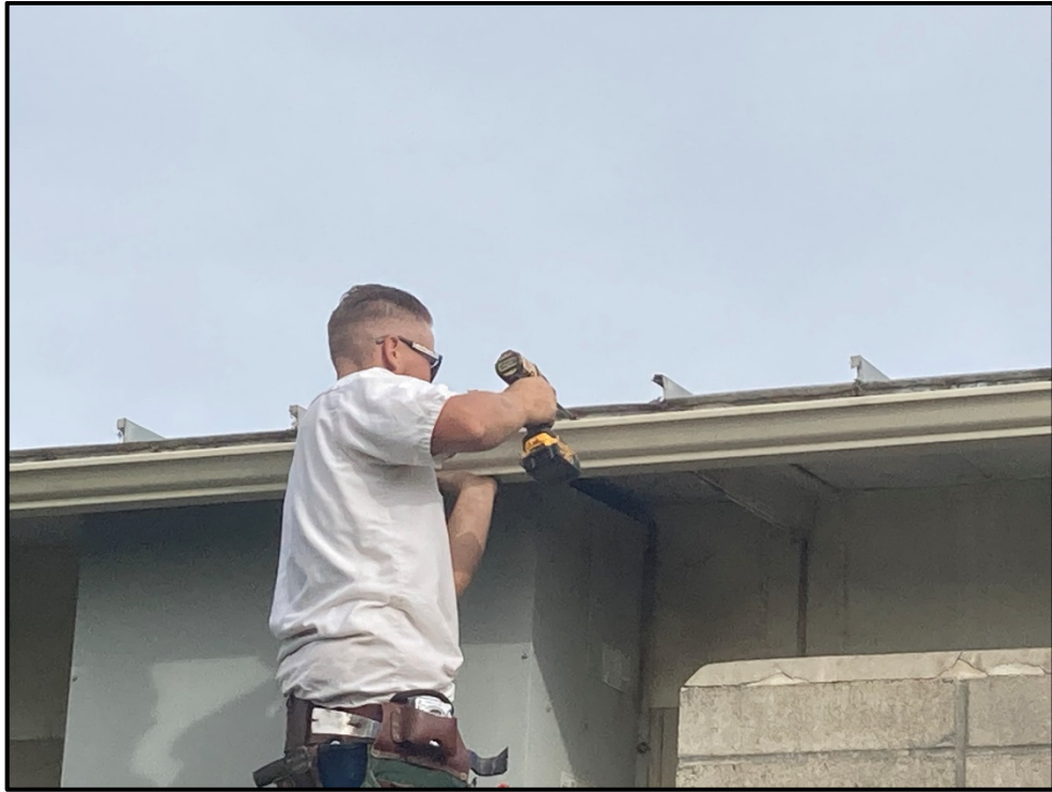
PVHS – Portable Classrooms Receive New Rain Gutters over Winter Break
