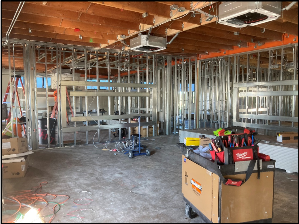
ERHS Modernization Phase II – HVAC Ceiling Distribution Cassettes are Installed in Classrooms
