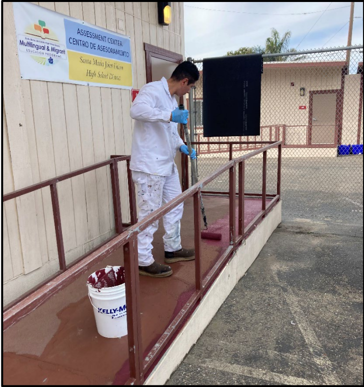
SMHS – Joel Amezcua Resurfacing the Lincoln Center Classroom Ramps
