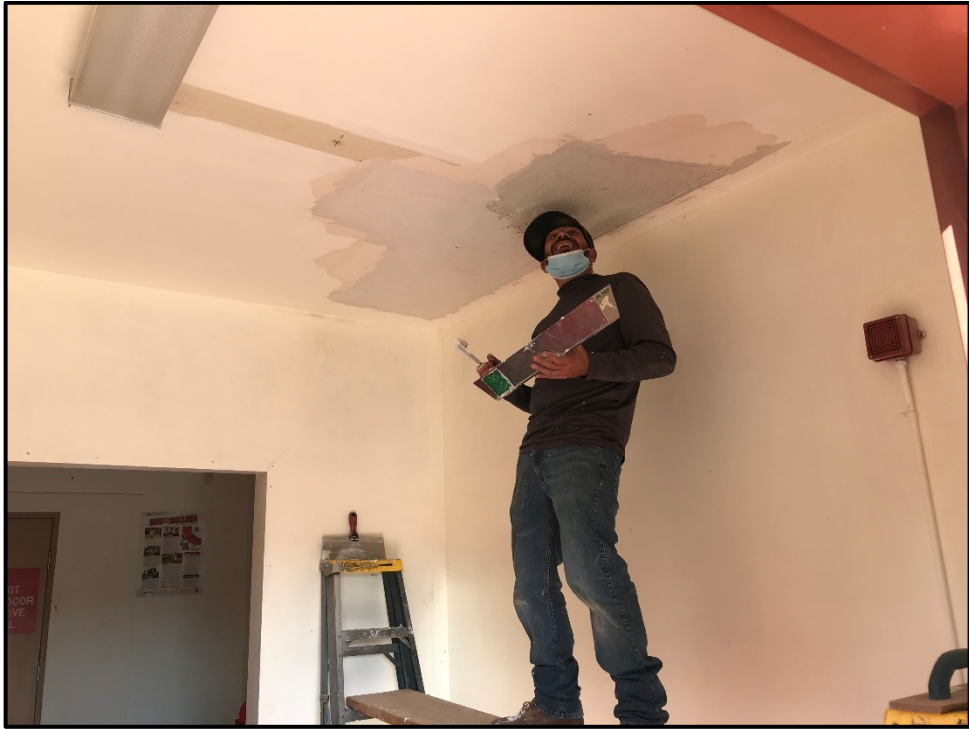
SMHS – Tom Harbold Applies Drywall Compound in the Small Gymnasium
