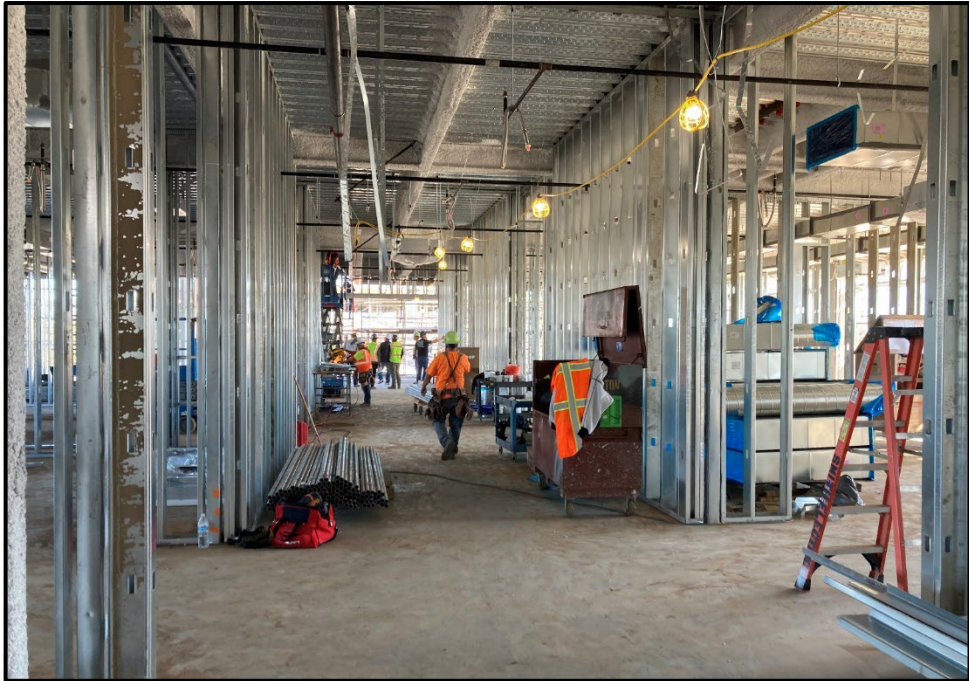
SMHS 50-Classroom Building – Interior Walls and Utilities Installation In-progress
