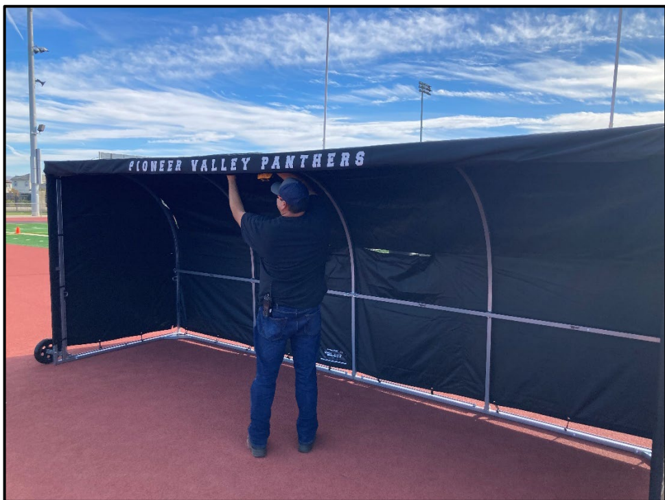
PVHS – Elias Camacho Installs Weather Protection Shells for the Athletic Department
