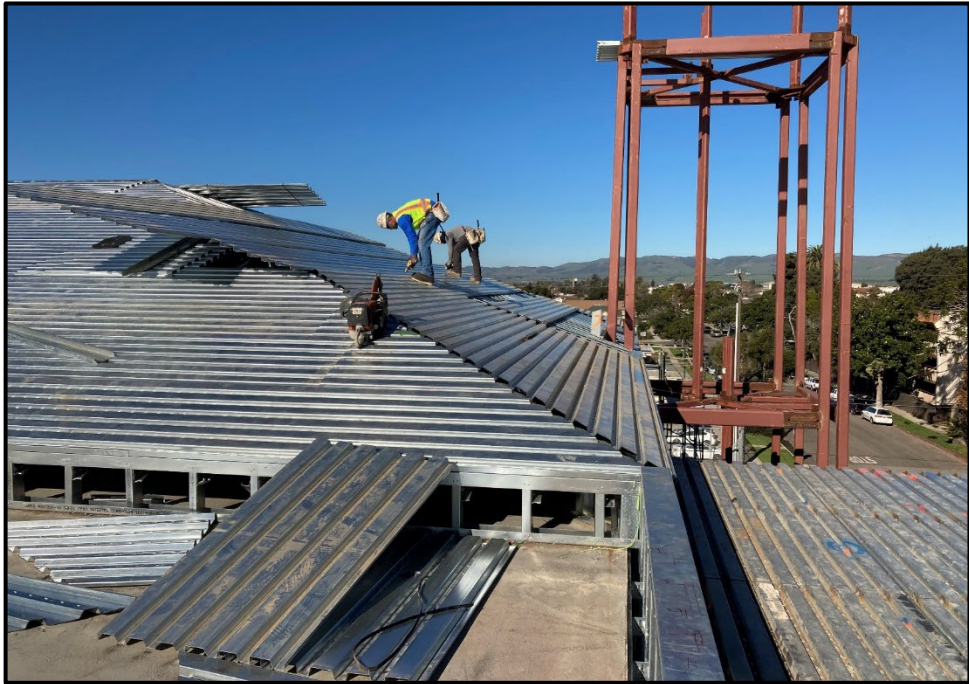
SMHS 50-Classroom Building – Framers Install the Roof Deck for the Tile Roofs
