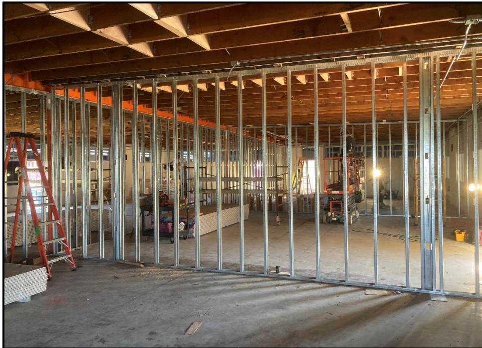
ERHS Modernization Phase II – New Metal Studs are in Place to Define Classrooms and Drywall Installations Begins
