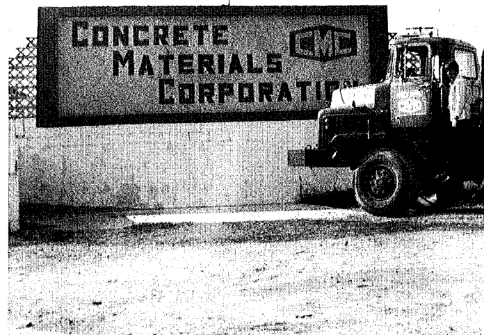
Concrete Materials on N. Scenic Hwy.
