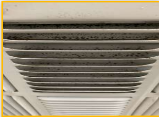
Location: ROOM 3 1.5 Microbial Growth Inside Air Vent
