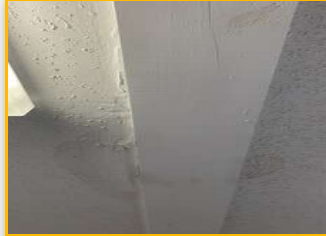
Location: ROOM 8 1.4 Past Water Stains
