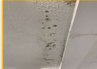
Location: ROOM 6 1.4 Mold Growth/Water Damage
