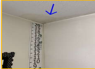
Location: ROOM 1 1.3 Moisture Stain
