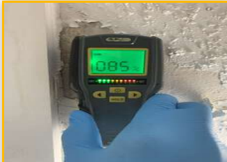
Location: ROOM 6 1.5 Moisture Detected/Ceiling
