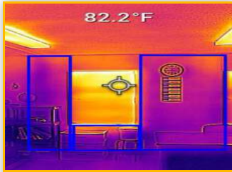
Location: ROOM 3 1.7 Moisture Detected in Wall/Infrared
