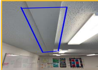
Location: ROOM 6 1.6 Moisture Detected/Ceiling
