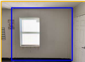
Location: ROOM 3 1.2 Moisture Detected in Wall
