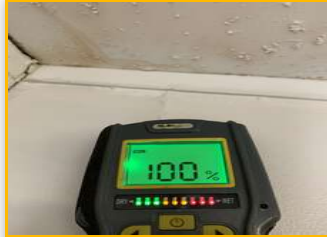
Location: ROOM 1 1.4 Moisture Stain/100% Moisture
