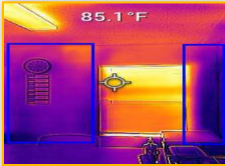
Location: ROOM 3 1.6 Moisture Detected in Wall/Infrared
