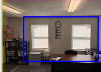
Location: ROOM 3 1.4 Moisture Detected in Wall
