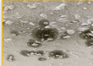
Location: ROOM 6 1.3 Mold Growth
