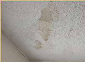
Location: ROOM 8 1.5 Past Water Stains
