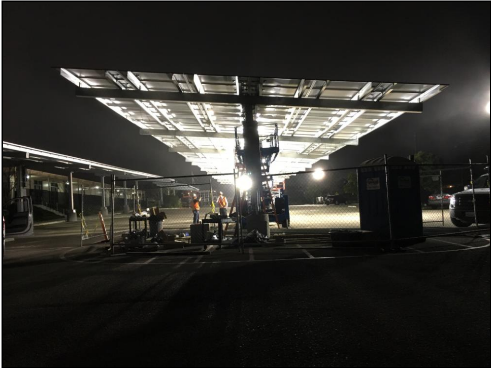
ERHS – After Hours Work Begins to Finish the Solar Installation Without Affecting Parking
