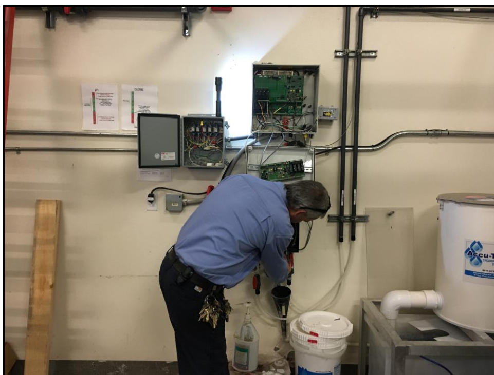
ERHS – Del Ward Repairs the Power Supply for the Pool Controller
