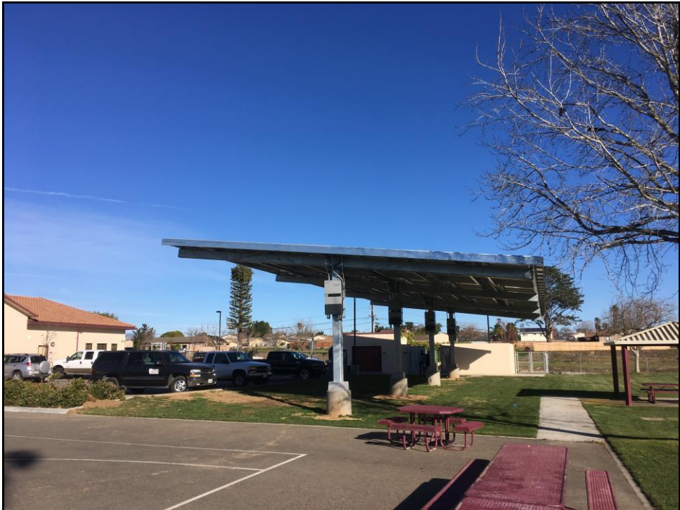
DHS Solar Power – Structure and Panels in Place: Awaiting Final Connection to Power Grid
