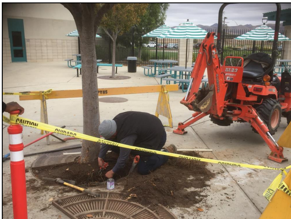
PVHS – Alan Rodriguez Repairs a Broken Sprinkler Line Near the Cafeteria
