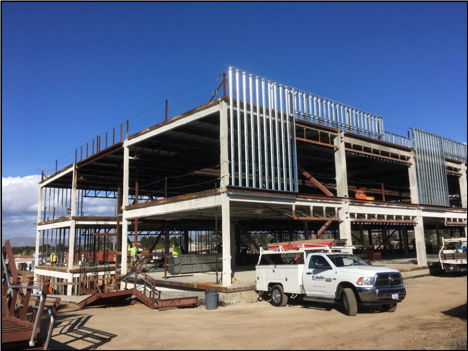
ERHS 38 Classroom Building – Exterior Wall Framing and Plumbing are Underway
