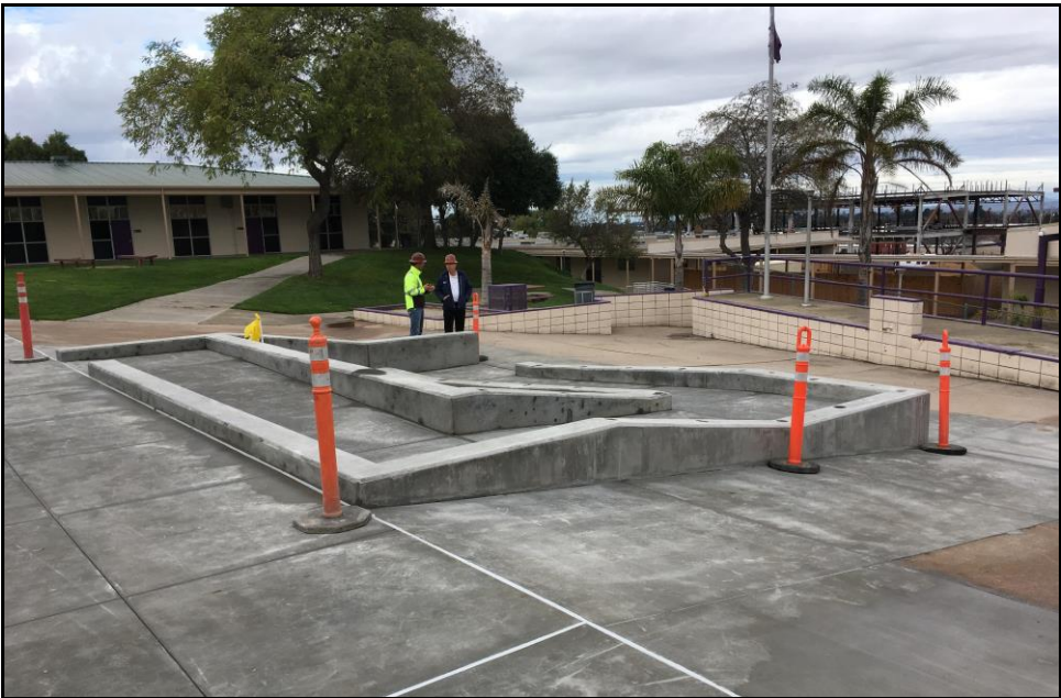
ERHS Student Quad – Replacement Concrete is in Place and ADA ramp is Poured
