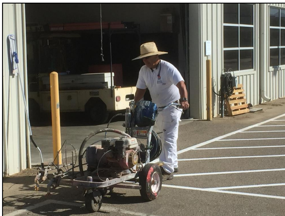
PVHS – Ray Segovia Stripes the Maintenance Access Apron
