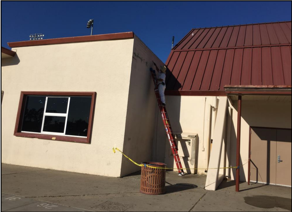
SMHS – Ray Segovia Repaints the Wilson Gymnasium Exterior
