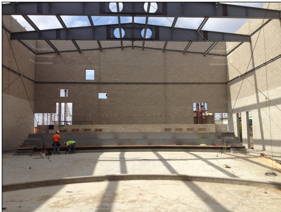
PVHS – Theater Interior as Roof Beams are Placed
