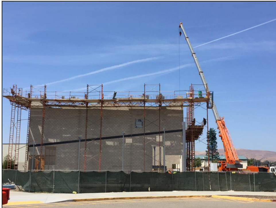
PVHS – A Crane Hoists Roof Beams for the Theater
