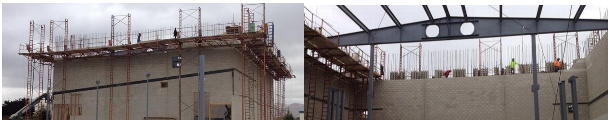
The new District Performing Arts Center under construction, as viewed from the exterior (left) and interior (right)
