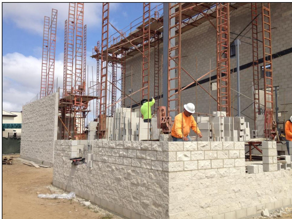
PVHS – Performing Arts Center Lobby Walls Begin to Take Shape
