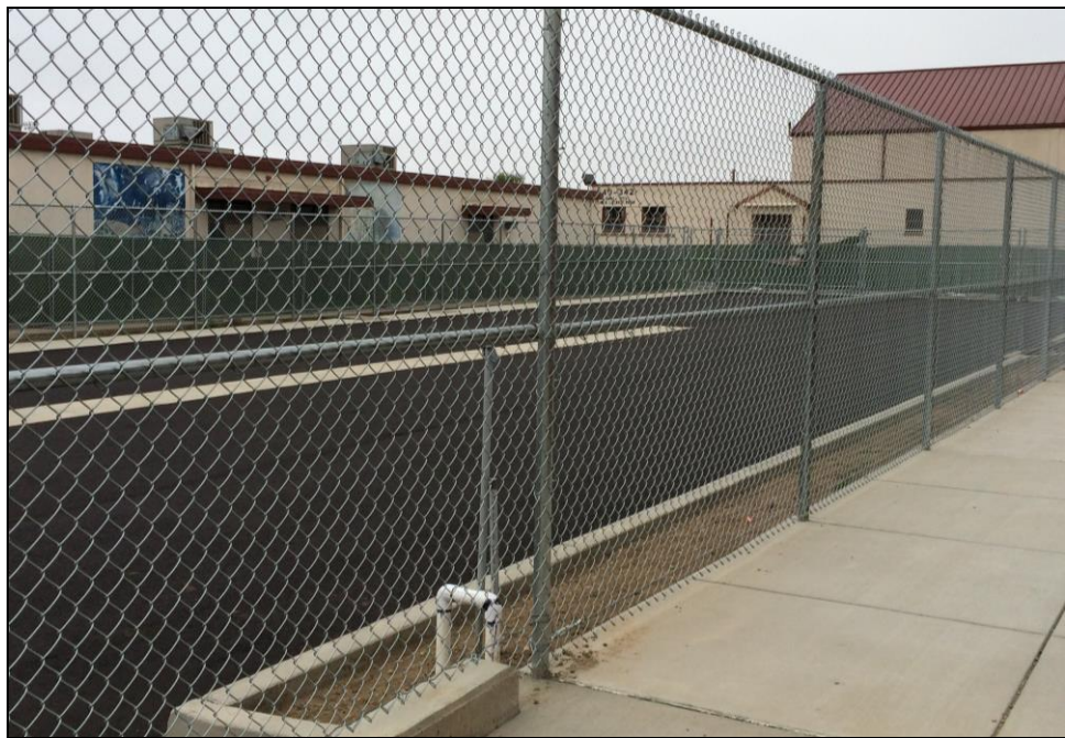
SMHS – Reconfigured Camino Colegio Parking Lot is Paved
