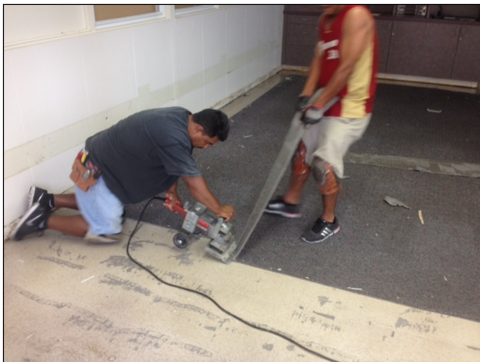
ERHS - Removing Carpet for Textbook Storage Unit Installation
