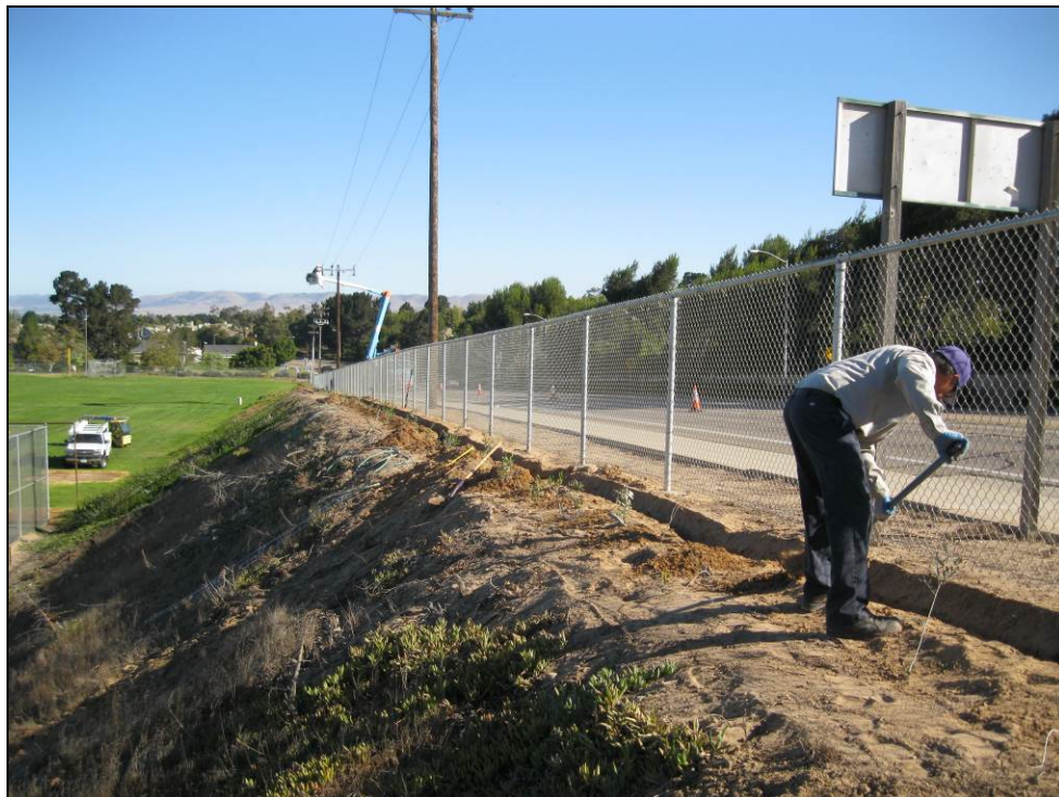
ERHS - Irrigation Installation above the Softball Field
