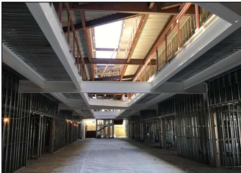
ERHS 38-Classroom Building – Metal Stud Walls Take Shape and Painting Begins
