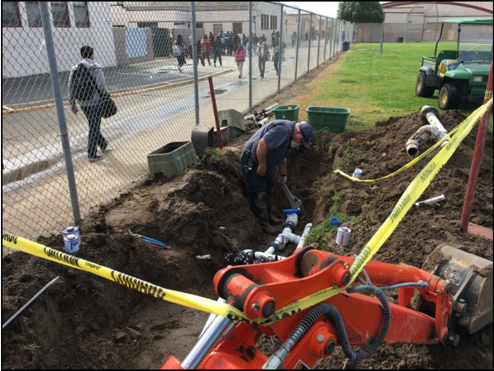
SMHS – Greg Matthews Replaces Three Irrigation Valves in the Softball Field
