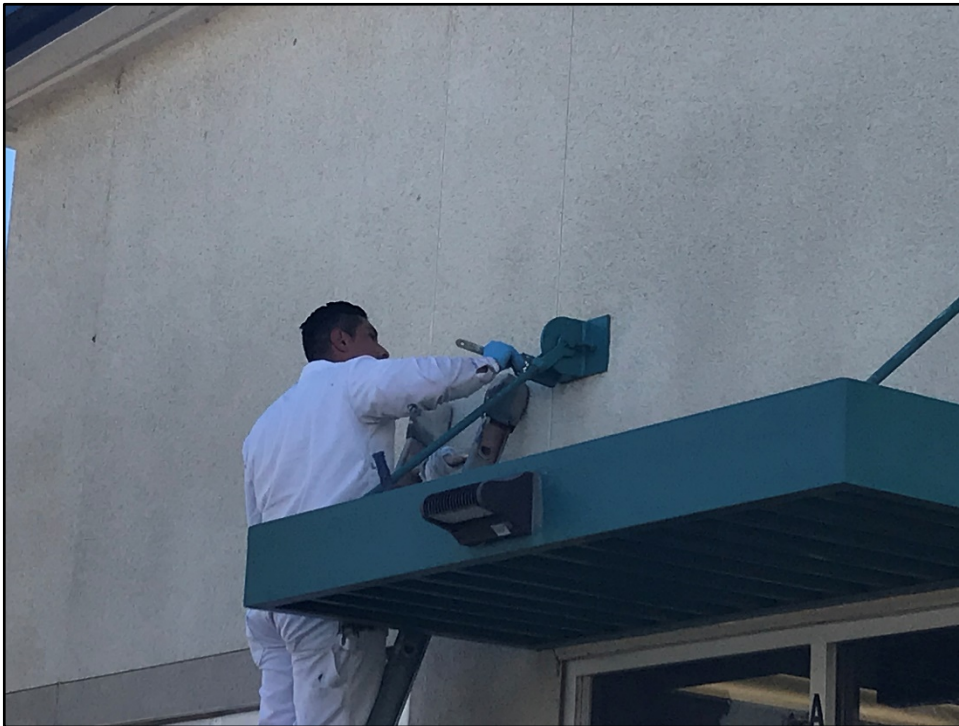
PVHS - Joel Amezcua Repaints Exterior Doors and Awnings
