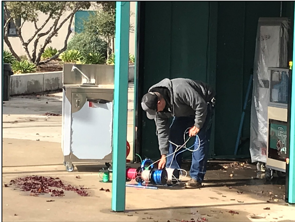
PVHS - Andy Freitas Pulling Wire for the Quick Café Food Service Station
