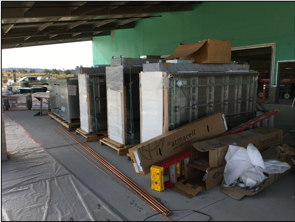
CTE Ag Center - Kitchen Equipment is Staged outside the Culinary Arts Center
