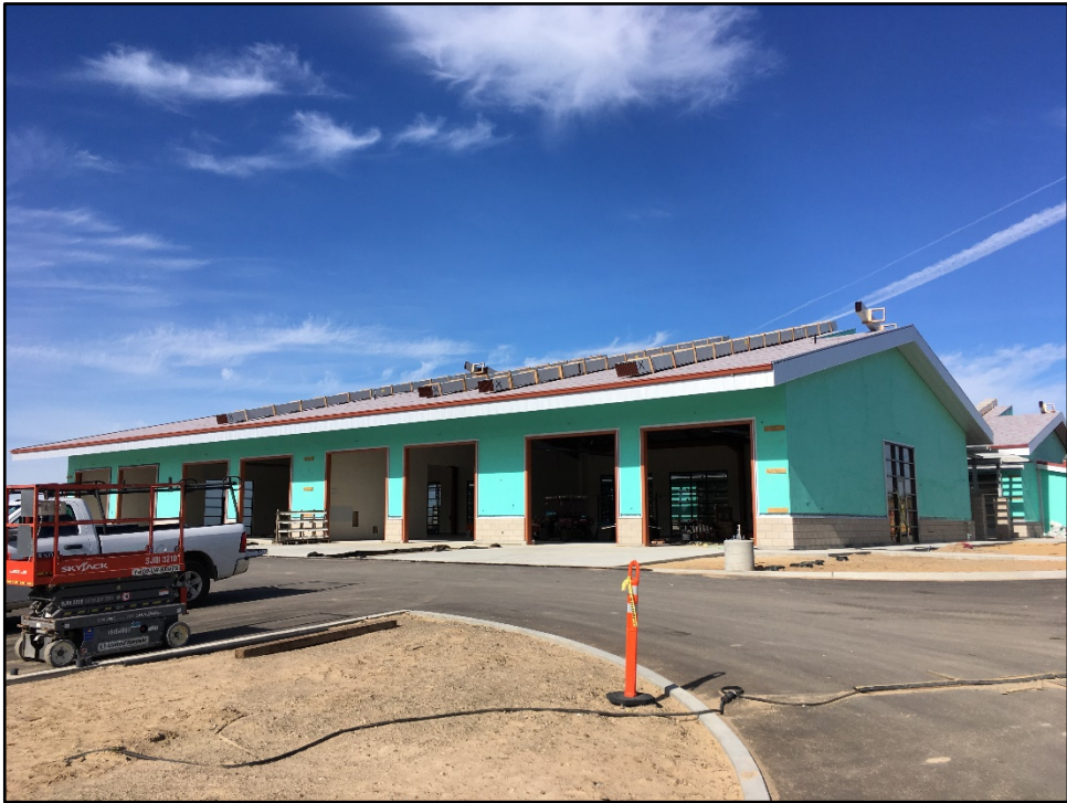
CTE Ag Center - Metal Roofing is Staged on the Roof Awaiting DSA approval of Attachment
