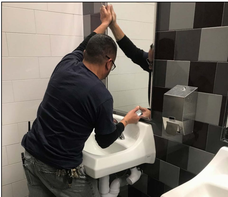
ERHS – Jimmy Salutan Replaces Damaged Mirrors in the New Building Restrooms
