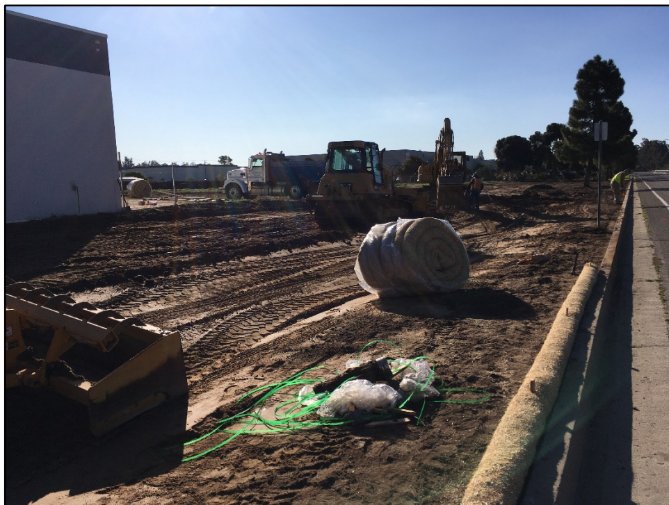
SSC West Parking – Excavation and Storm Water Pollution Prevention are Underway
