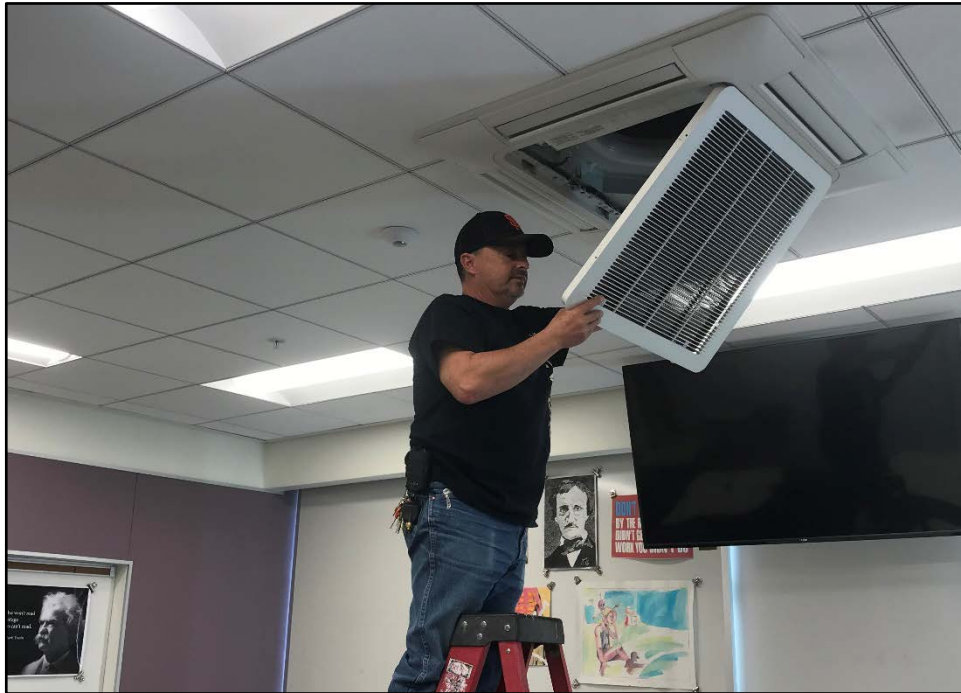
ERHS - Bernie Rayner Cleans the Air Filters in the New Classroom Building
