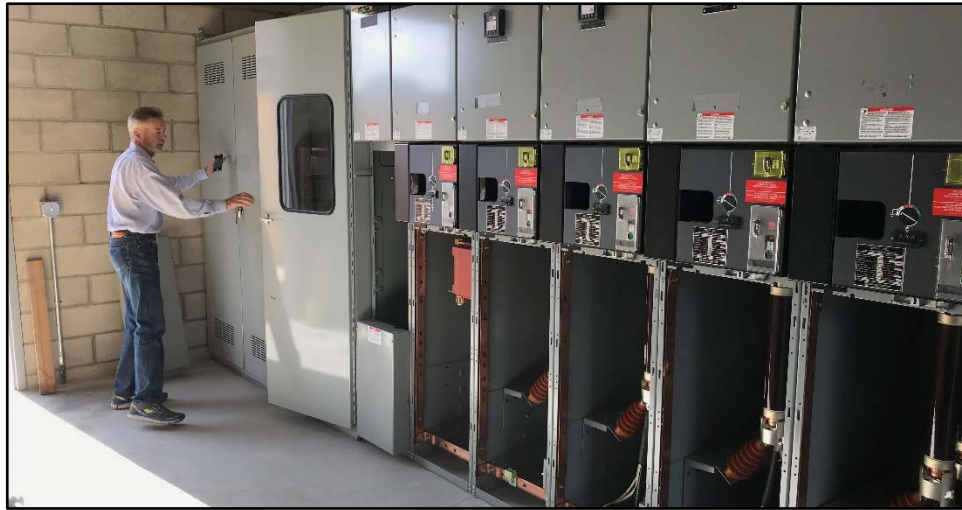
SMHS Reconstruction - Energy Manager Marc Brogotti Inspects the New Switchgear in the Powerhouse
