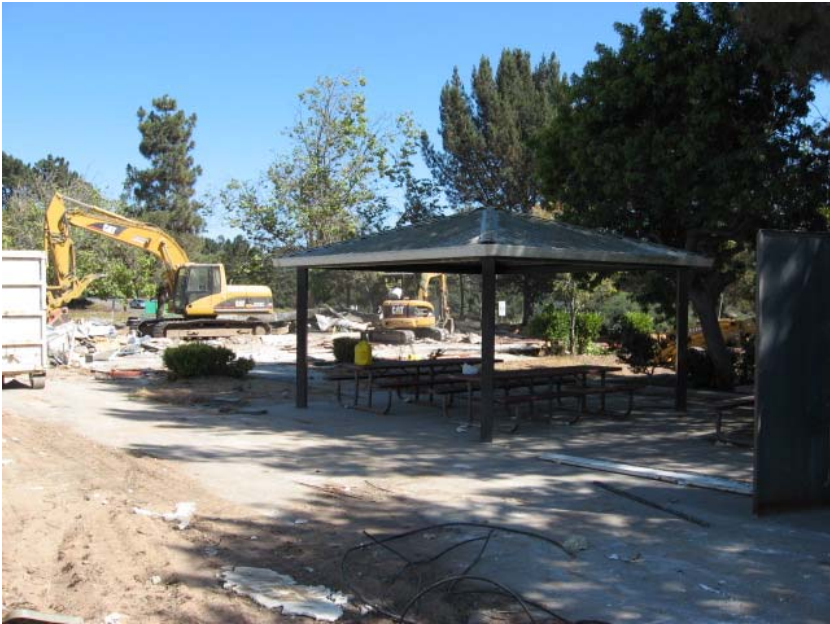
Delta High School Demolition
