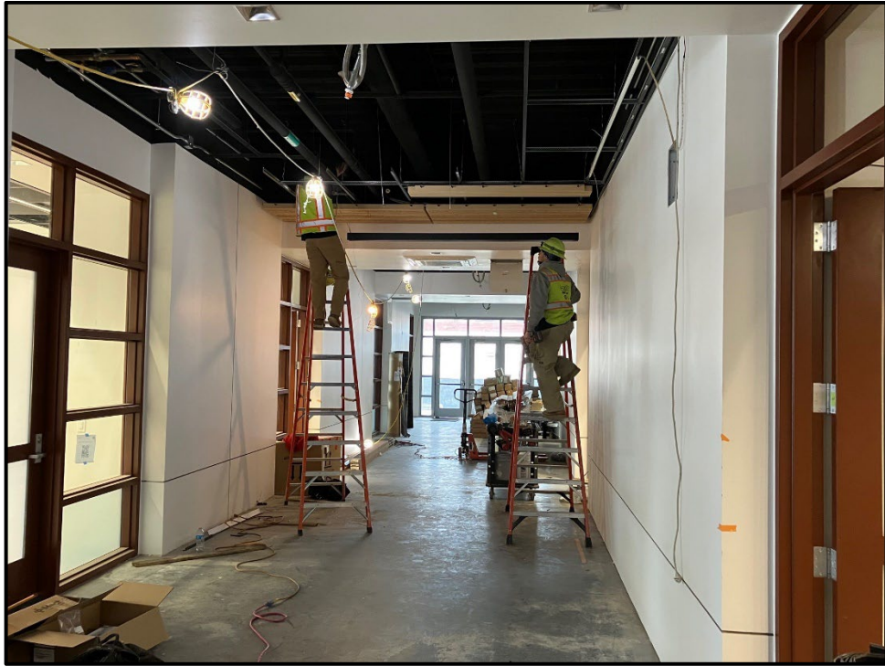
SMHS 50-Classroom Building – Hallway Lighting Installation Is In-progress
