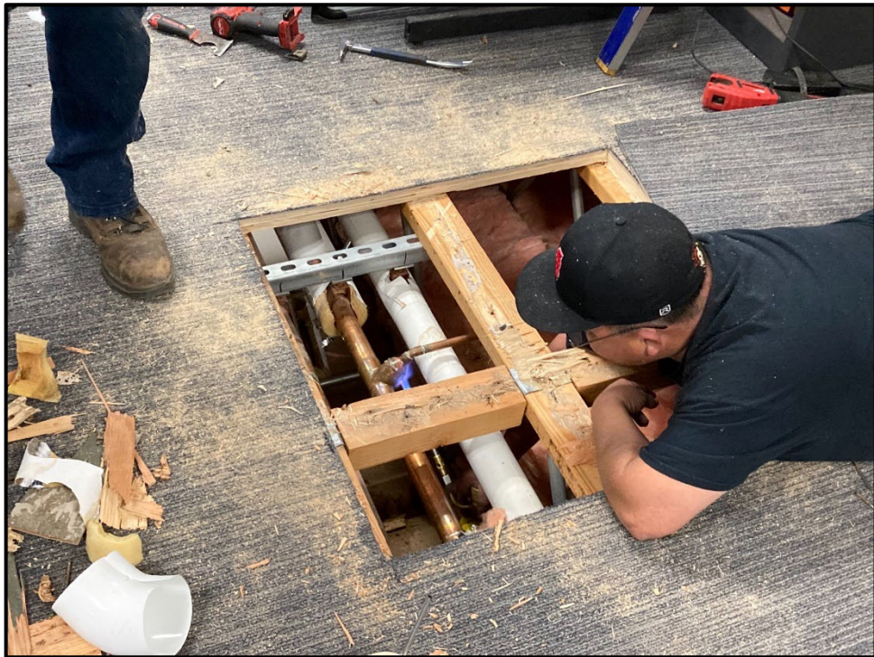
PVHS – Jesus Reyes Repairs a Leak in the 300 Building
