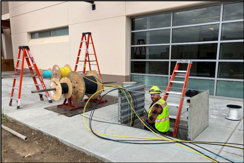
SMHS 50-Classroom Building – Telephone and Fiber Optic Cables are Installed
