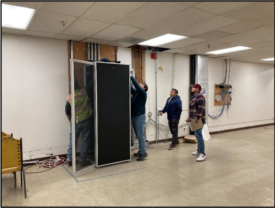
SSC Second Story Reconfiguration – Relocating Existing Technology Cabinet
