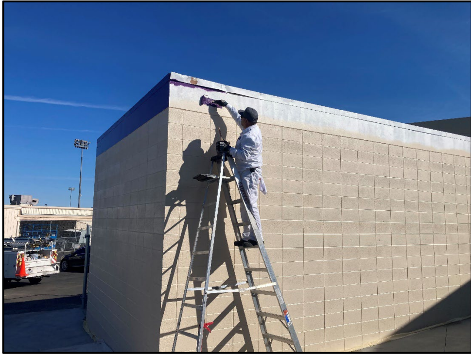
ERHS – Ernest Paz Paints the Block Wall of the Power House
