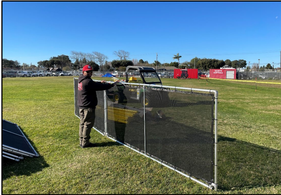
SMHS – Nelson Frutos Installs the New Softball Outfield Fencing
