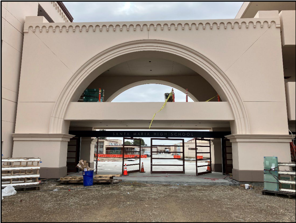
SMHS 50-Classroom Building – The New Entrance to the School is Taking Shape
