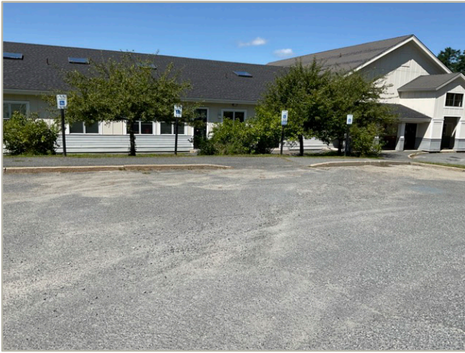
1 - OVERVIEW OF ACCESSIBLE PARKING AREA
