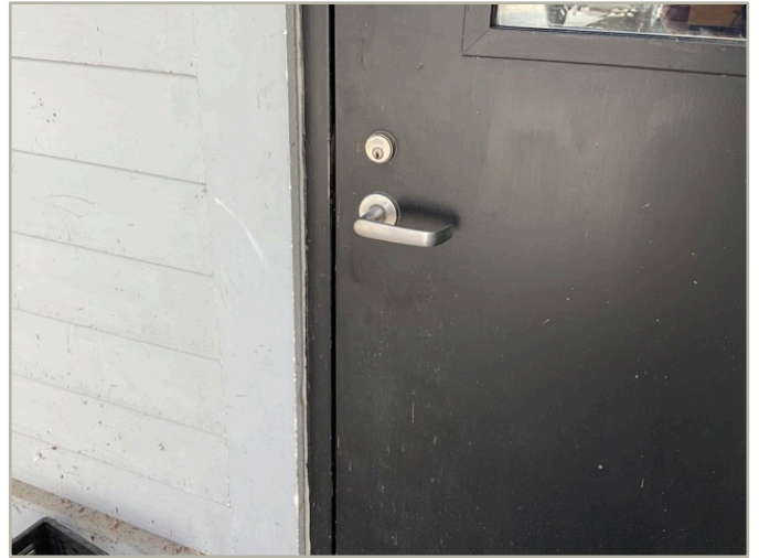
8 - INTERIOR PATH DOOR HARDWARE
