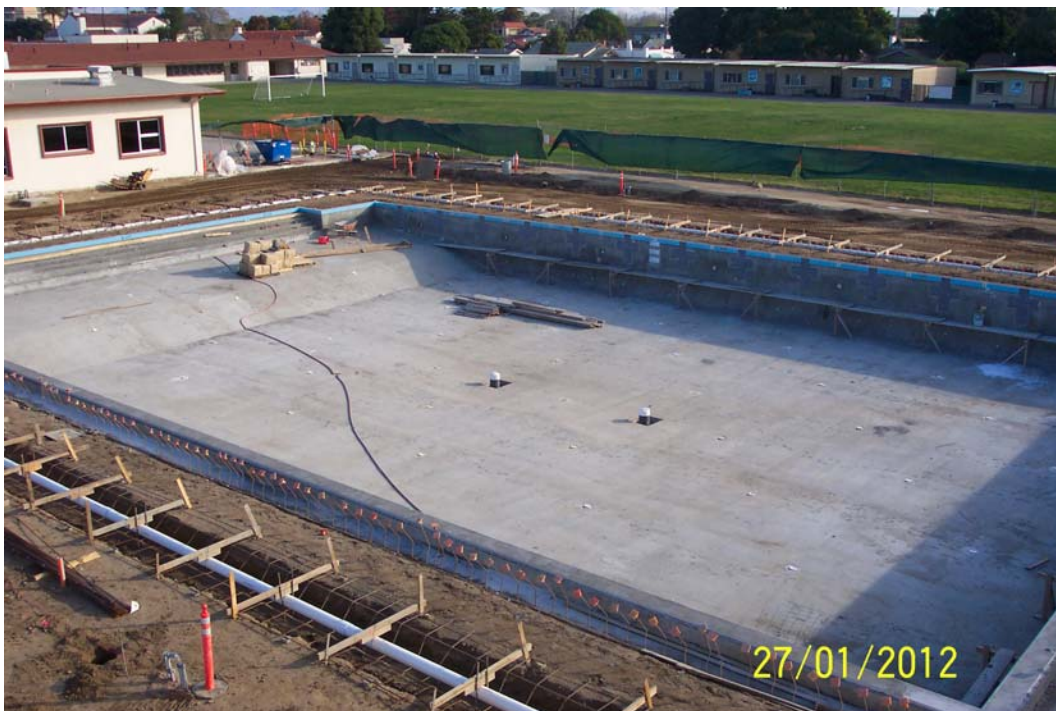
SMHS Pool Under-Deck Pipe Ready For Concrete
