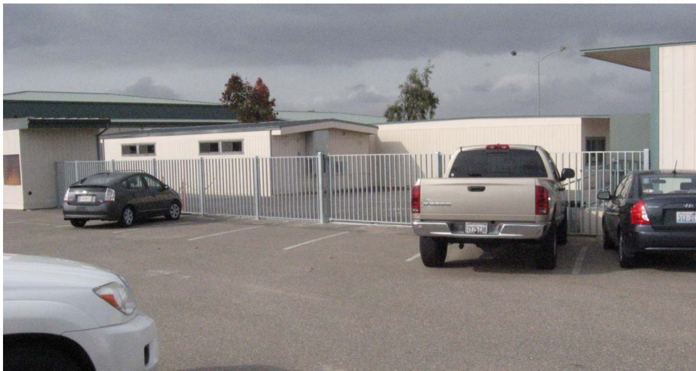
ERHS East Parking Receives a New and Improved Fence
