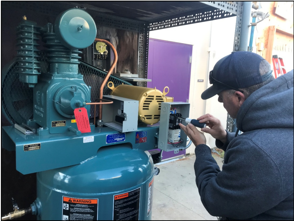
ERHS - Andy Freitas Wires the New Compressor for Industrial Arts
