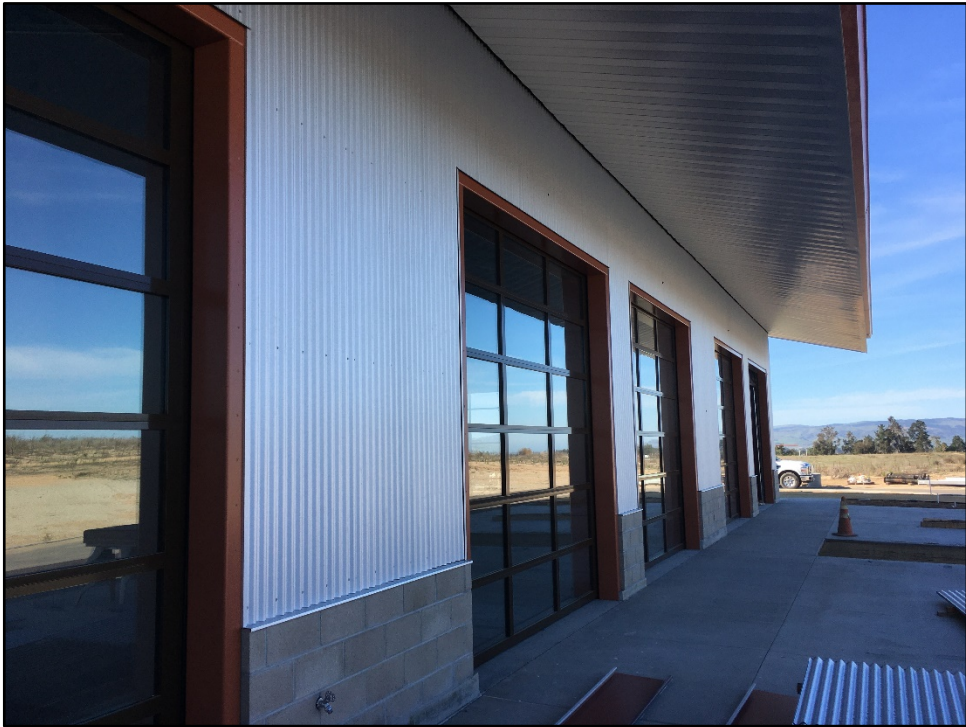
CTE Ag Center – Shop Classrooms Receive Metal Siding and Roll-up Doors
