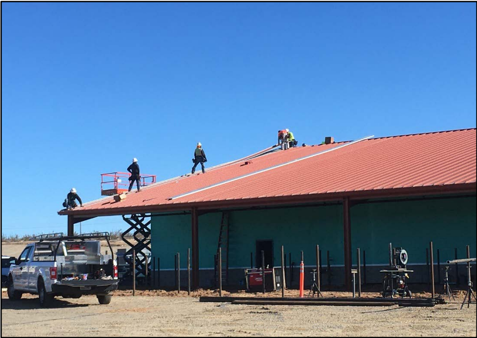
CTE Ag Center – Roof Decking is Placed on the Culinary Arts Building
