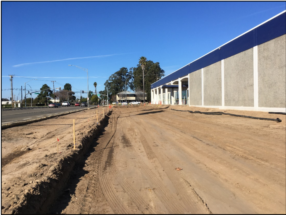
SSC West Parking – Parking Lot is Starting to Show General Dimensions
