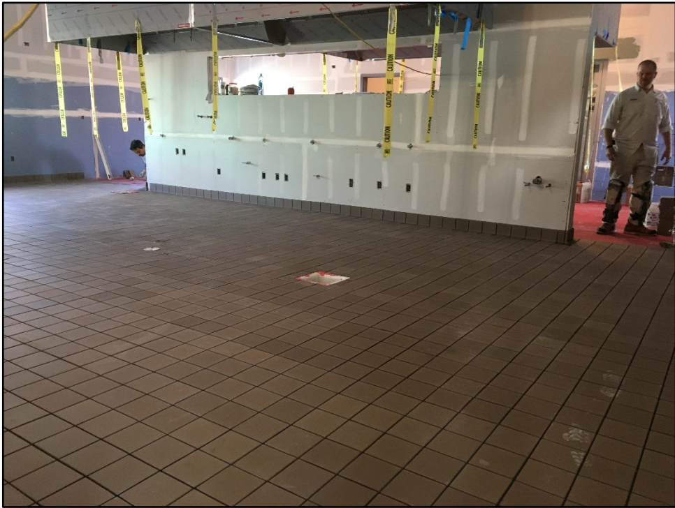
CTE Ag Center - Kitchen Floor Tile Installation is Underway
