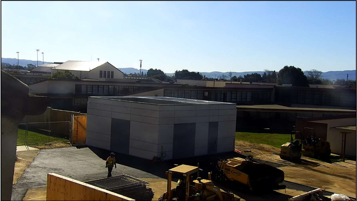
SMHS Reconstruction – Asphalt Paving is Placed Around The New Powerhouse
