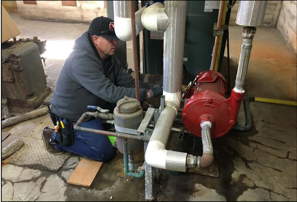
SMHS – Andy Freitas Rewires the New Boiler Circulating Pump Motor
