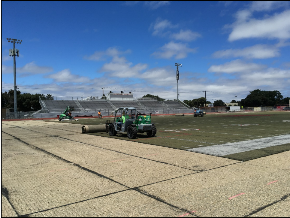
SMHS Synthetic Turf – Existing Turf is Rolled and Removed
