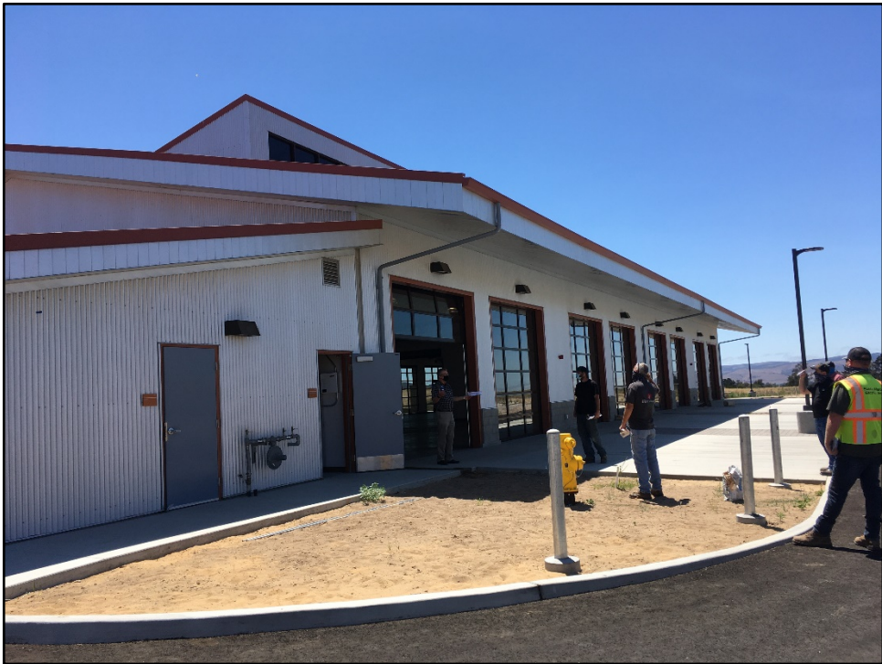
CTE / Ag Center – District and Contractors Review Security Camera Locations
