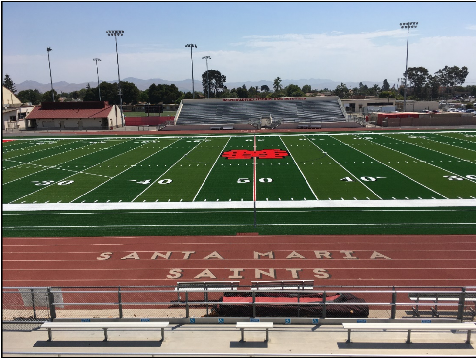
SMHS Synthetic Turf – Completed Installation Transforms the Stadium
