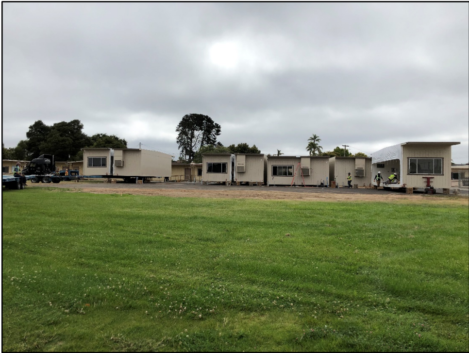
SMHS Eight Portable Classrooms – Building Halves are Aligned and Assembled
