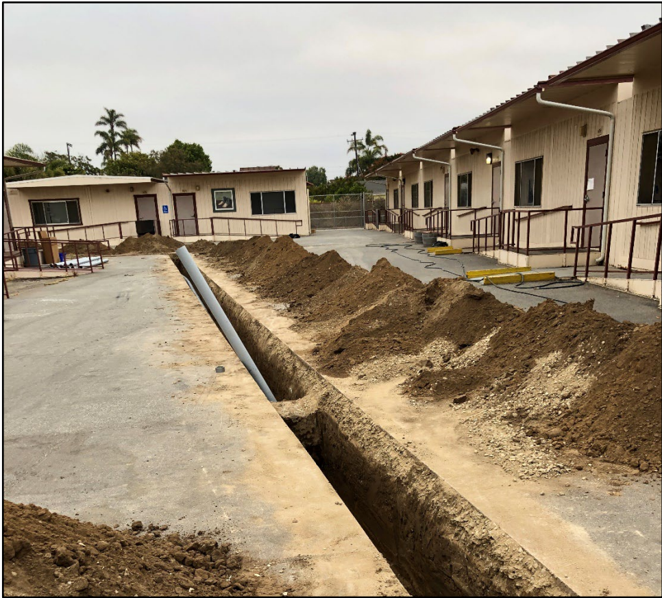
SMHS Eight Portable Classrooms – Conduit for Power and Communications Ties into Existing Switchgear
