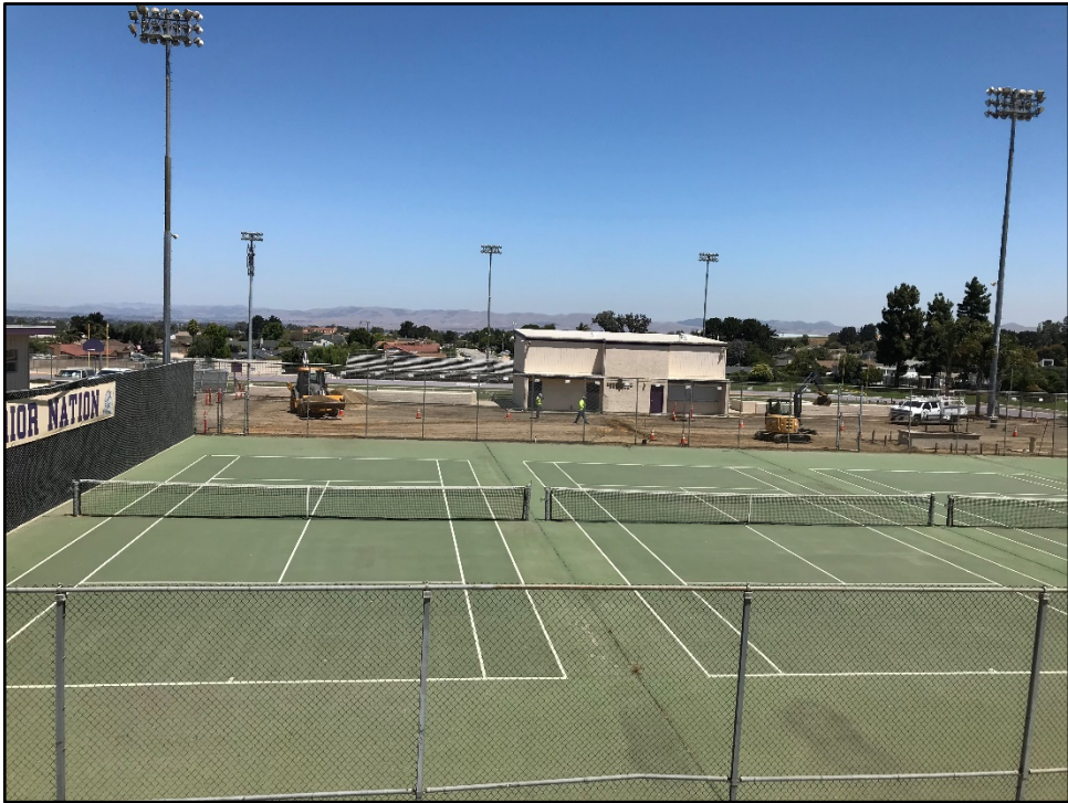
ERHS 2020 Paving – Excavation Begins to Remove Old Asphalt
