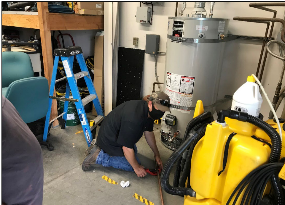
PVHS – Erik Fulton Replaces the Water Heater in the Maintenance Shop
