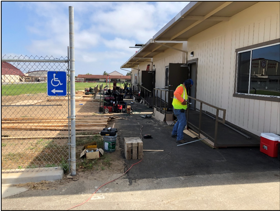
SMHS Eight Portable Classrooms – Ramps and Wooden Foundations are Installed
