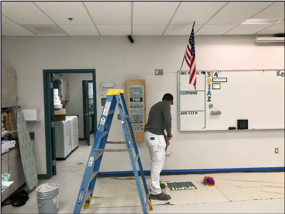
PVHS – Joel Amezcua Refreshes Classroom Interiors
