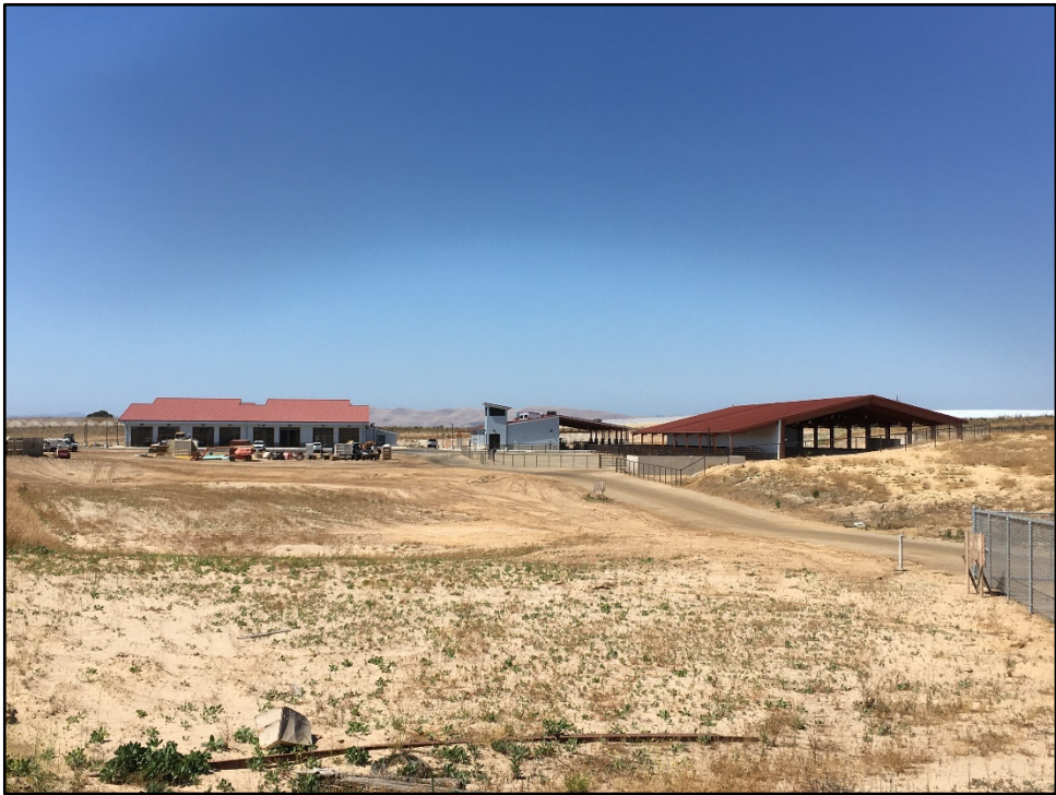
CTE / Ag Center – Overall View as the Project Nears Completion
