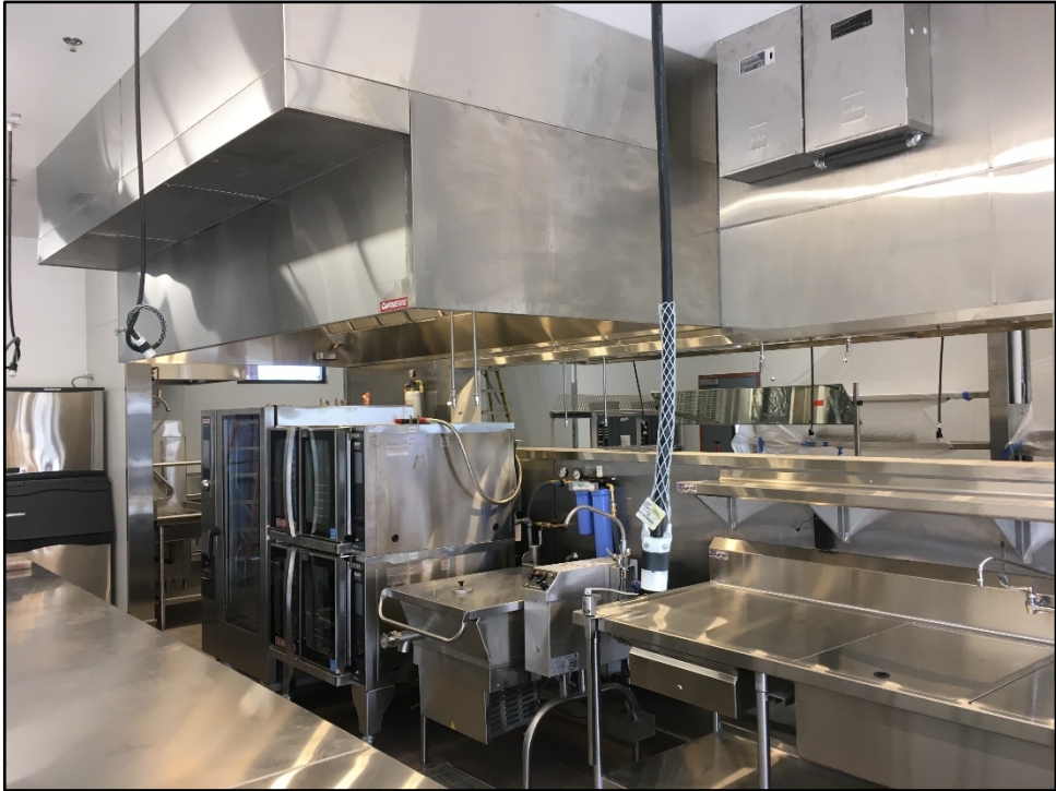
CTE / Ag Center – Culinary Arts Kitchen is Complete and Ready to Go!
