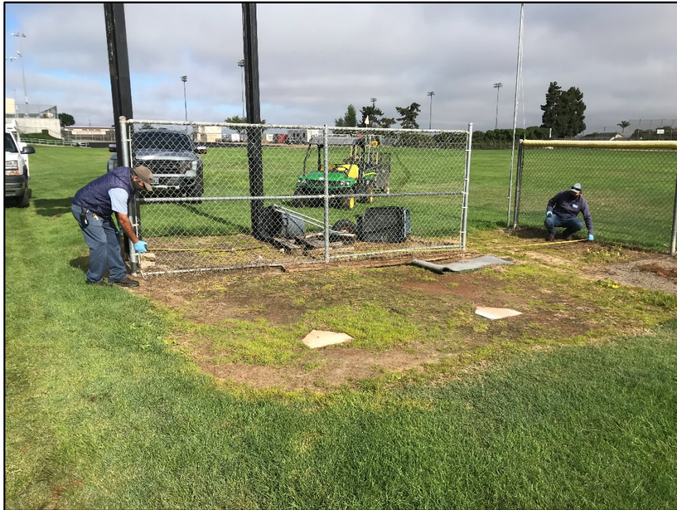
ERHS – Juan Rodriguez and Joseph Campos Begin Renovation of the Softball Bullpens
