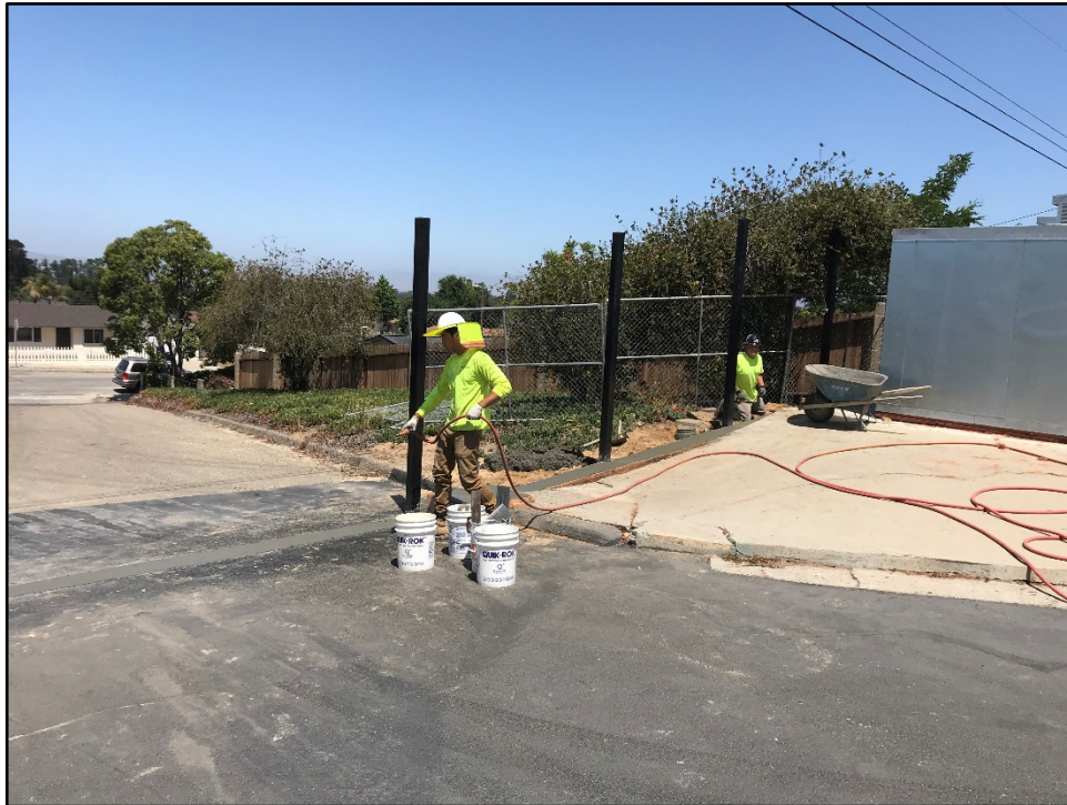
ERHS – Automatic Gates and Remote Controllers are Installed to Provide Emergency Access
