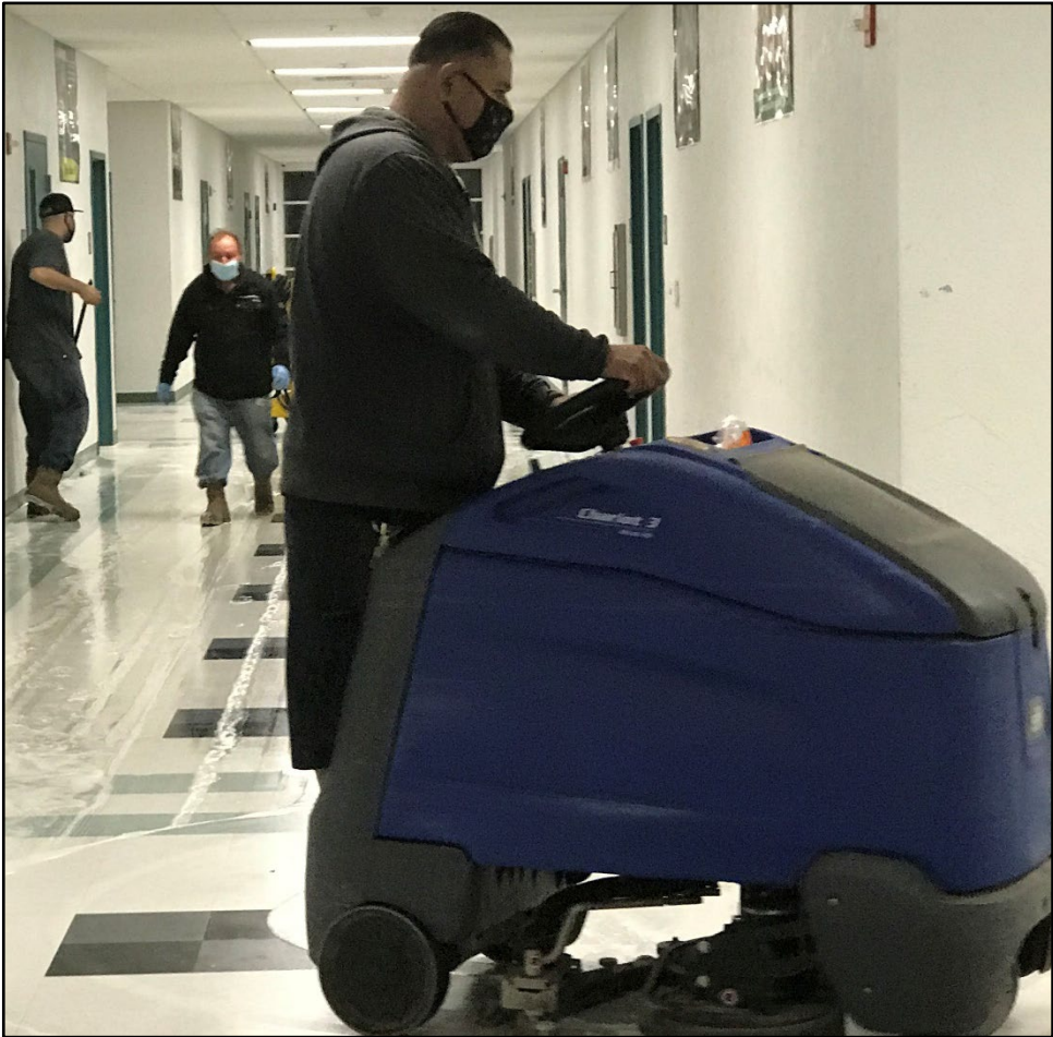
PVHS – Ruben Rodriguez Scrubs the Tile Floors Prior to Applying New Floor Finish
