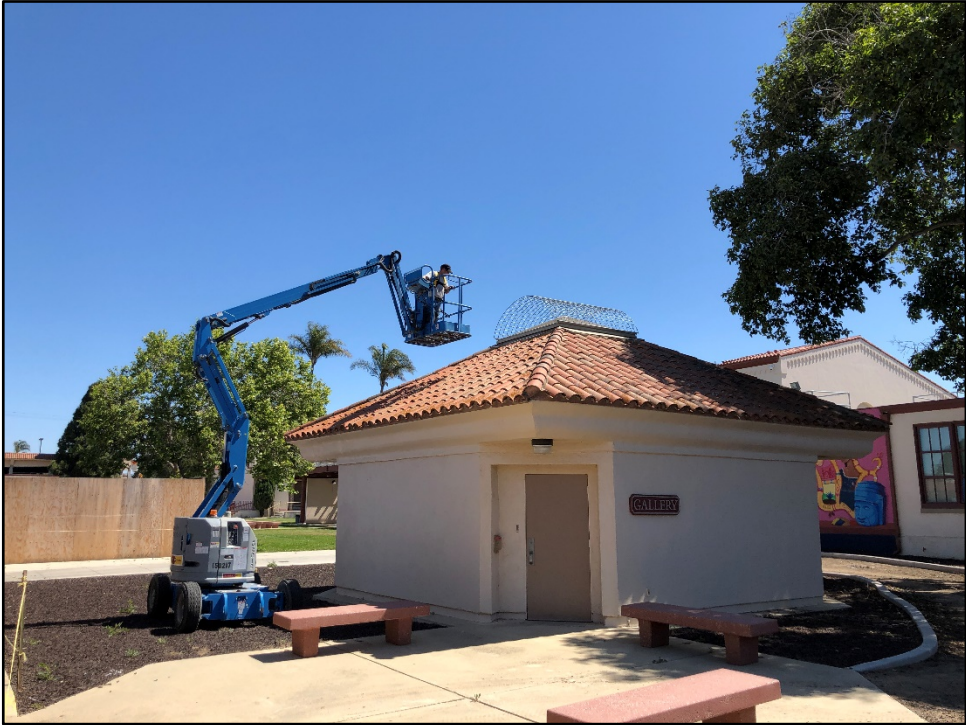
SMHS – Erik Fulton Completes the Skylight Protection at the Art Gallery
