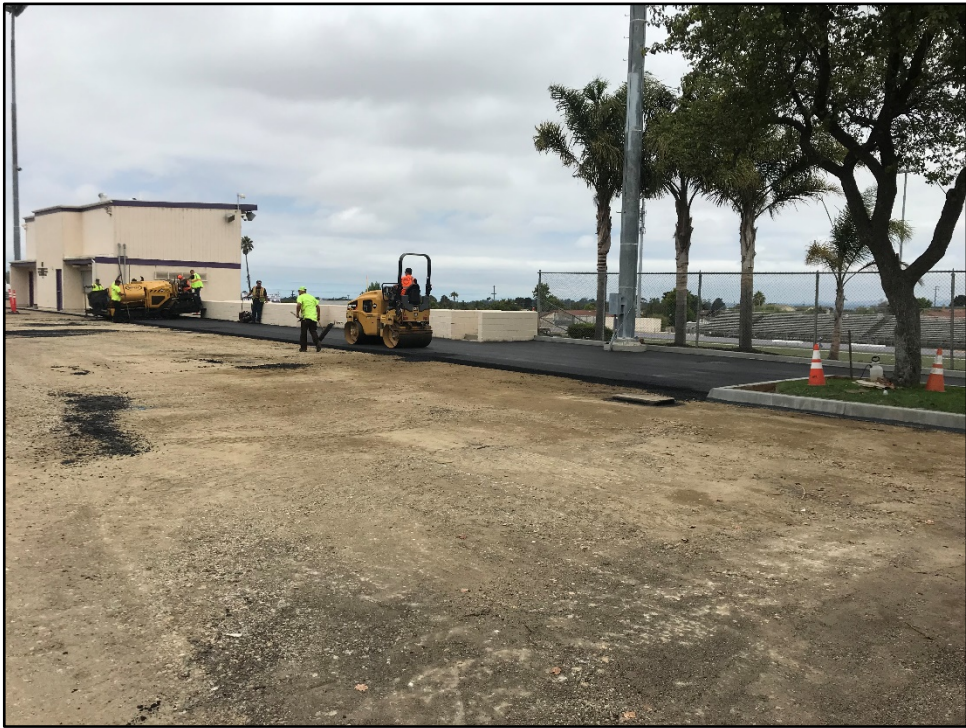
ERHS 2020 Paving – New Asphalt Goes Down at the Press Box and Physical Education Area
