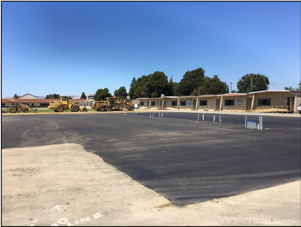
SMHS Eight Portable Classrooms – Paving is Complete and Awaits Classroom Buildings
