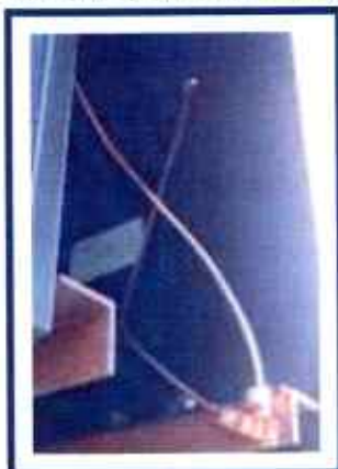
Support structure cannot be used as means of an earth ground
