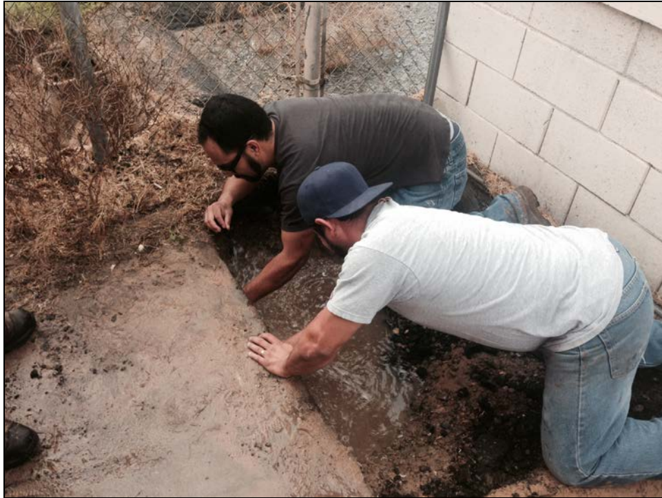
ERHS – Richardo Elisario & Flavio Rodriguez Repair a Water Leak at the Maintenance Shop
