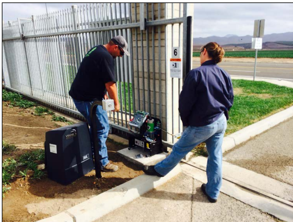
PVHS – New Gate Controls Installed & Programmed at Student Parking Lot
