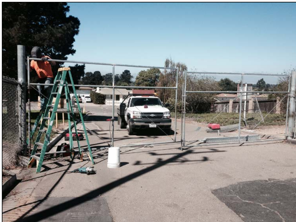
ERHS - New Gates and Fencing at the Berry Drive Entrance
