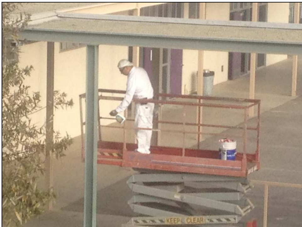
ERHS – Ernest Paz Prepares Walkway Columns for Paint
