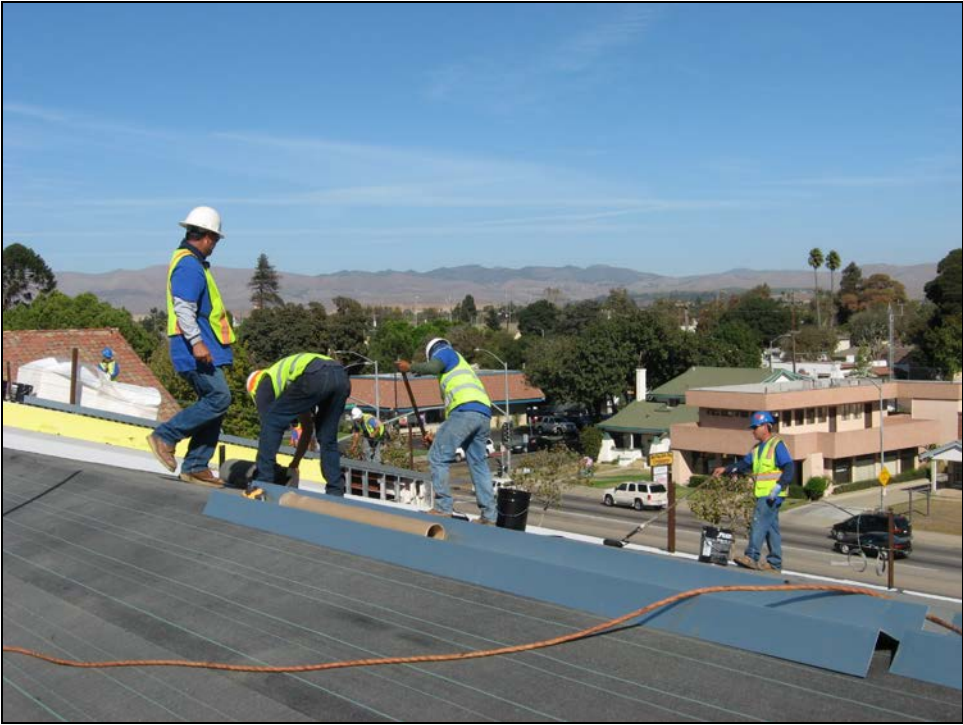
SMHS – 14 Classroom Building Roof Installation Underway
