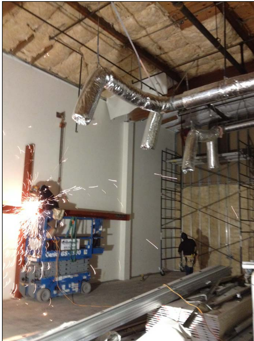
Support Services Center – Professional Development Center Steel Supports for Doors and Windows Set in Place & Welded
