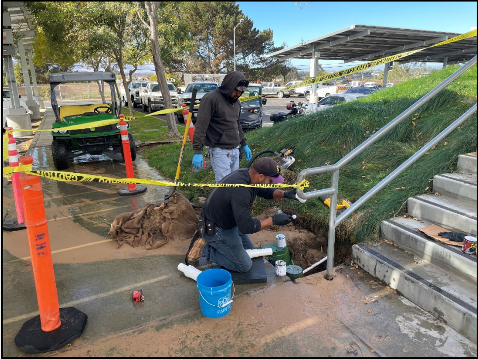
ERHS – Joseph Campos and Erick Escobar Repairing a Water Main Leak
