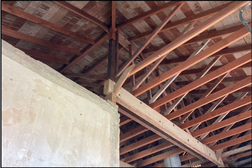
SMHS Admin to Classroom – Roofing Support Changes Are Being Made
