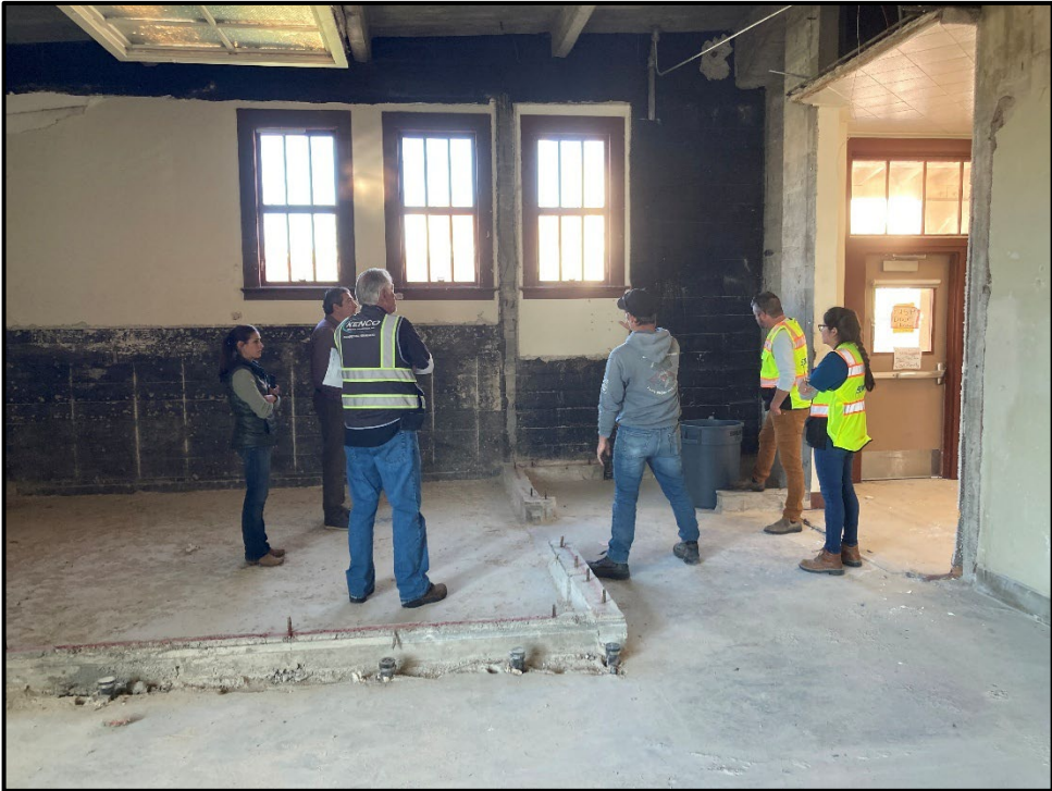
SMHS Admin to Classroom – Reviewing Demolition of Concrete Pillars
