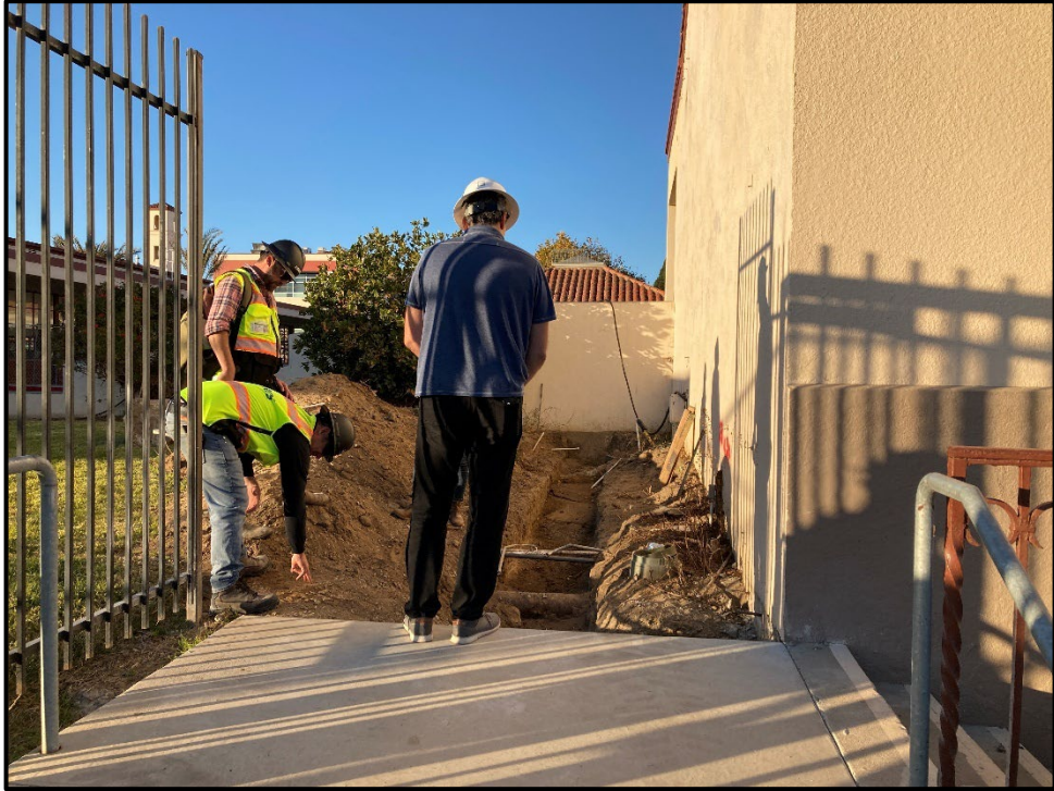
SMHS Admin to Classroom – Reviewing Existing Concrete Footings
