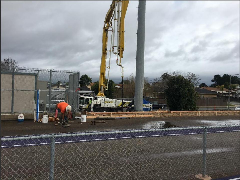
**ERHS – Concrete Pumper is Ready to Pour a Slab for Track & Field Storage**
