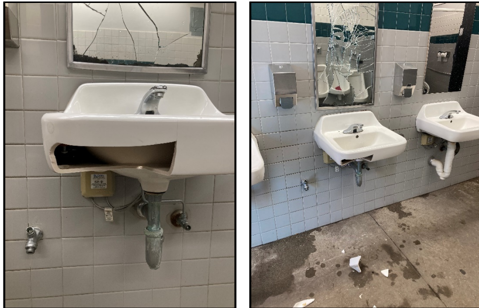
PVHS Restroom Damage – Sink and Mirror Broken
