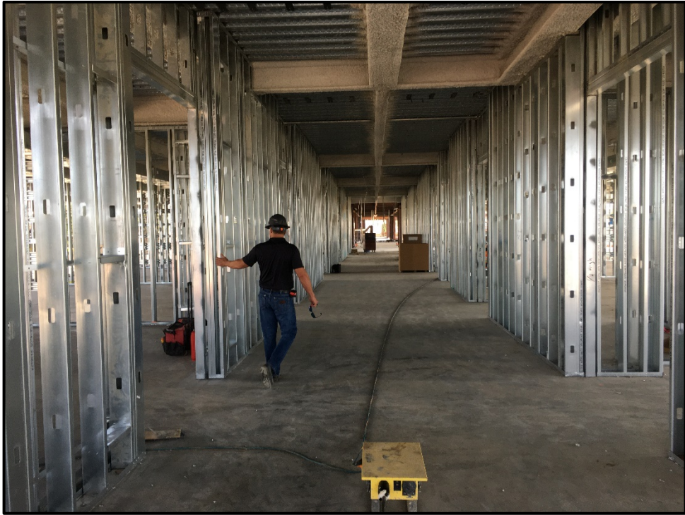
SMHS 50-Classroom Building – Inspector Reviews First Floor Hall Metal Studs
