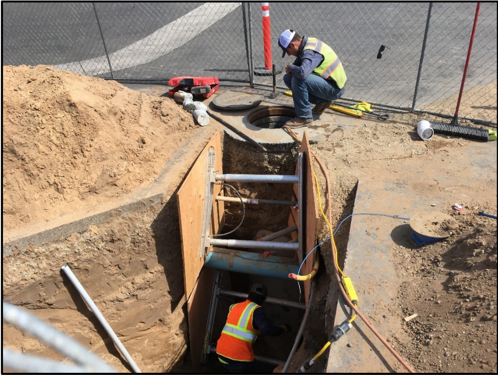
ERHS Maintenance and Operations Building – Sanitary Sewer Tie-in is In Progress
