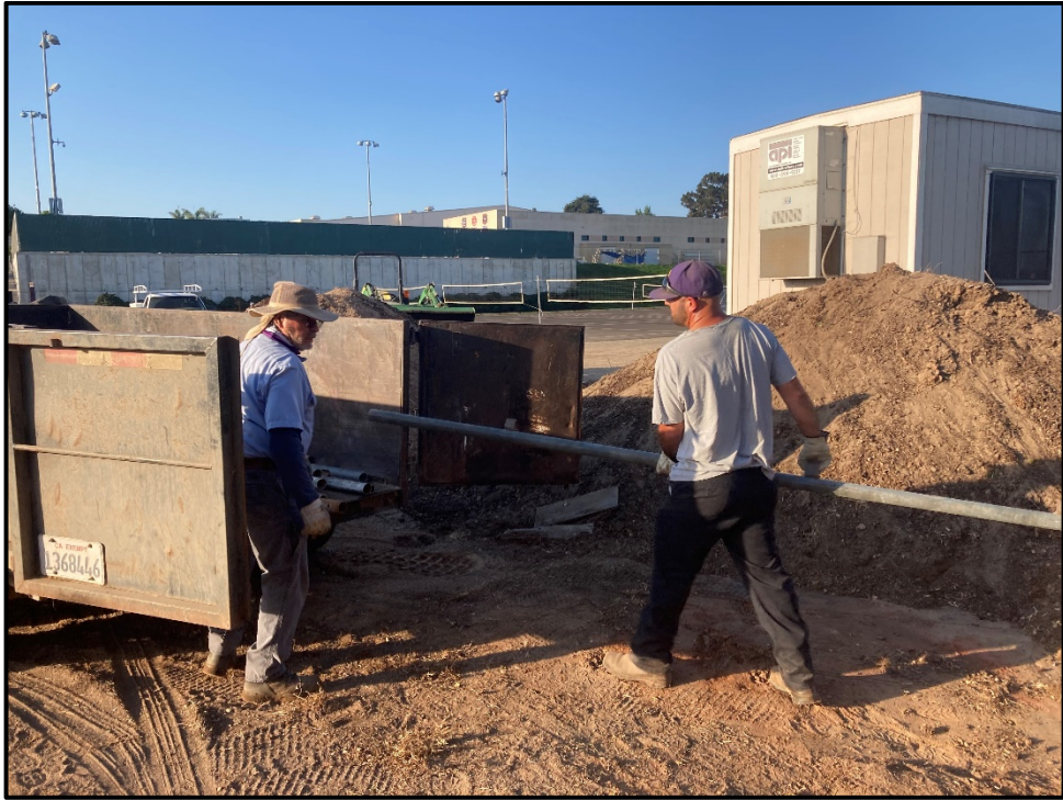
ERHS – Joseph Campos and Juan Rodriguez Remove Salvage Material to Prepare a Grounds Material Storage Area
