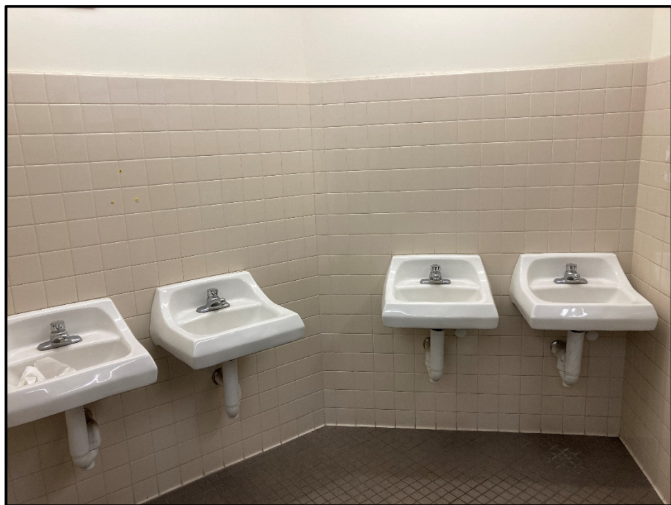
SMHS Restroom Damage – Soap Dispensers Completely Removed
