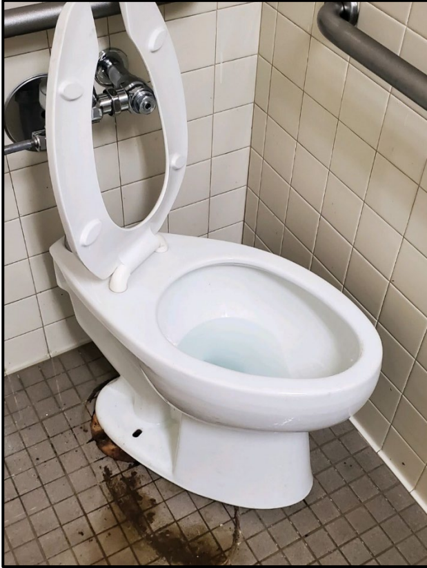
ERHS Restroom Damage – Toilet Knocked off its Base and Towel Dispenser Pried Open
