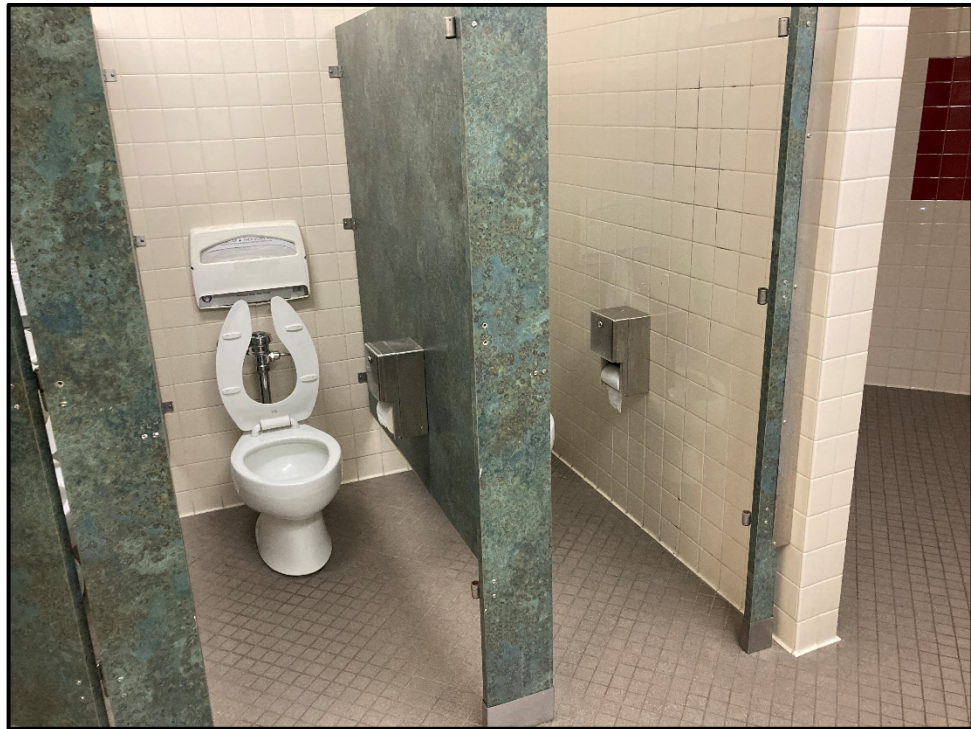
SMHS Restroom Damage – Partition Door Hinges Stolen
