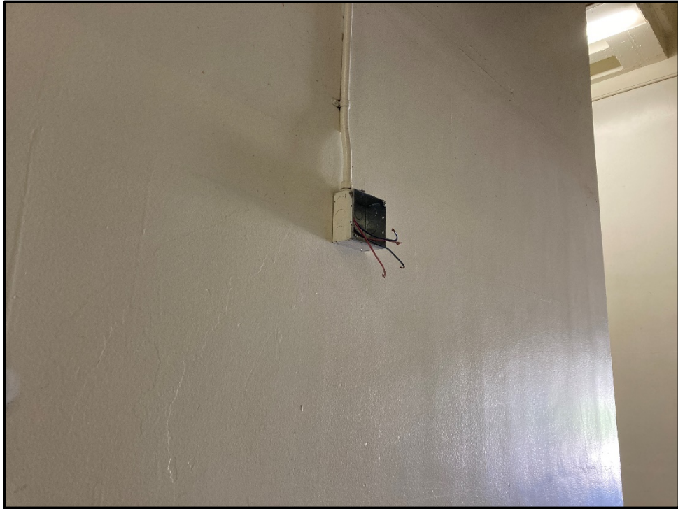
SMHS Restroom Damage – Fire Alarm Annunciator Removed from the Wall
