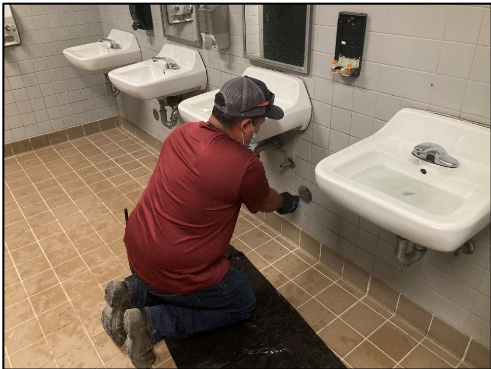
PVHS – Elias Camacho Clears a Plugged Drain
