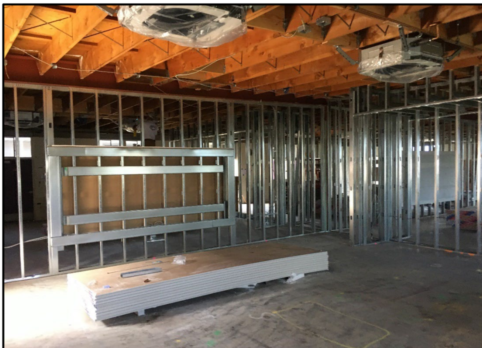
ERHS Modernization – New Metal Studs are in Place to Define Classrooms and Drywall Installations Begins
