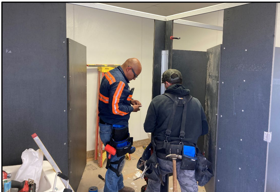
SMHS – Alex Banda and Tom Harold Re-install Restroom Partitions after New Flooring is Placed
