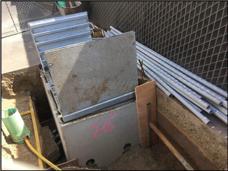
ERHS Maintenance and Operations Building – Underground Electrical Box is Installed
