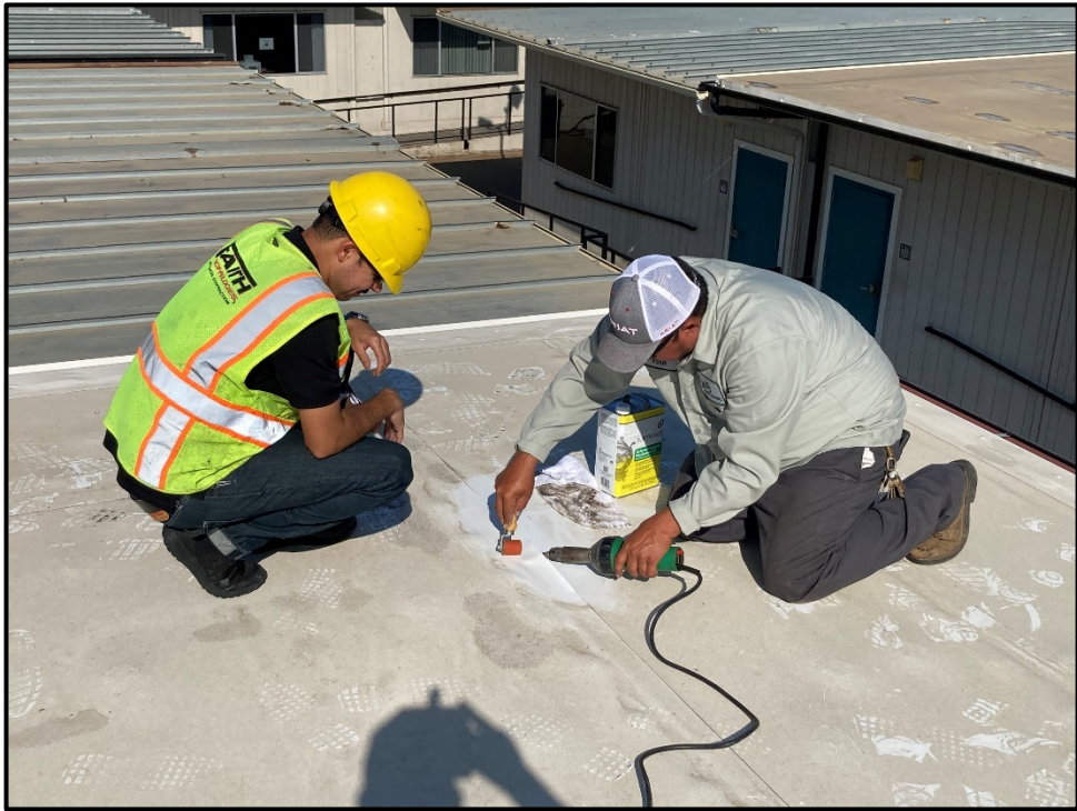
PVHS – Roofers Complete Repairs on the Replacement Roof at Classroom 620
