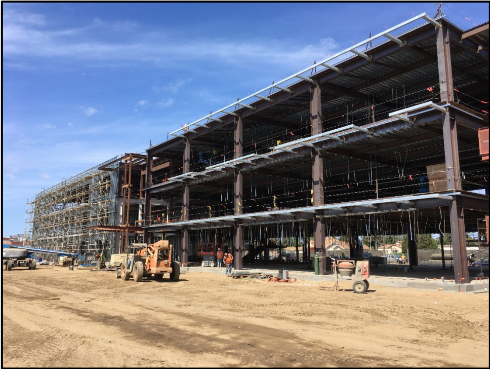
SMHS 50-Classroom Building – Campus View Shows the Exterior Structure Underway
