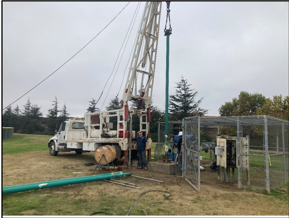
PVHS – Irrigation Well Piping is removed to Replace the Submersible Motor and Pump
