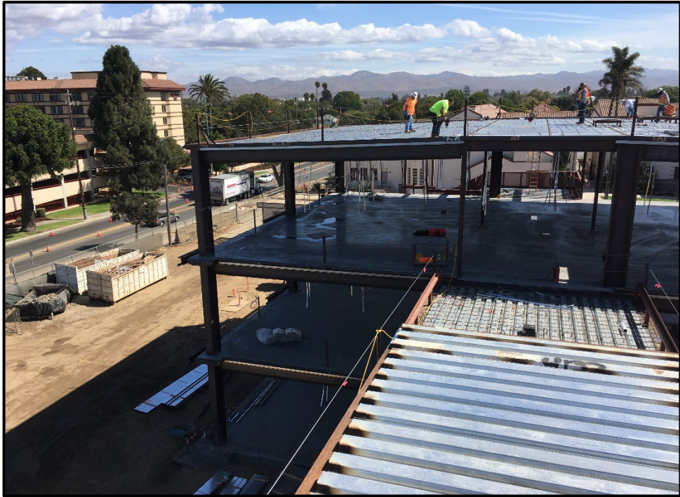
SMHS 50-Classroom Building – View from Roof Deck Shows Scale of the Building
