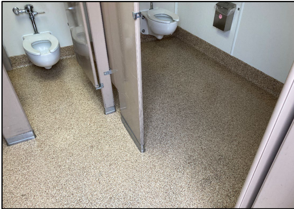
SMHS – New Flooring Installed in Two Portable Restroom Buildings
