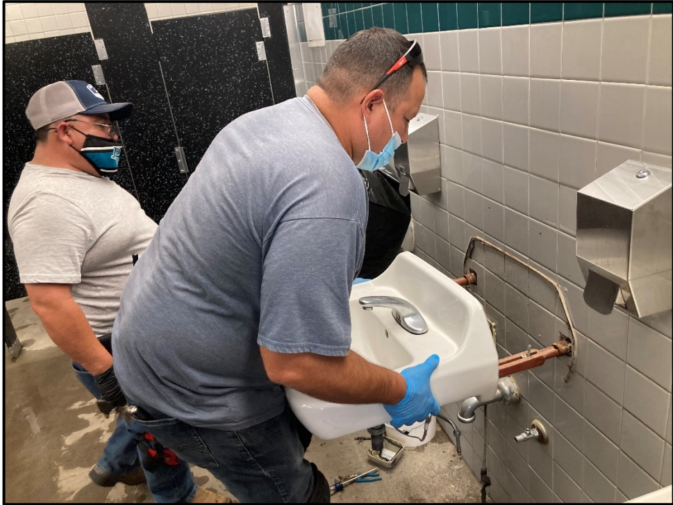
PVHS Restroom Damage – Elias Camacho and Jesus Reyes Re-install a Sink Pulled of the Wall
