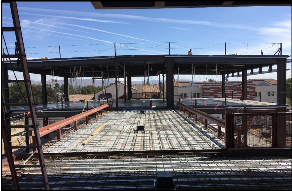
SMHS 50-Classroom Building – View of Walkway Decking Between Administration and Classrooms
