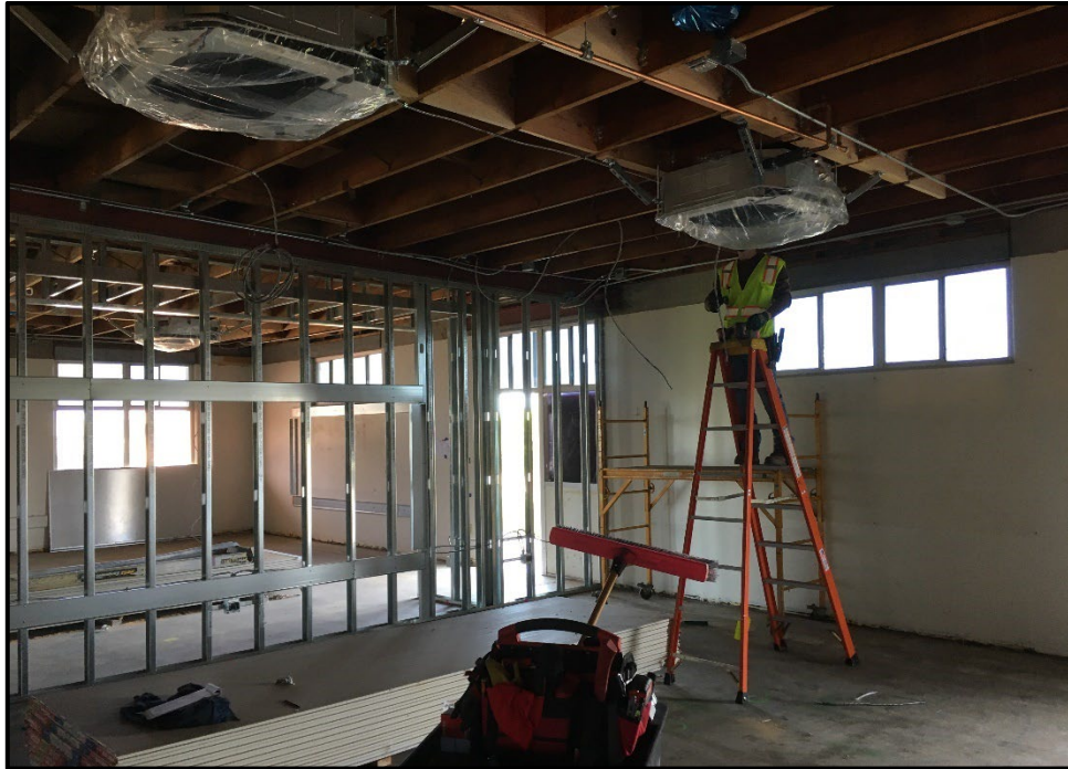
ERHS Modernization – HVAC Distribution Cassettes Installed and Plumbed to Variable Refrigerant Flow Compressors
