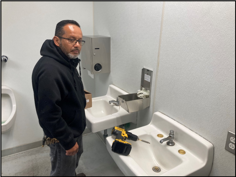
ERHS Restroom Damage – Jimmy Salutan Replaces Stainless Steel Soap Dispensers
