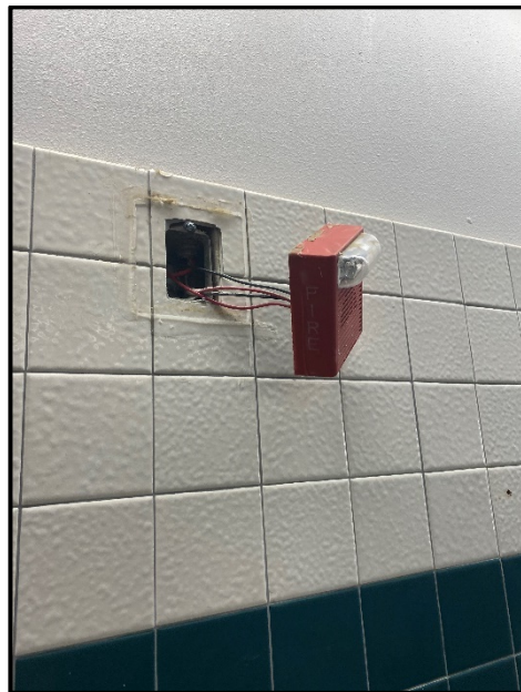
PVHS Restroom Damage – Fire Alarm Annunciator Ripped off the Wall
