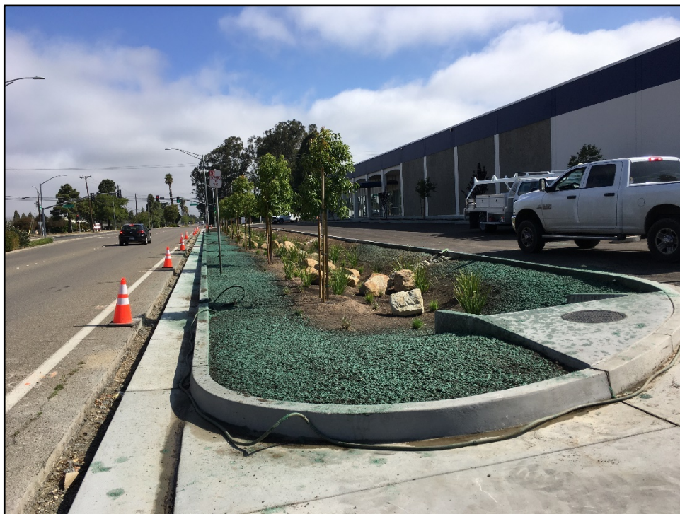
SSC West Parking - Landscaping In-Progress
