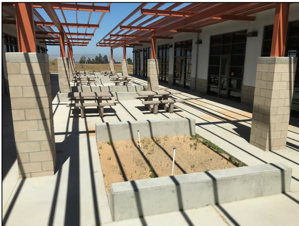
CTE Ag Center - Courtyard Between Shop Buildings is Finished
