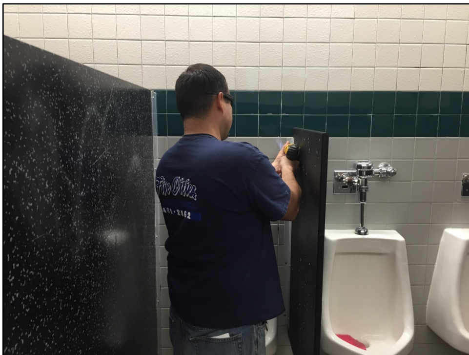
PVHS – Elias Camacho Repairs a Broken Partition in a Student Restroom
