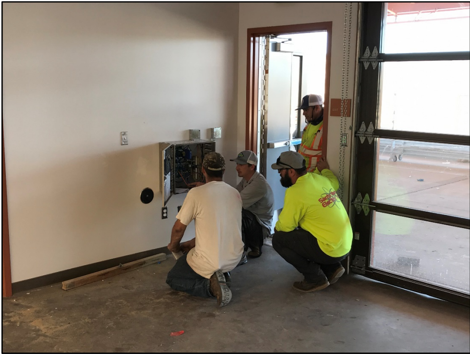
CTE Ag Center – Details on Air Handling Controls are Finalized
