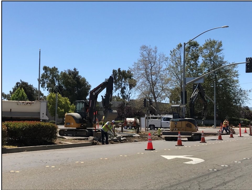
SSC West Parking - Existing Entrance Ties into the New Parking Lot
