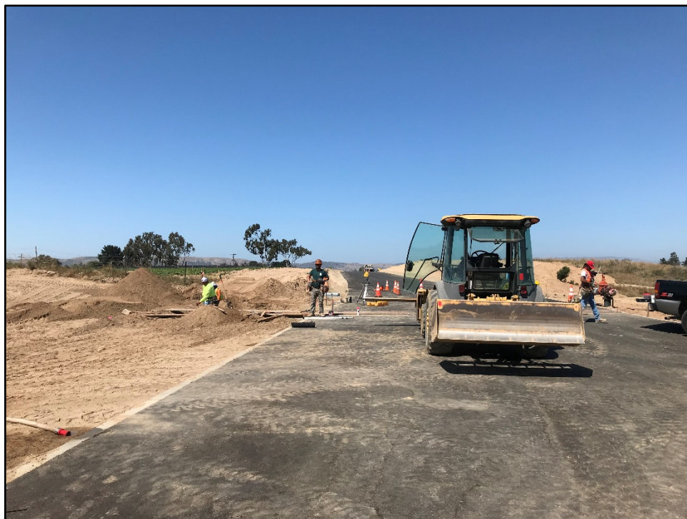
CTE Ag Center – Entrance Road with Rolling Gate Installation In-Progress
