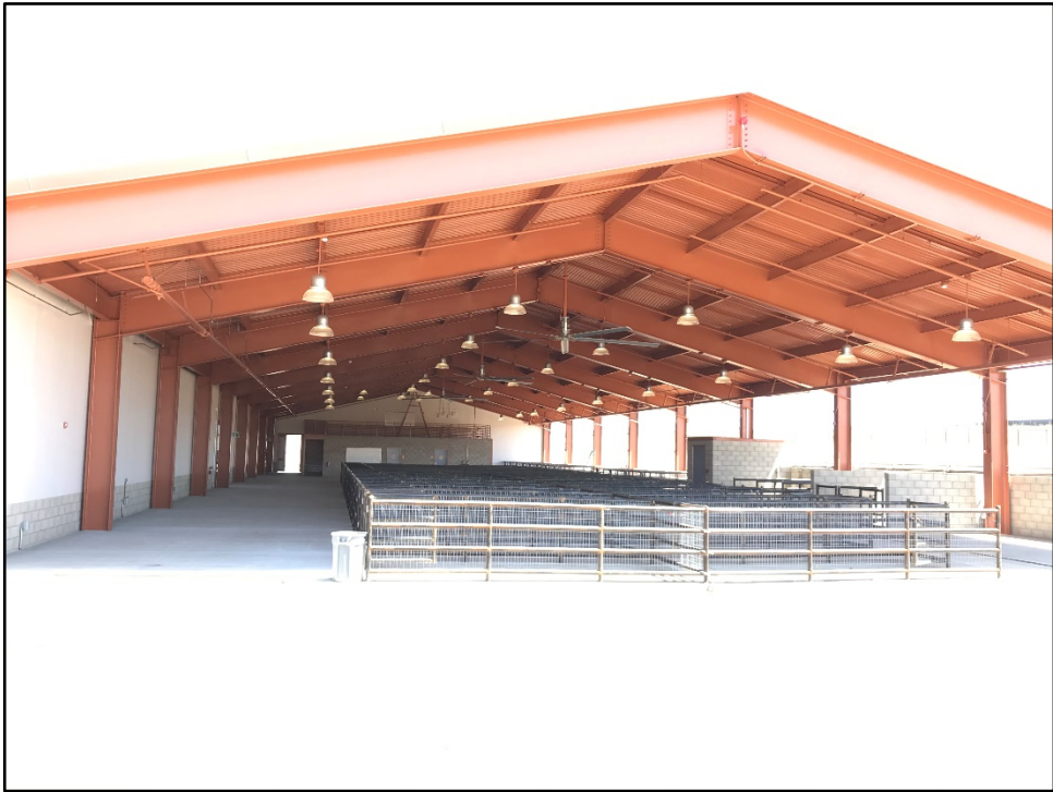
CTE Ag Center – Barn Painting, Lighting, and Animal Pen Installation Complete
