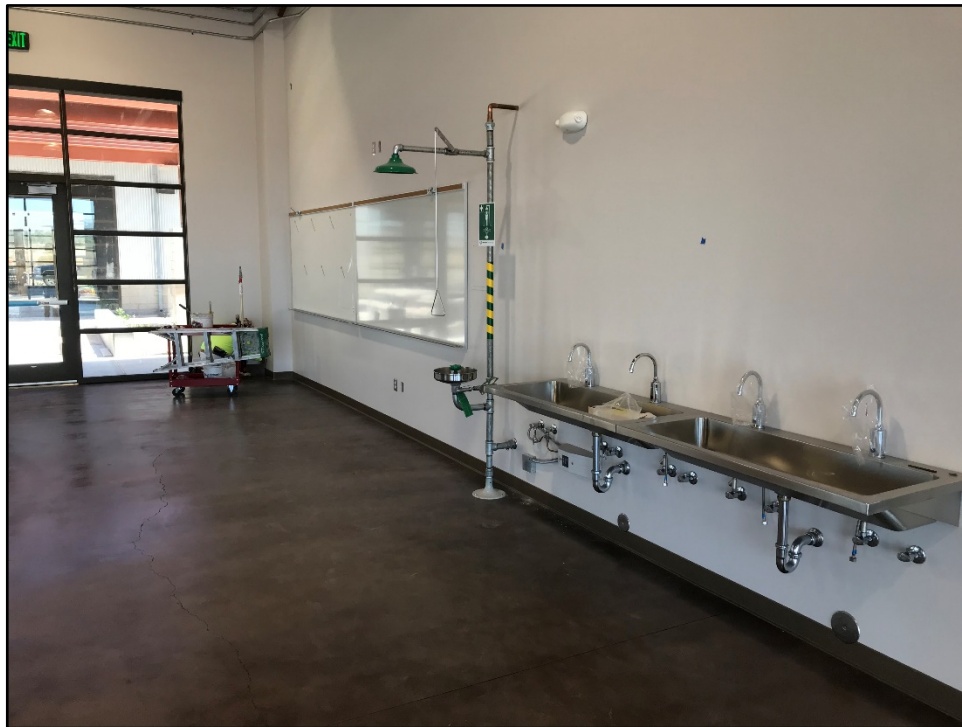
CTE Ag Center – Shop Spaces Include Sanitation and Emergency Equipment
