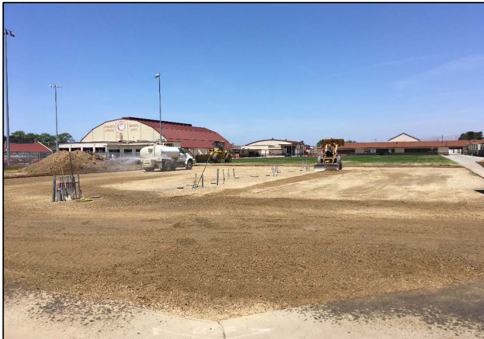
SMHS Eight Portable Classrooms – Underground Utilities Installed and Final Grading Begins
