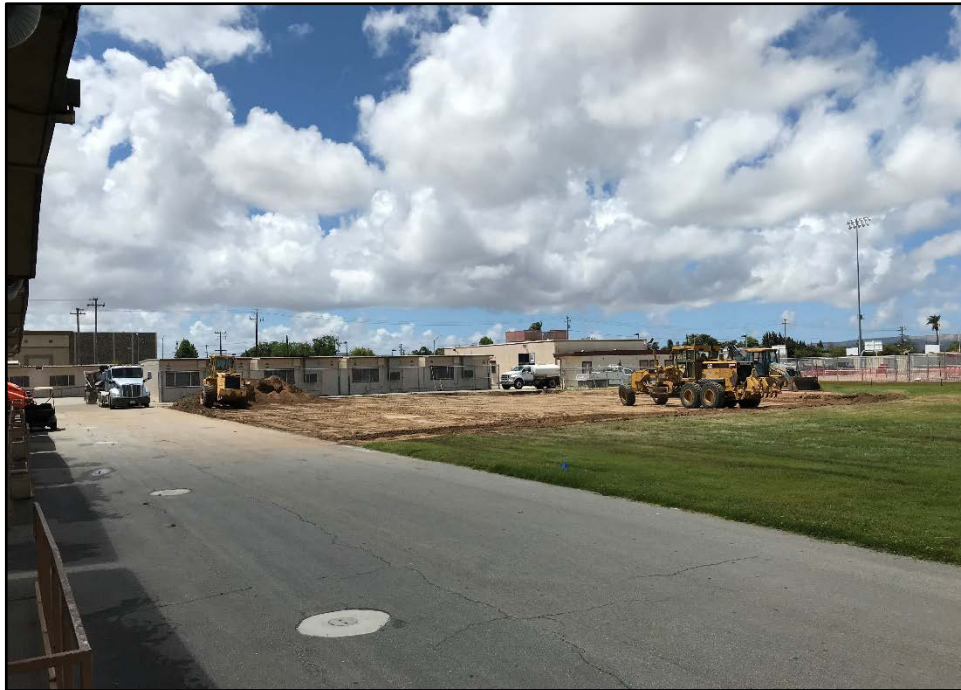
SMHS Eight Portable Classrooms – Removal of Softball Field and Earth Work Begin
