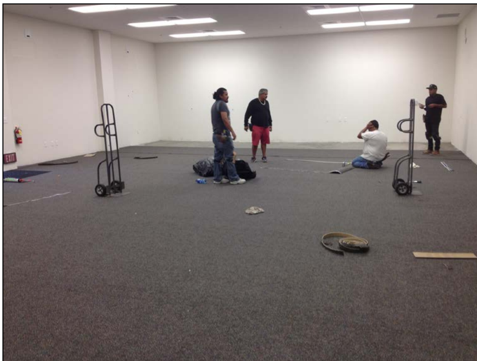
SSC – Professional Development Center Receives New Flooring
