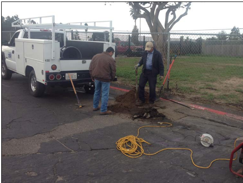
ERHS – Juan Rodriguez & Bernie Rayner Investigate a Water Leak in the Staff Parking Lot
