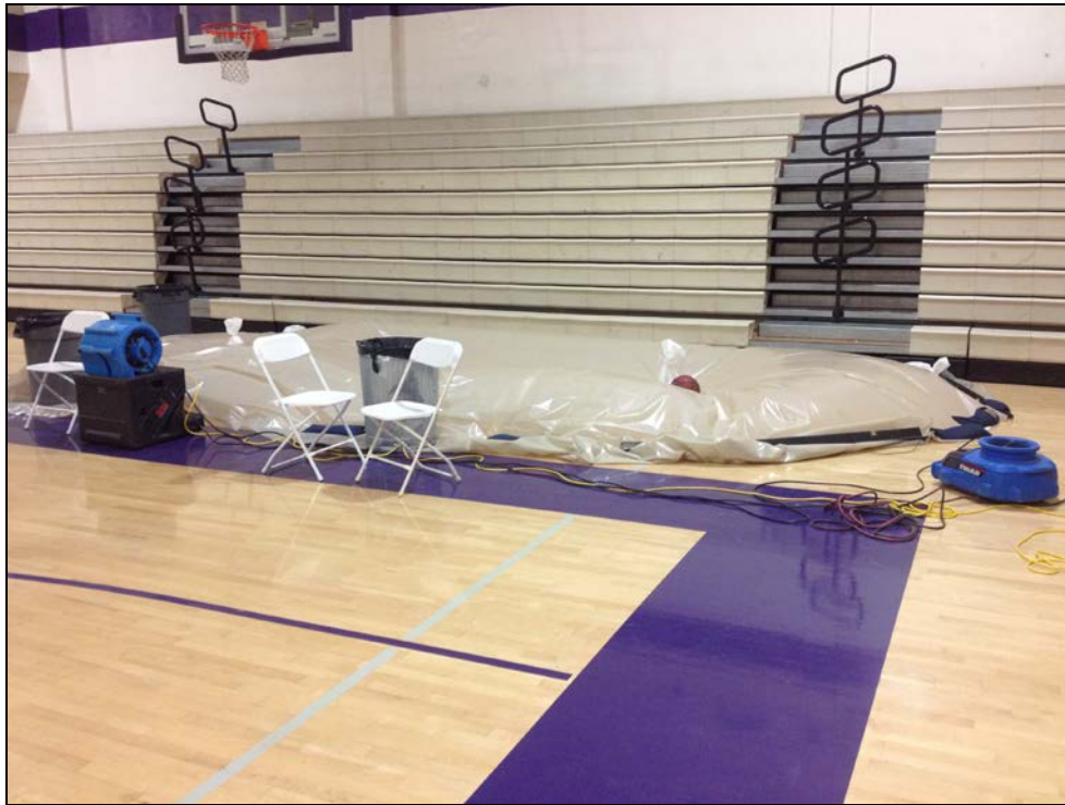
ERHS - Heat and Lots of Air Remove Moistures from the Gymnasium Floor
