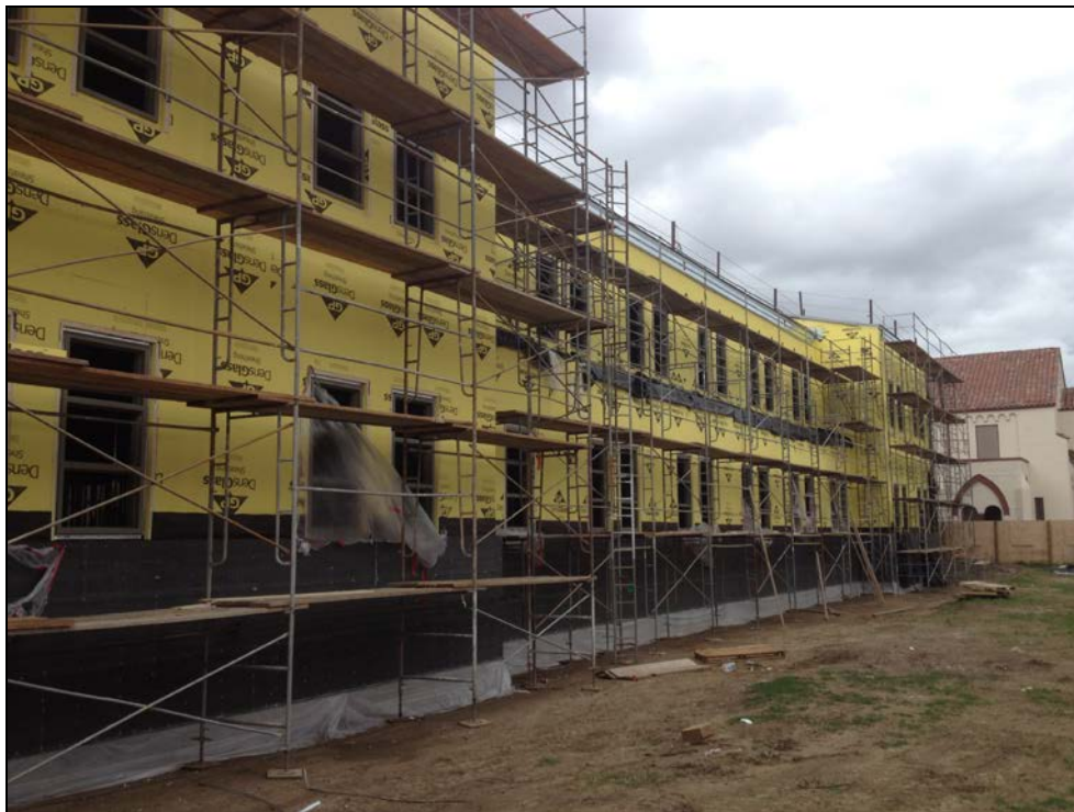
SMHS – 14 Classroom Window Frames and Stucco Paper Installation in Progress
