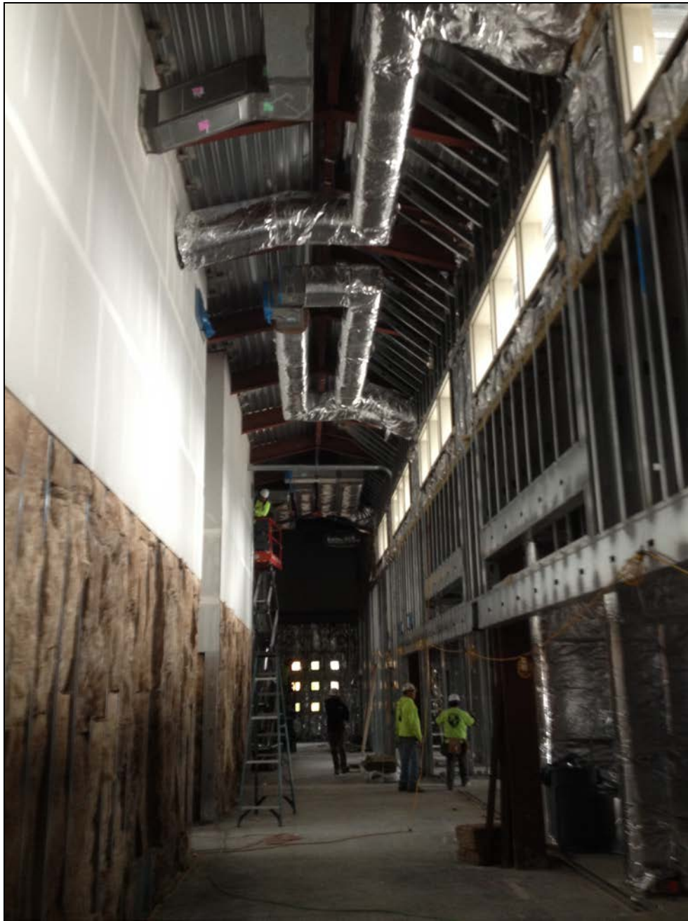
SMHS - Second Story Drywall Installation in the 14 Classroom Hallway
