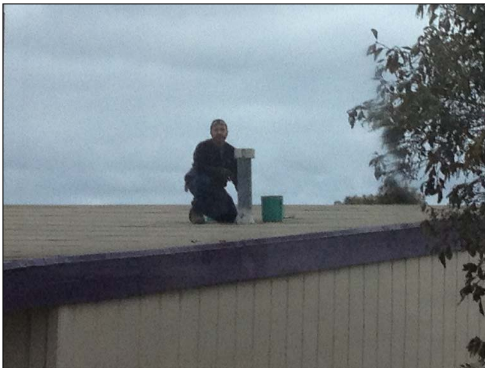
ERHS - Bernie Rayner Addresses a Water Leak on the Weight Room Roof
