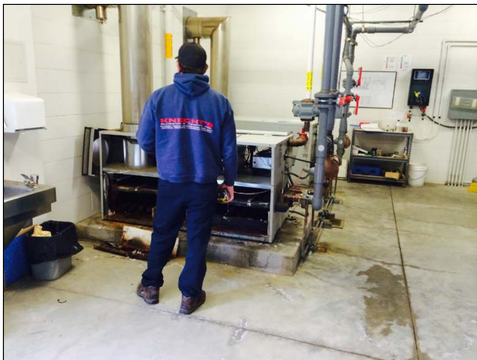
PVHS – Service Technician Inspects Leaking Pool Heaters
