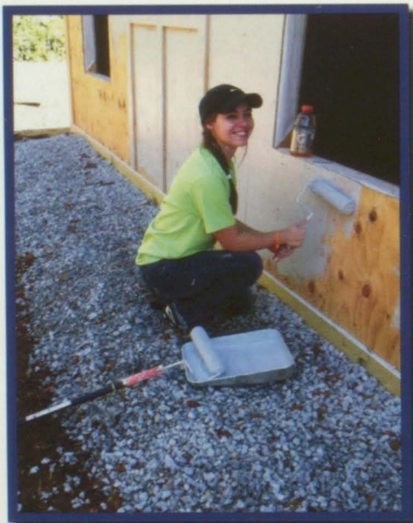
Senior Abby Rainwater works diligently to finish painting the house.
