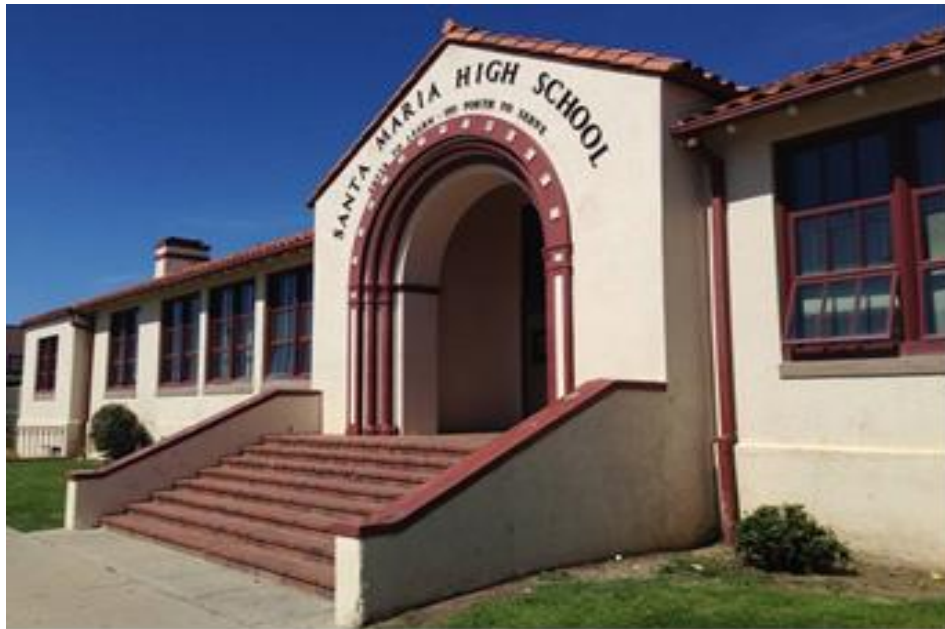
Santa Maria High Camino Colegio main entrance
