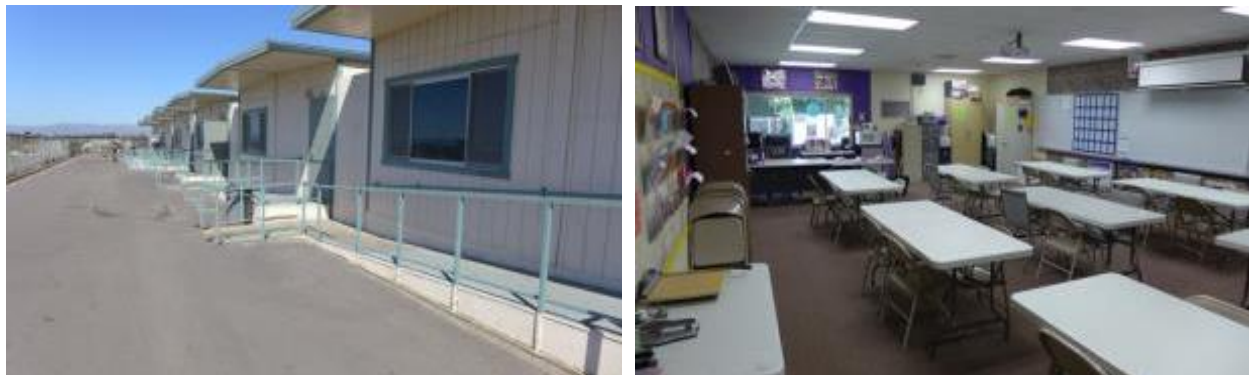
Exterior and interior views of typical existing portables.
