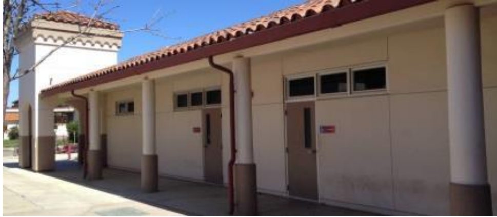
Exterior condition of Classrooms 230-235
