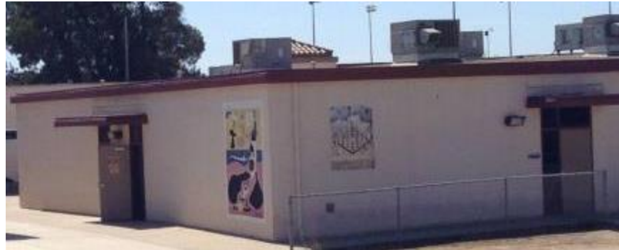
Exterior condition of Classrooms 240-247
