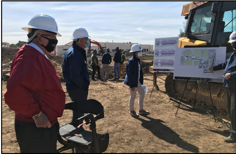
SMHS 50-Classroom Building – School Board Members Review the Construction Plan
