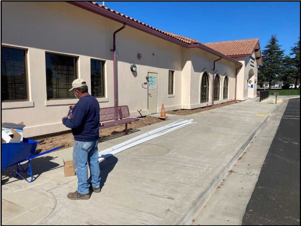
DHS – Lorenzo Mendez Assembles New Sprinkler Lines for the Entry Planter
