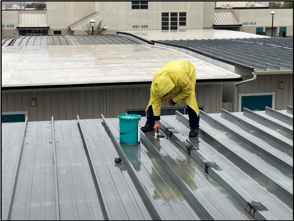
PVHS – Elias Camacho Patches a Portable Classroom Roof
