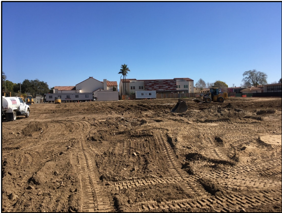
SMHS 50-Classroom Building – Clear View from Industrial Arts to Ethel Pope Auditorium
