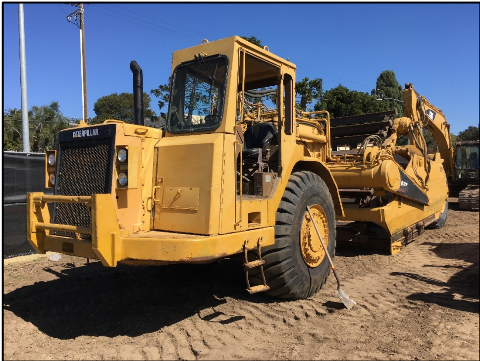
SMHS 50-Classroom Building – Equipment of All Sizes Required on this Project
