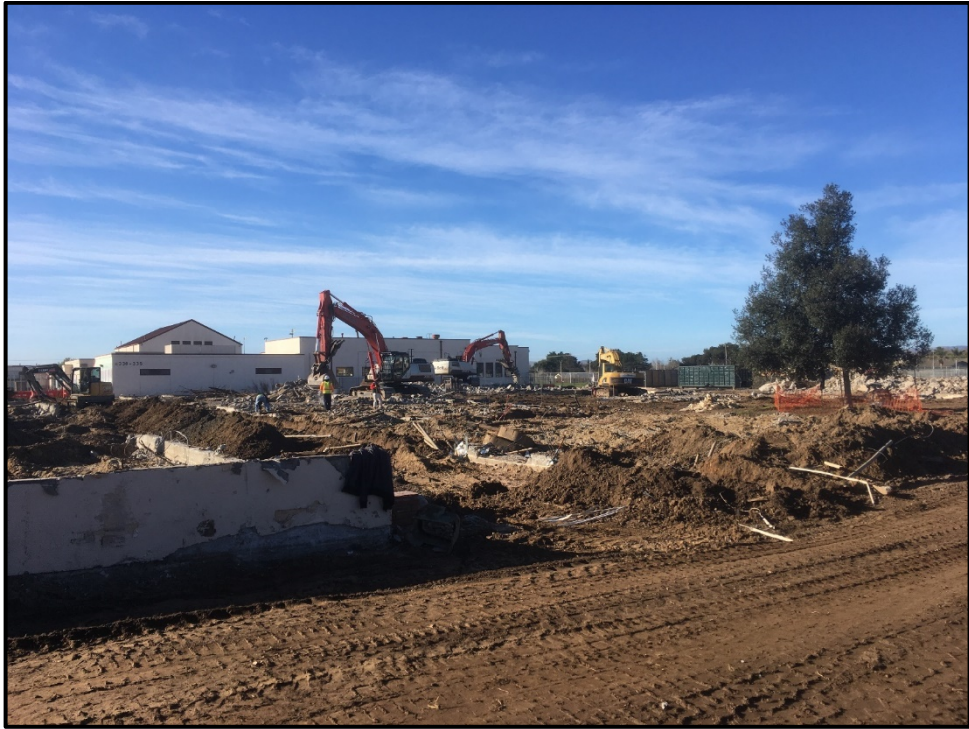
SMHS 50-Classroom Building – Demolition Nears Completion
