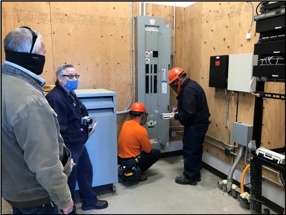
PVHS – Del Ward Assists with an Electrical Arc-Flash Assessment
