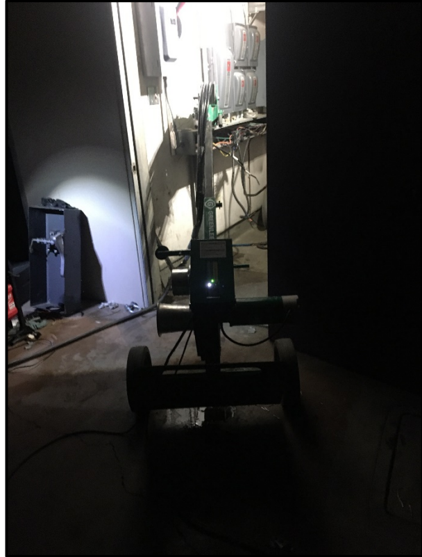
ERHS – Replacing Failed Electrical Feeders Over a Holiday Weekend
